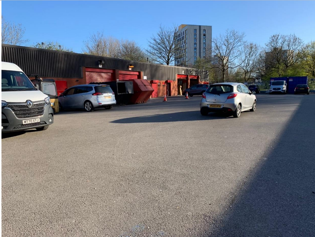
PLATE 1 LOOKING NORTH ON THE SITE
