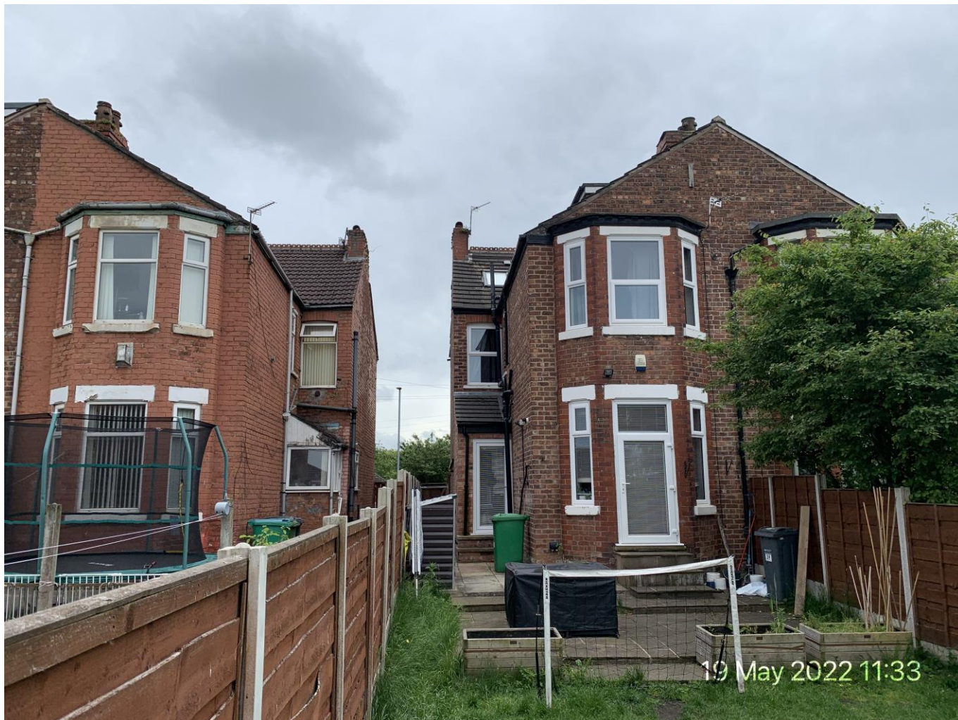
Photograph 2: Rear elevation and existing conservatory. Source: Site Photographs
