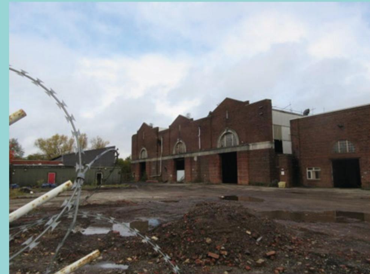
Image 7: Later, likely late 1930s' structures east of the canal in 2020. The simpler style may reflect architectural fashion rather than finances.
