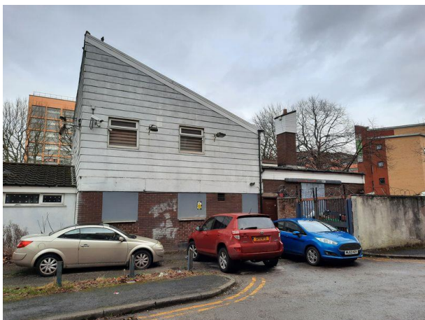
Plate 9.3: Building and Rendered Wall (Right).
