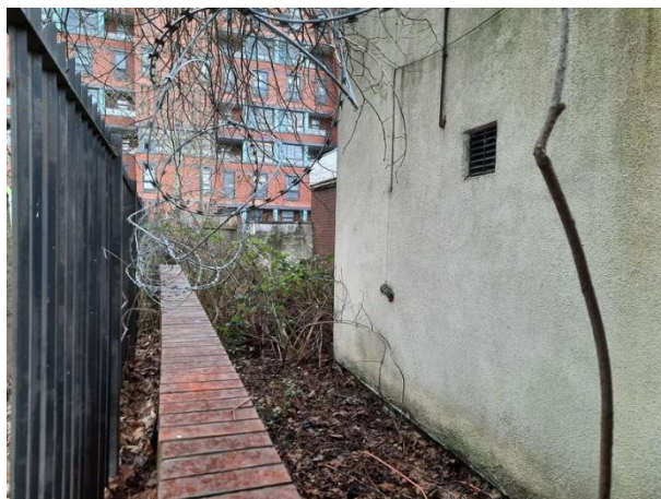
Plate 9.2: Bare Ground, Building (Right), Wall and Fence (Left).
