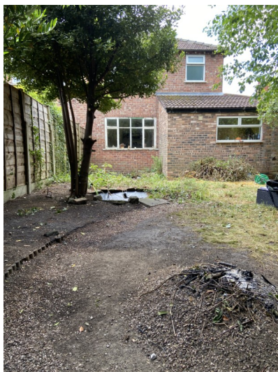
North facing rear elevation of 17 Lynton Drive
