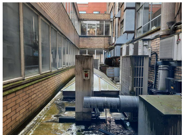
Plate 9.6: The Southern Hardstanding Courtyard, at the First Floor Level of Building 2.
