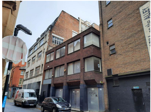
Plate 9.2: West Side of 5 Ridgefield (Building 2) in relation to Old Colony (Left) and Grange House (Right).
