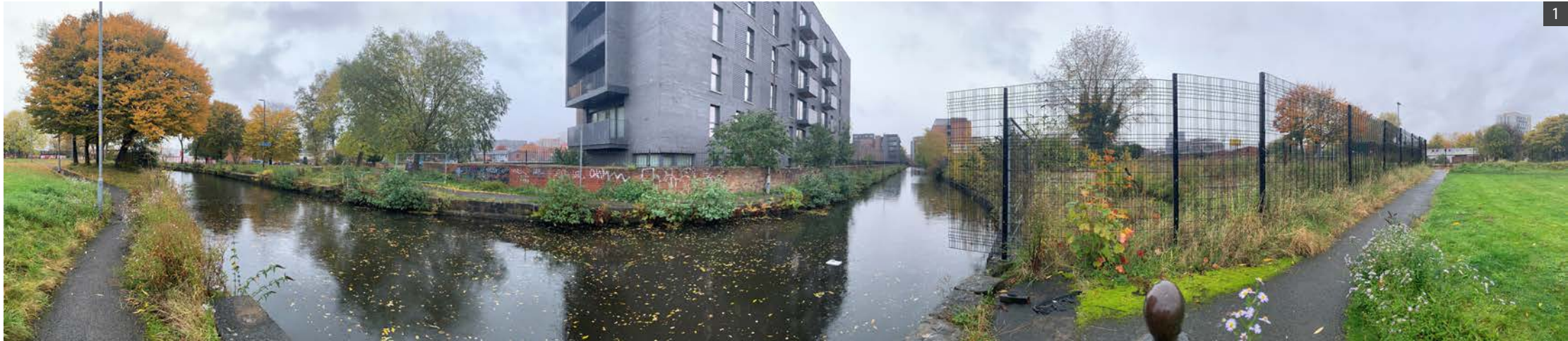
East and west view along Rochdale Canal
