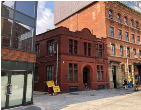
Cutting Room Square
