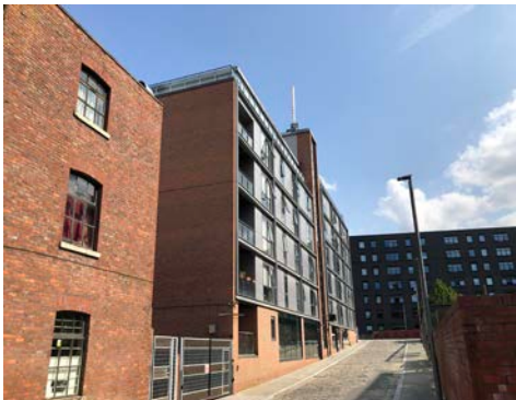
Flint Glass Wharf
