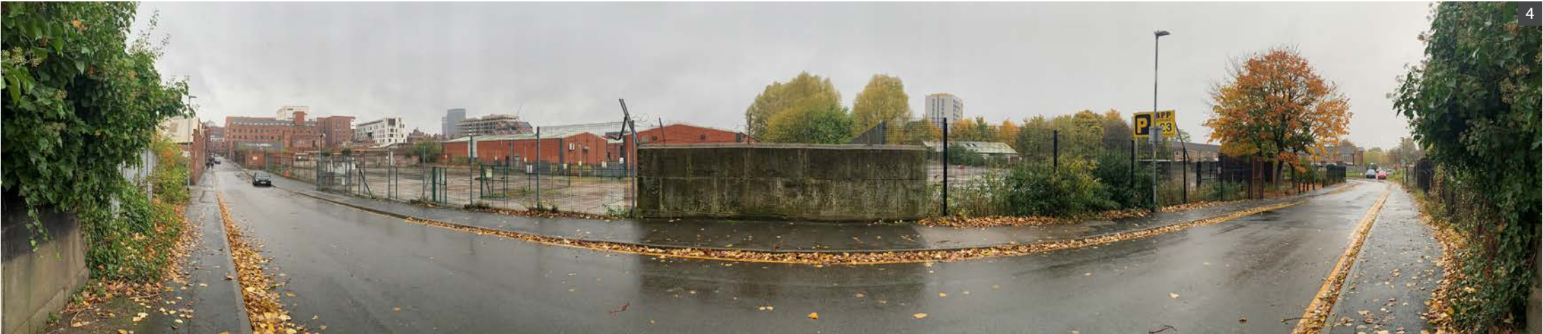
Canal arm bridge wall looking north
