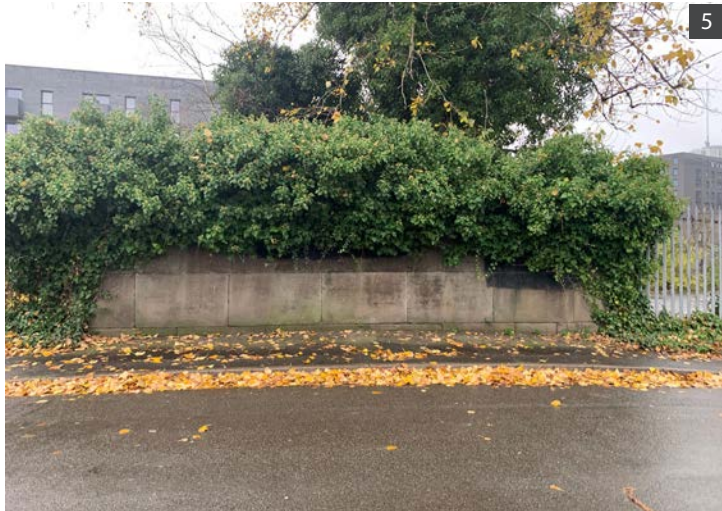
Canal arm bridge wall looking south
