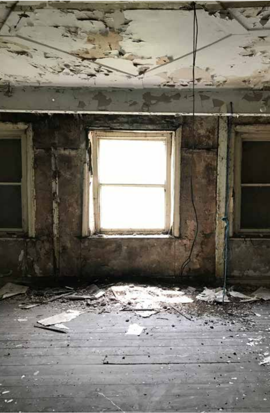
photograph of townhouse at second floor
