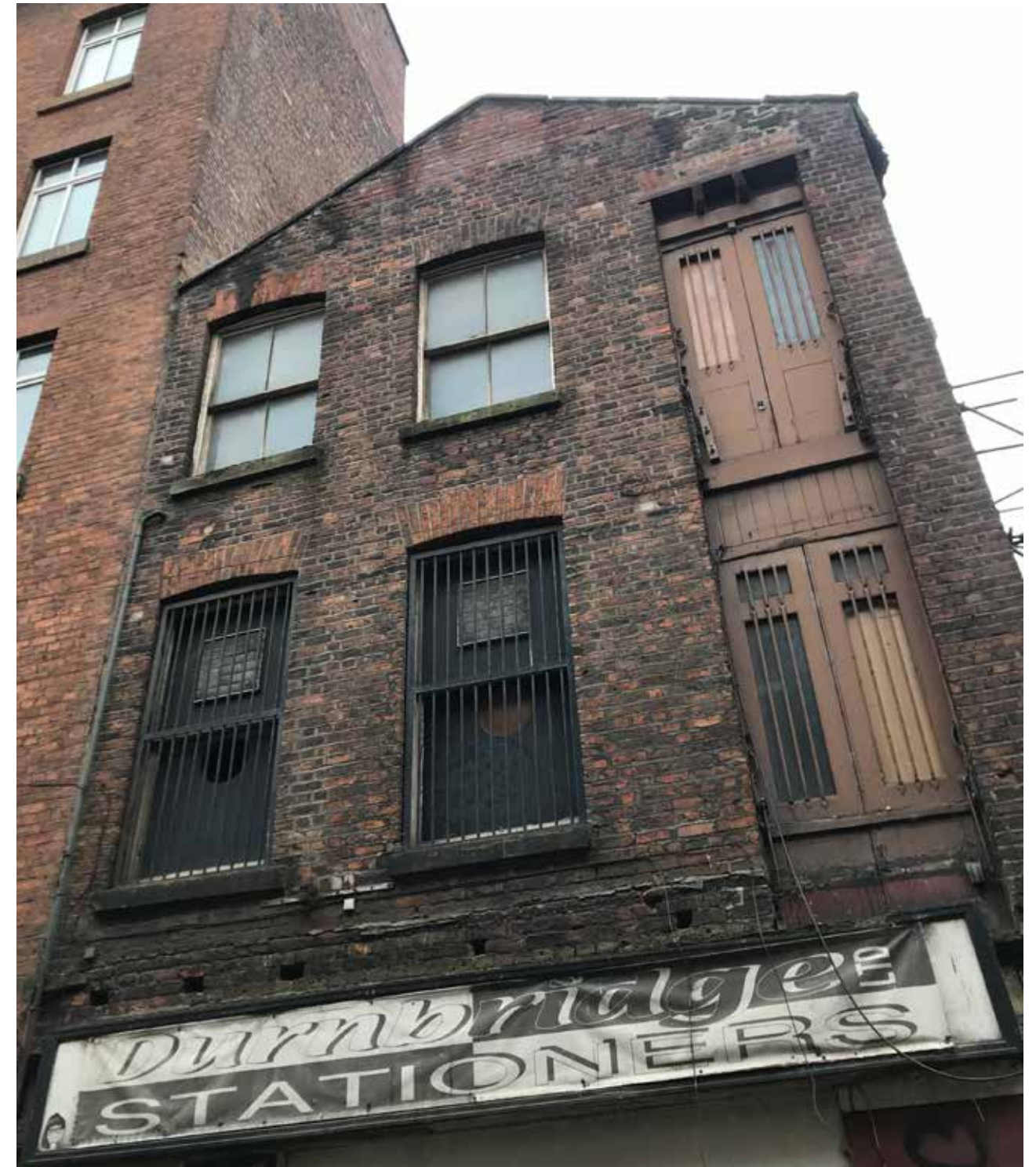
photograph of warehouse from Back Piccadilly
