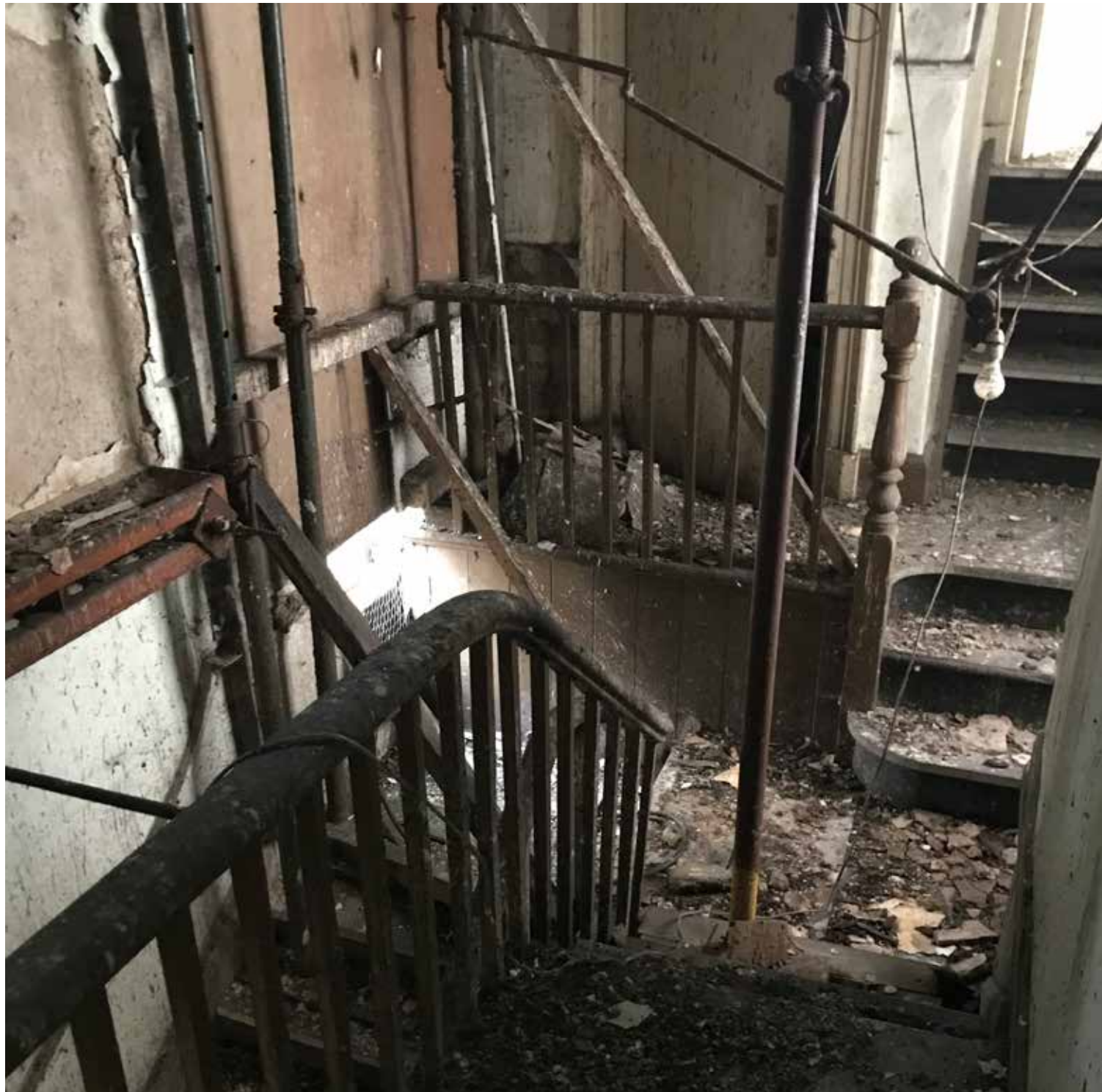
photograph of townhouse staircase at first and second floor
