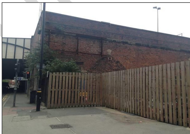
Figure 2: Photo of the easternmost part of the listed viaduct, looking east from Great Bridgewater Street. The Great Bridgewater Street bridge is glimpsed into view to the left.
