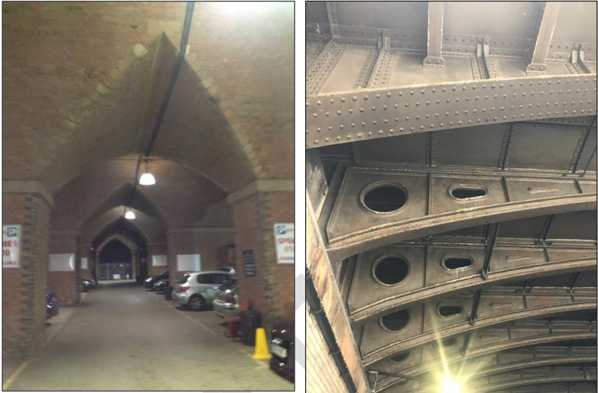
Figure 3 (left): Photo of the interior of the listed viaduct c.2019, comprising original vaulted brick undercroft complete with stone quoins and stringcourse. Figure 4 (right): Photo of the cast iron girders to the Great Bridgewater Street Bridge.
