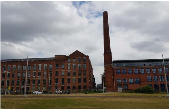
Chimney On Pollard Street
