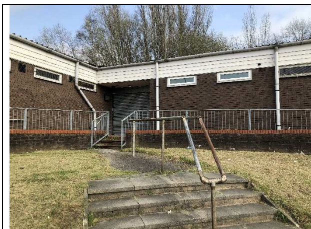
Photo 7: Entrance to building - south east side
