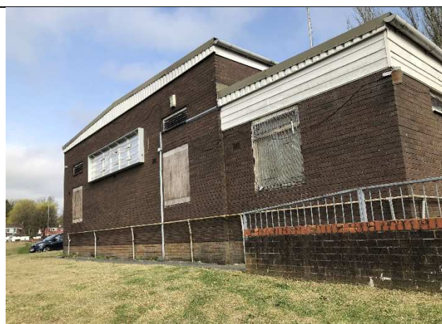
Photo 5: Building – southern side.
