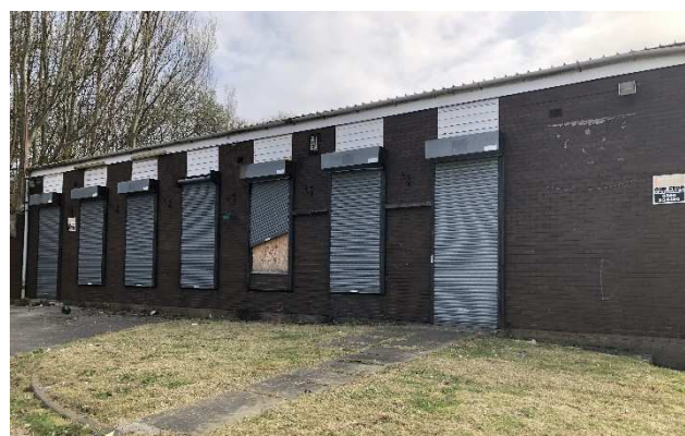
Photo 6: Building- western side.
