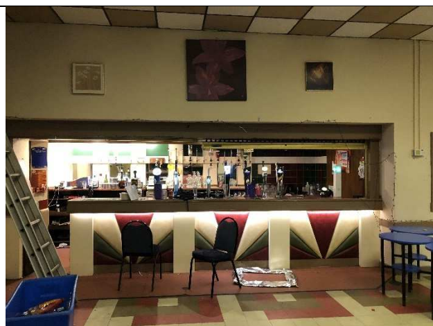
Photo 15: Bar area west side of building.
