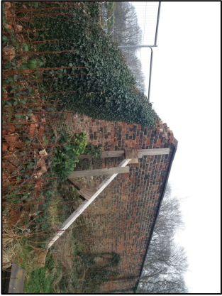
P8. View of collapsed section of boundary wall to South Elevation
