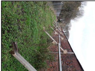
P3. View along wall to West Elevation showing raking shores.
