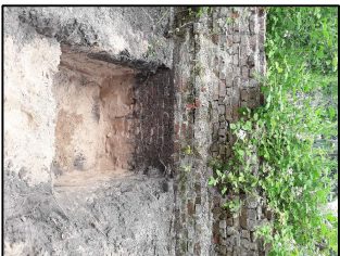
P11. View of trial hole dug at the base of the South Elevation boundary wall.
