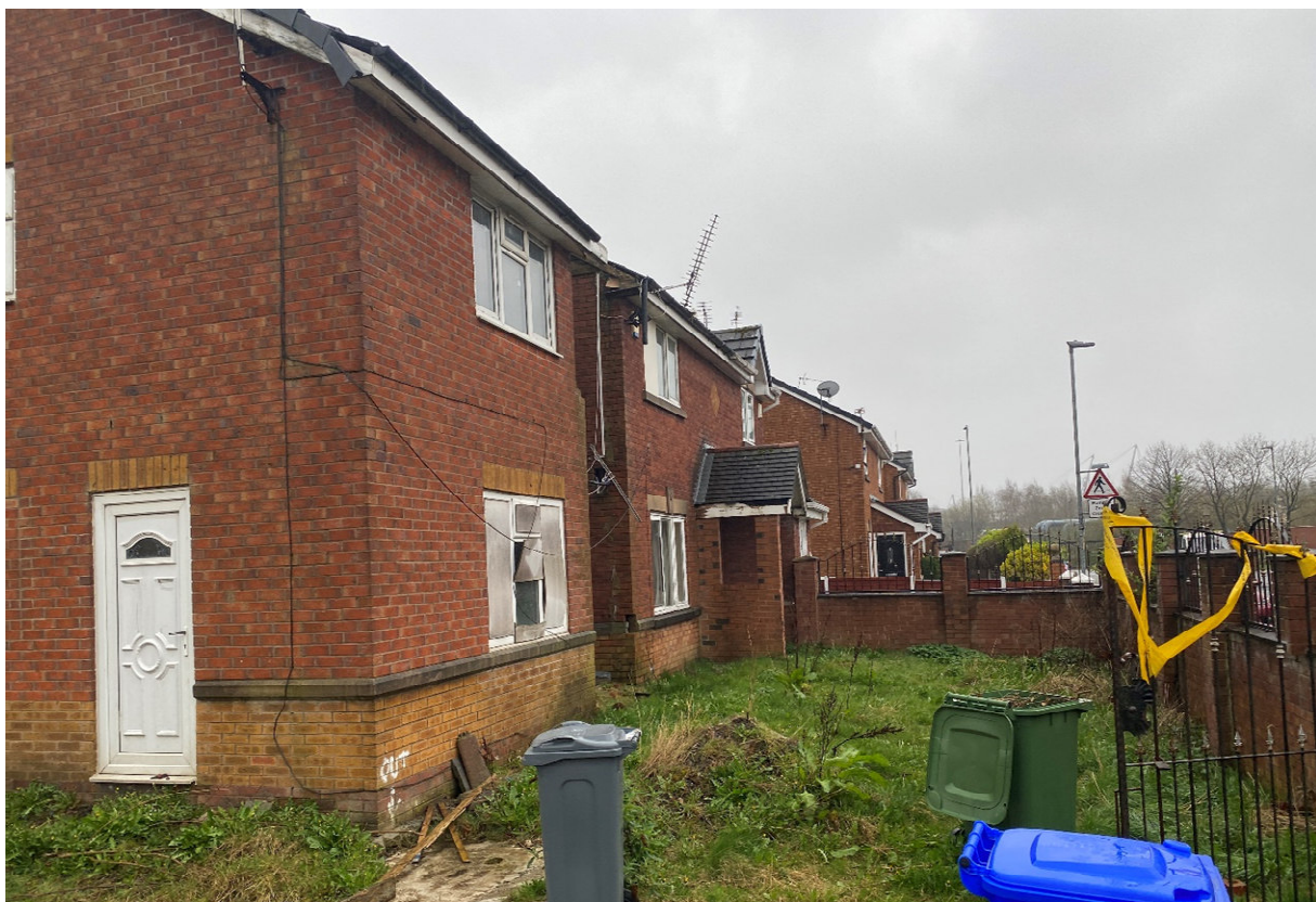
Photograph 2 – Western extent off Saxon Street
