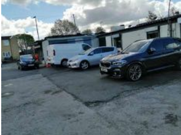
P3: North-east portion of the site, looking south-east
