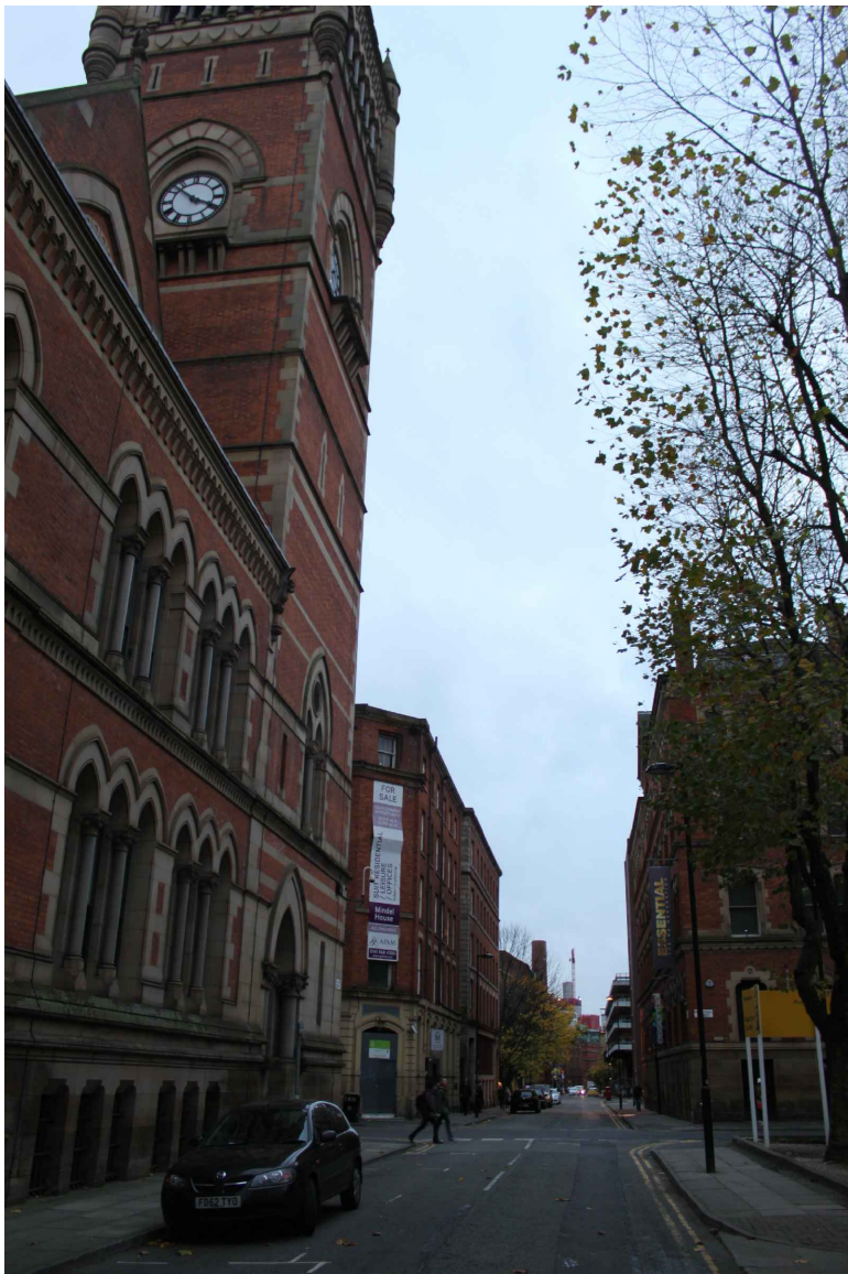
Existing Street View 4
