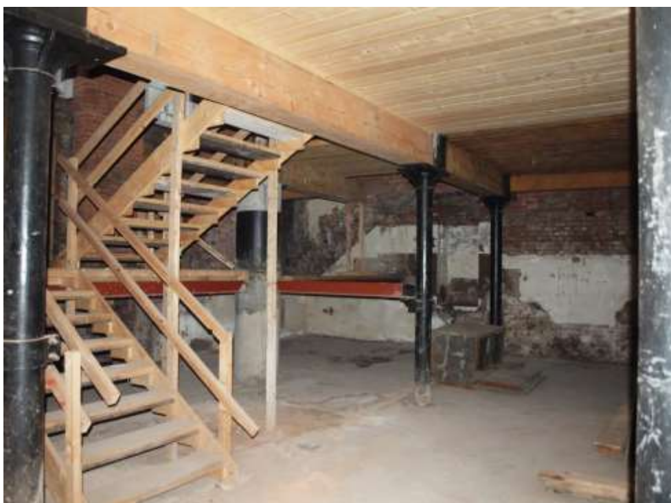
Plate 30: Detail of inserted staircase to ground floor
