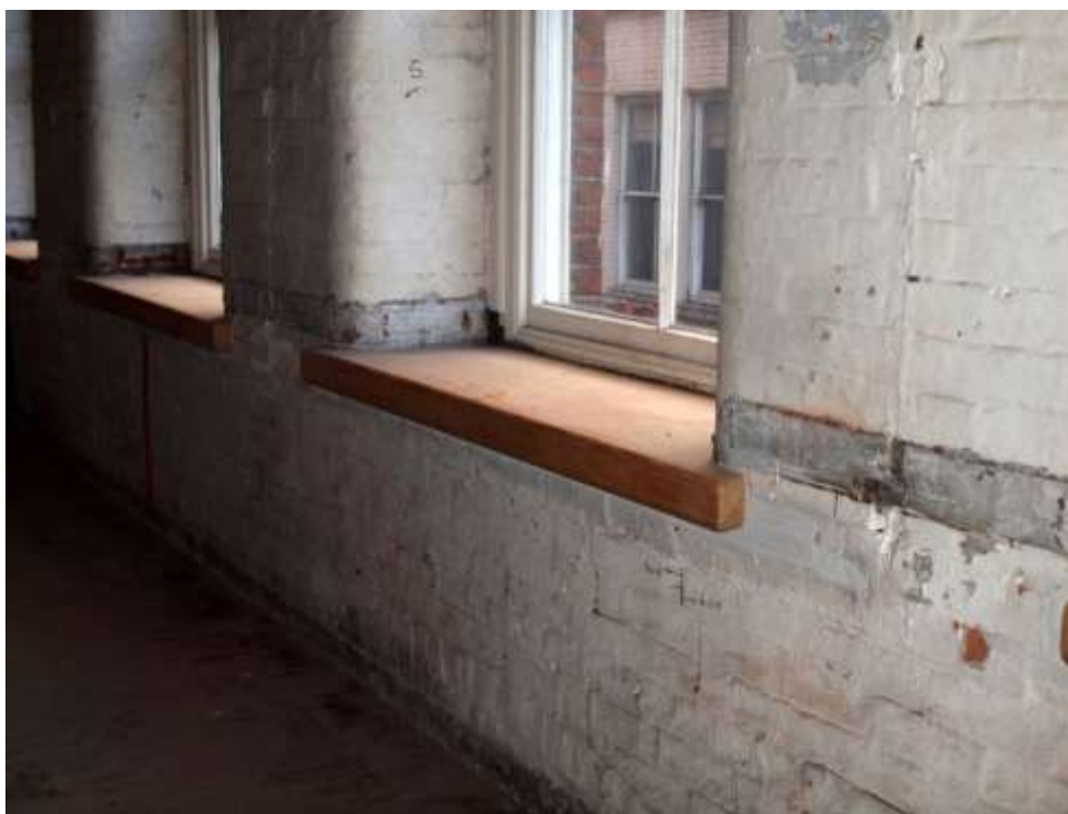
Plate 57: Detail showing replaced window cills
