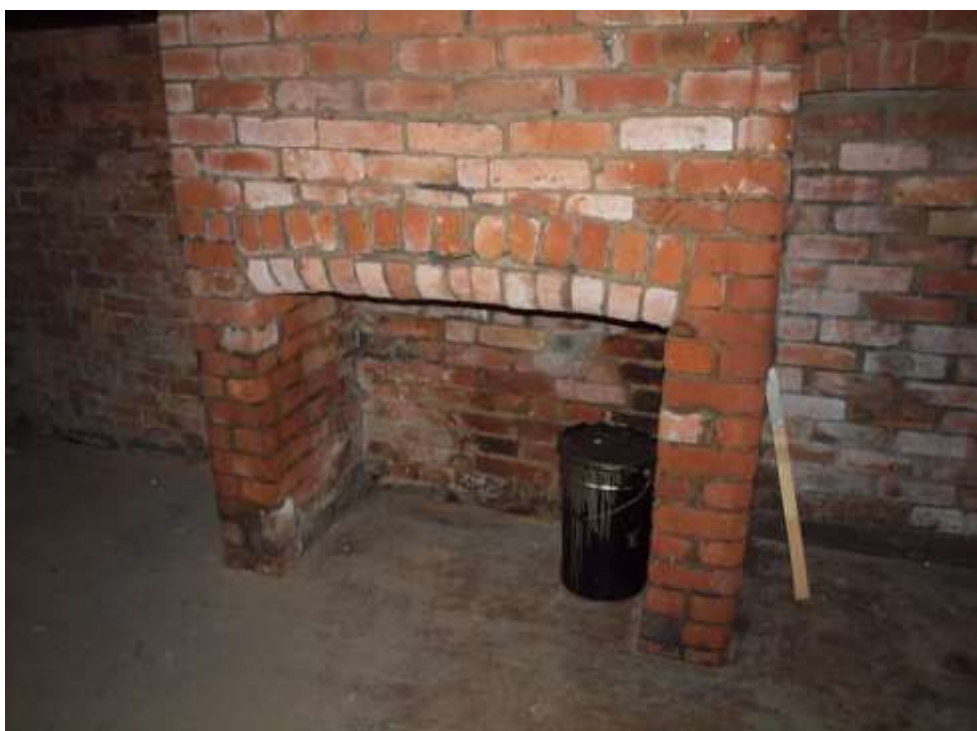
Plate 26: Detail of inserted fireplace
