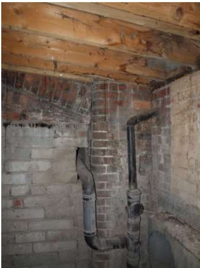
Plate 48: Detail of west end of raised floor above loading bay
