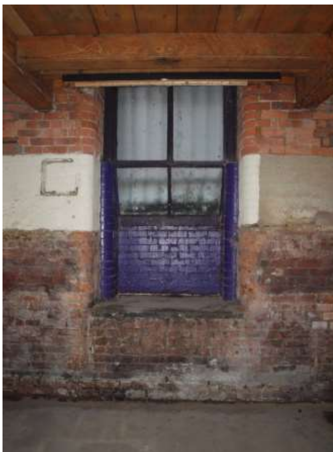
Plate 27: Detail of cellar light
