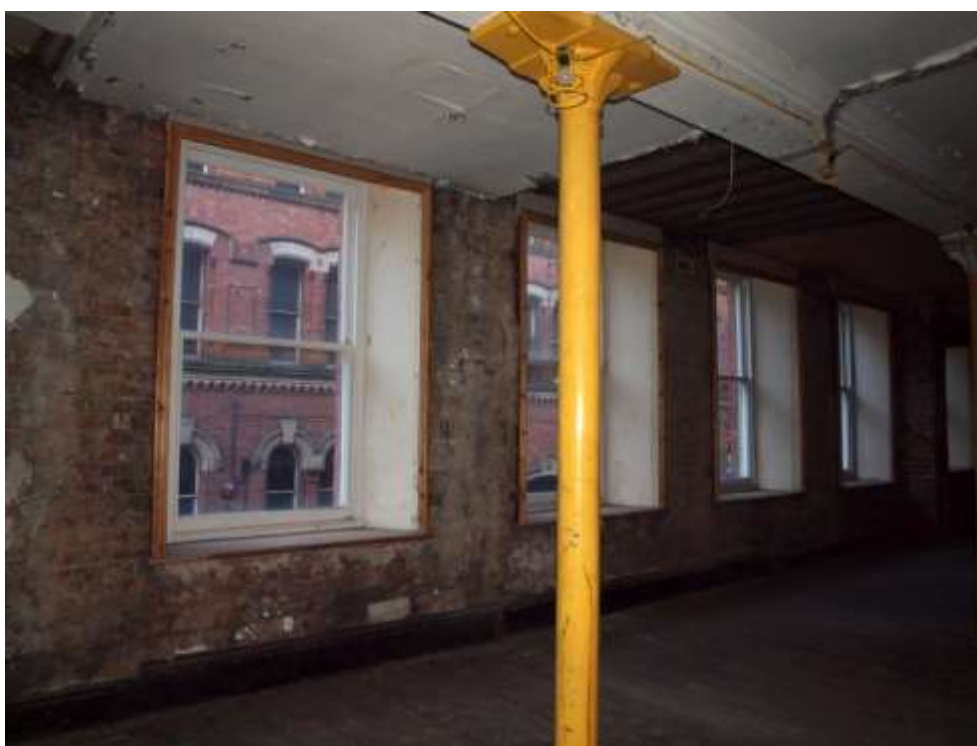
Plate 54: Detail of windows with replaced surrounds
