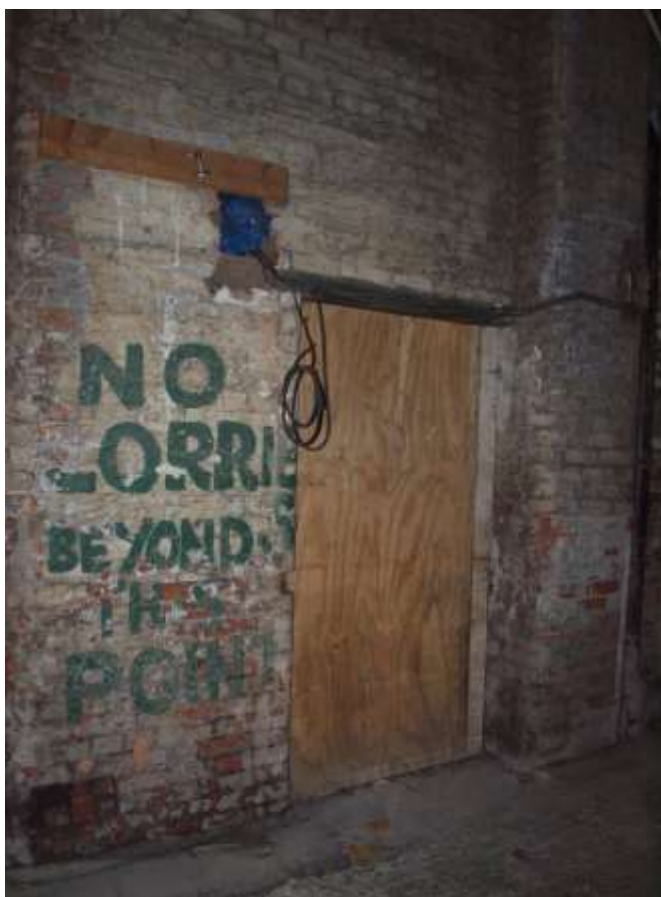
Plate 19: Blocked doorway in loading bay
