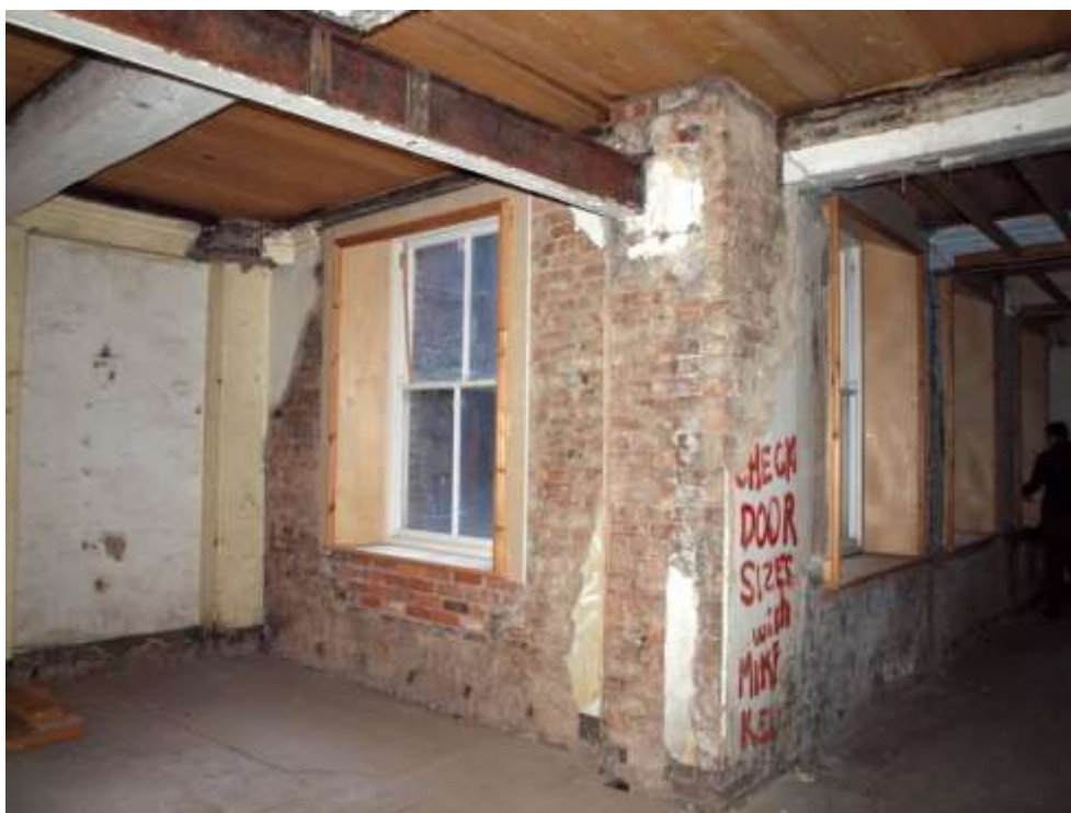
Plate 55: Northwest corner of first floor
