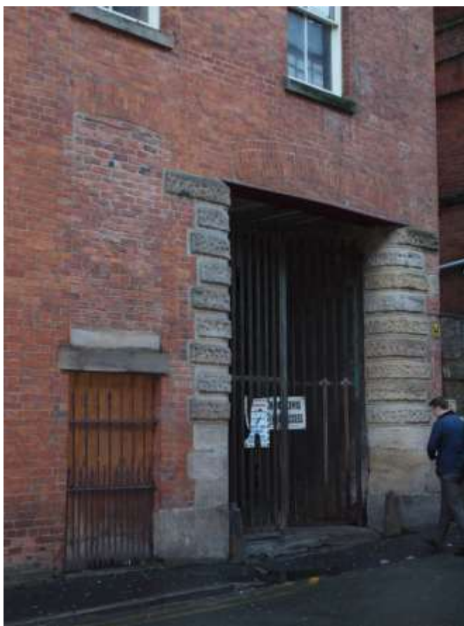
Plate 11: Loading doorway at north end
