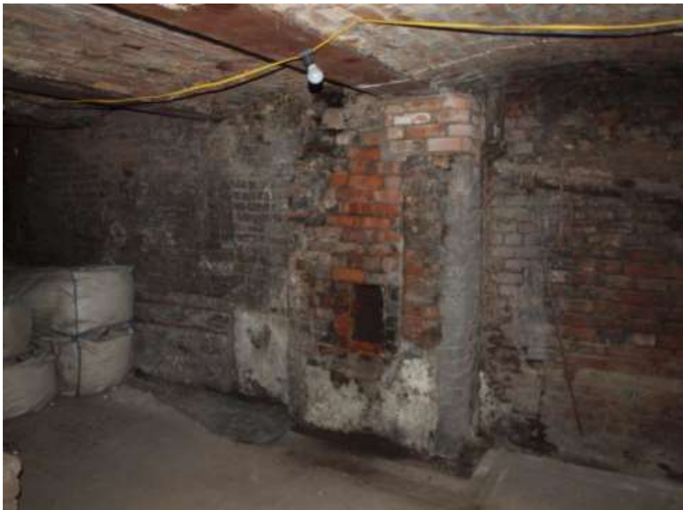
Plate 32: Detail of pillar with grated opening in sub-basement. Note the straight joint in the wall to the left of it
