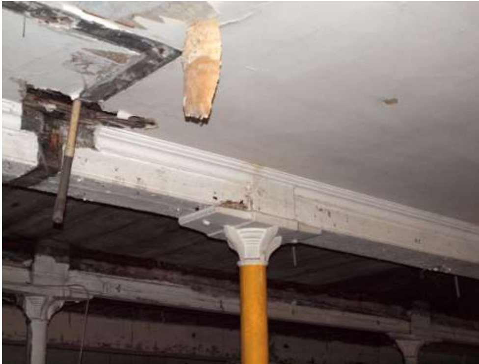
Plate 61: Lath and plaster ceiling and remains of cornicing
