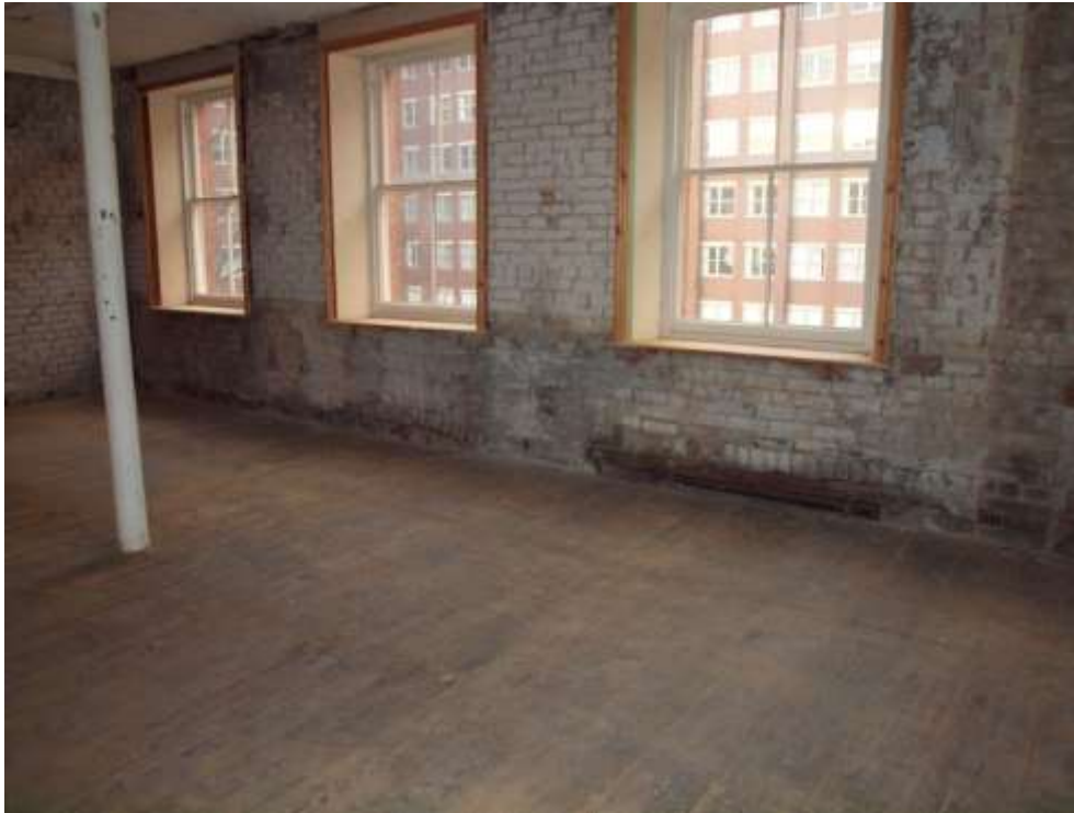
Plate 69: Detail of windows with lintels of the lower floor windows visible just above the floor
