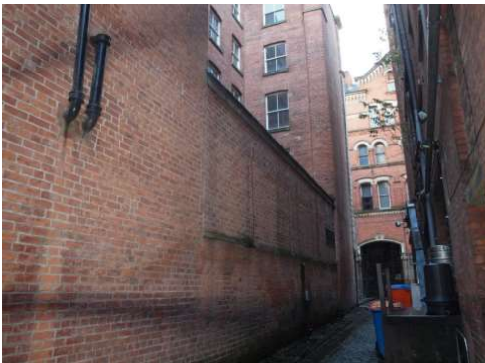
Plate 13: Ground floor north elevation
