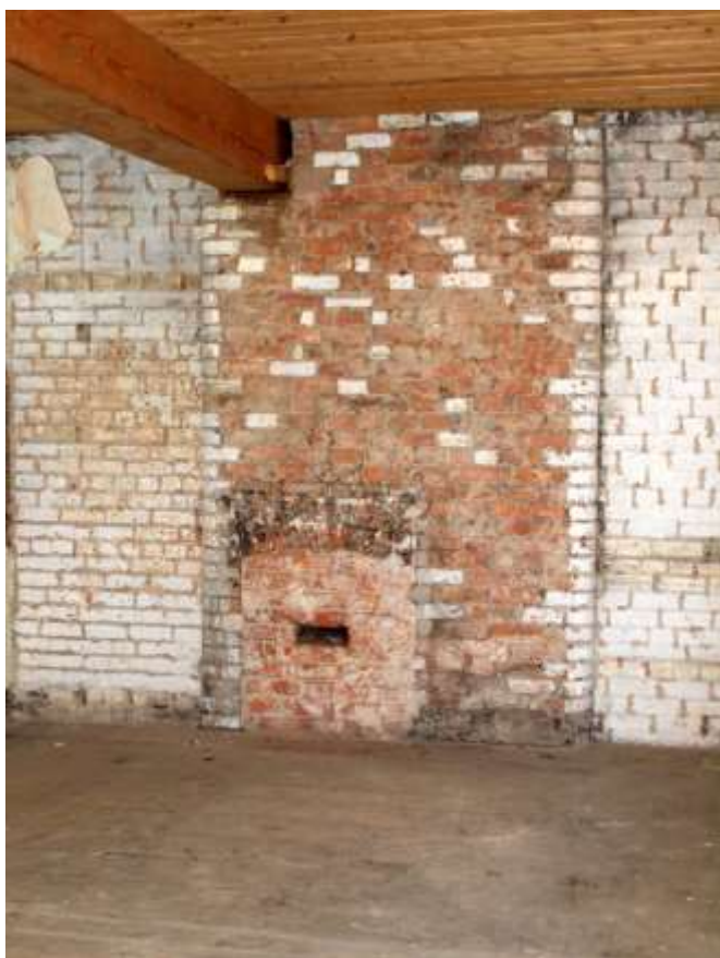
Plate 77: Blocked fireplace in southwest corner
