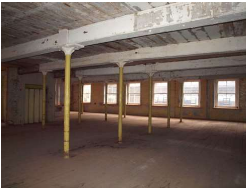
Plate 68: General shot of the second floor
