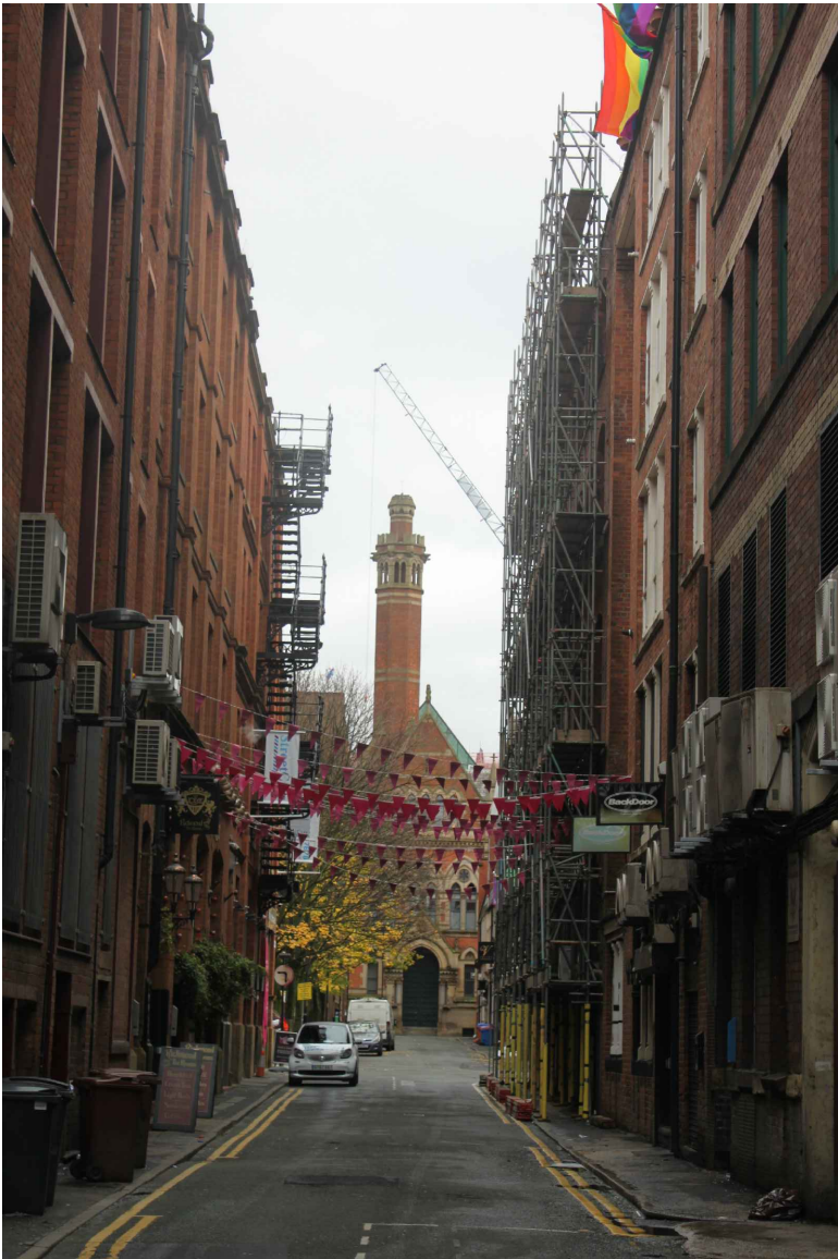
Existing Street View 8
