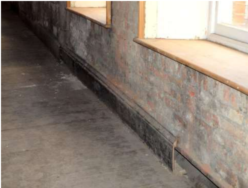
Plate 60: Detail of remains of timber skirting
