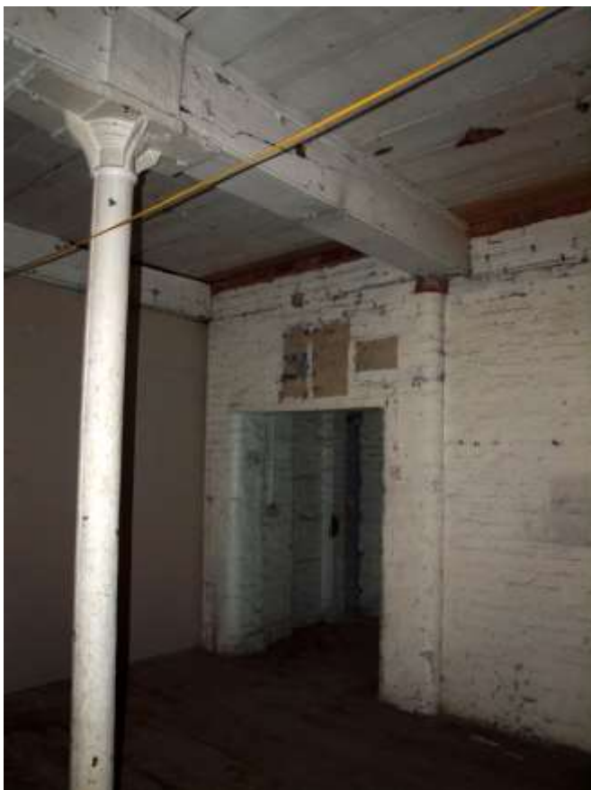
Plate 66: Opening to the east of the safe with arched lintel visible
