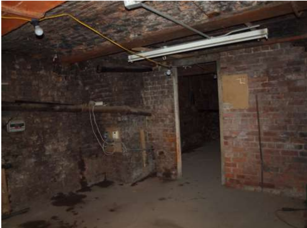
Plate 31: Inserted dividing wall in sub-basement
