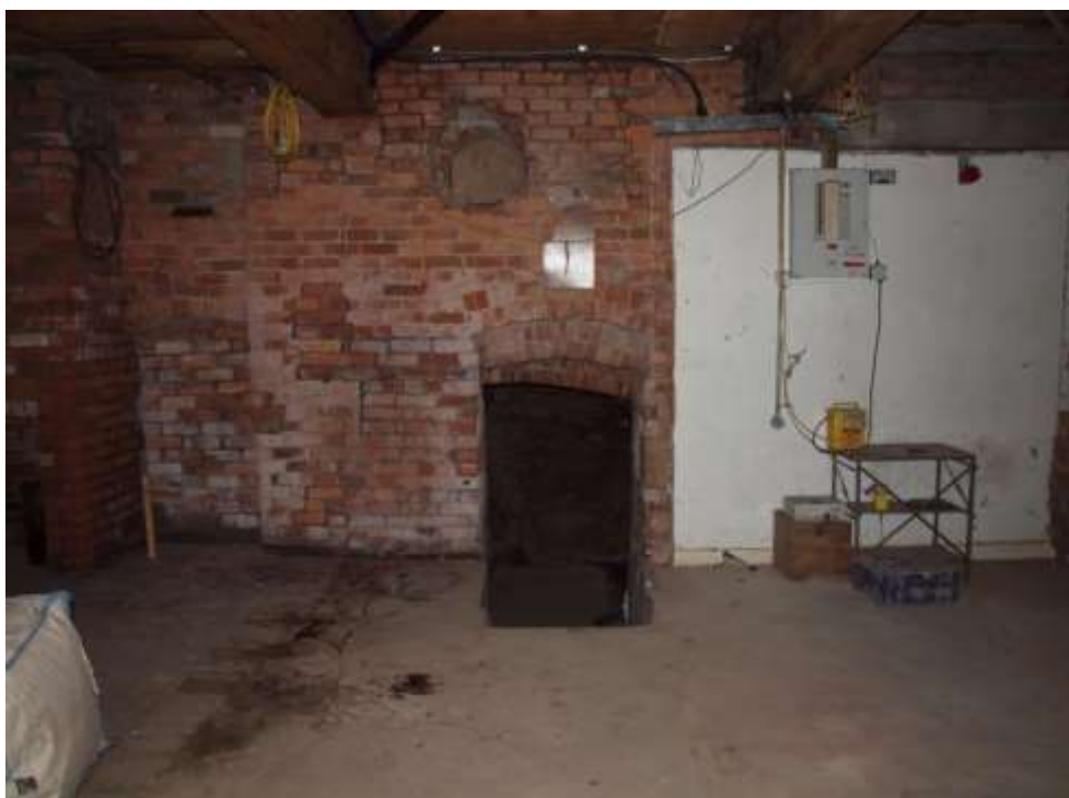
Plate 25: Detail of sub-basement entrance
