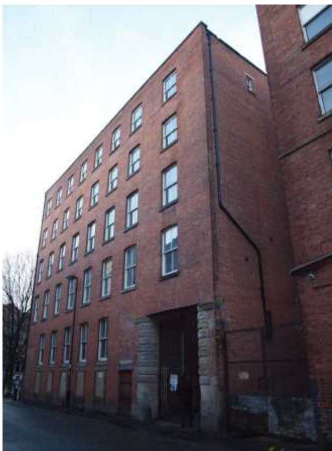
Plate 7: Richmond Street elevation
