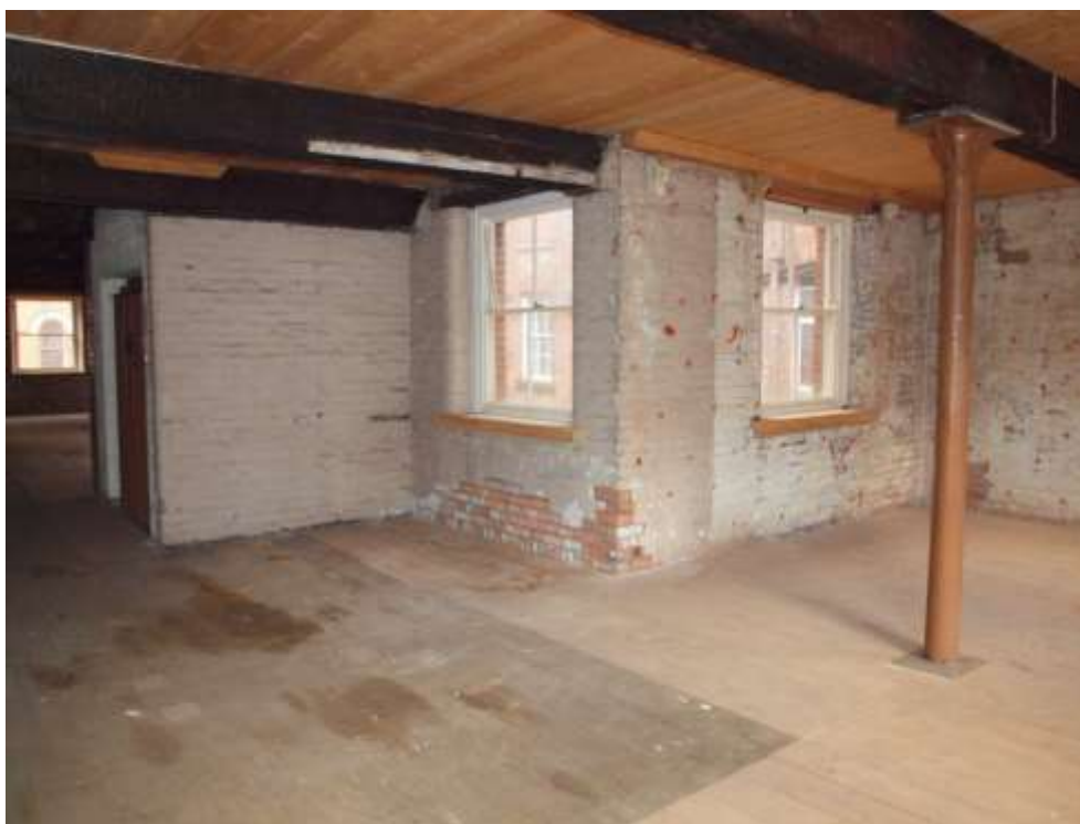
Plate 82: North east corner of the floor showing repairs
