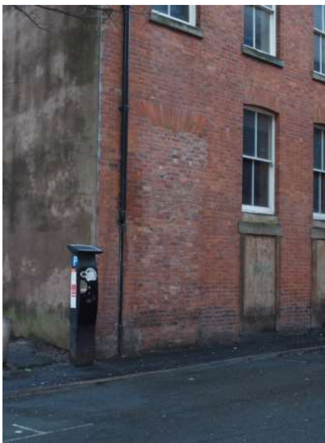
Plate 10: Blocked opening at southern end
