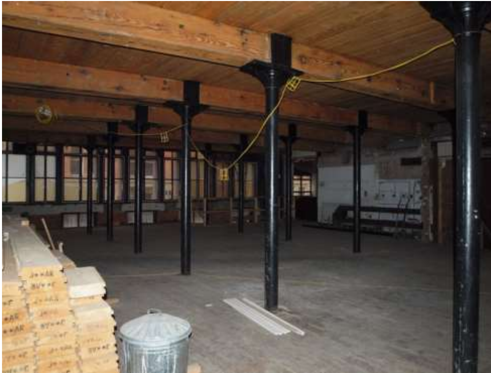
Plate 43: General shot of ground floor showing stanchions and replaced timber
