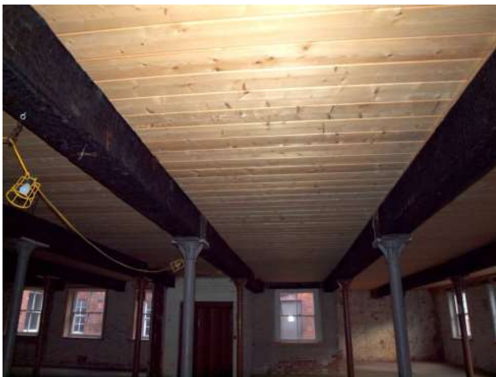
Plate 76: Replaced timber boards of ceiling
