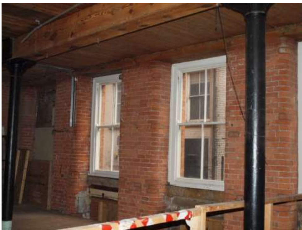
Plate 45: Detail of windows facing Richmond Street
