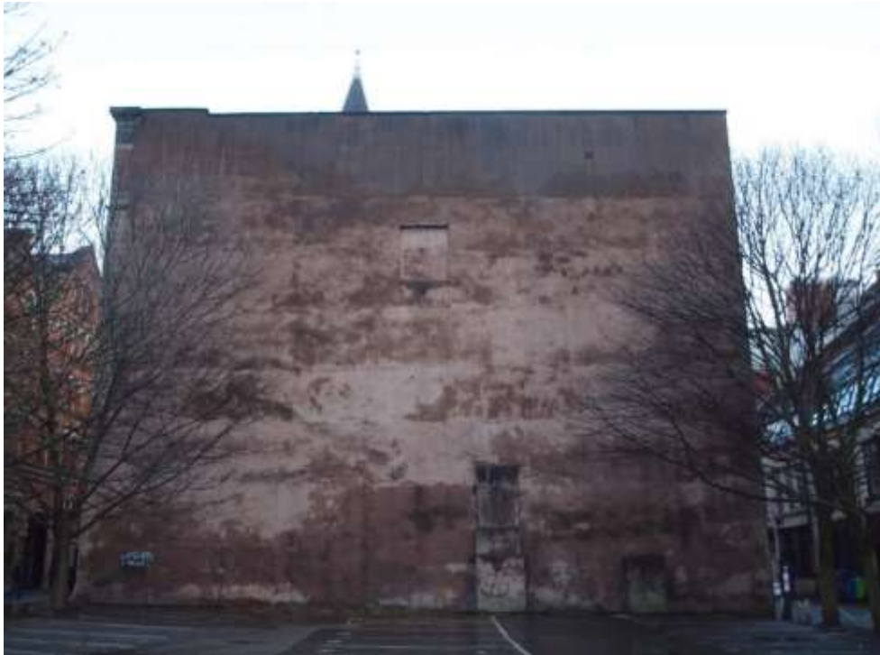
Plate 5: Southern elevation with blocked window
