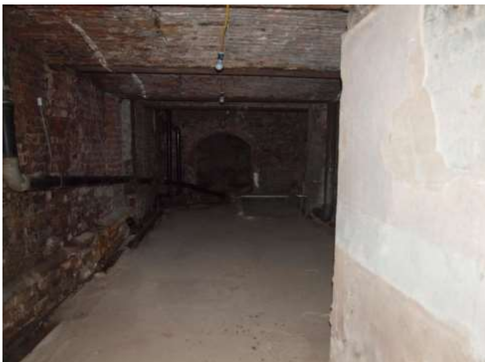
Plate 33: East end of sub-basement showing arched opening in east wall.
