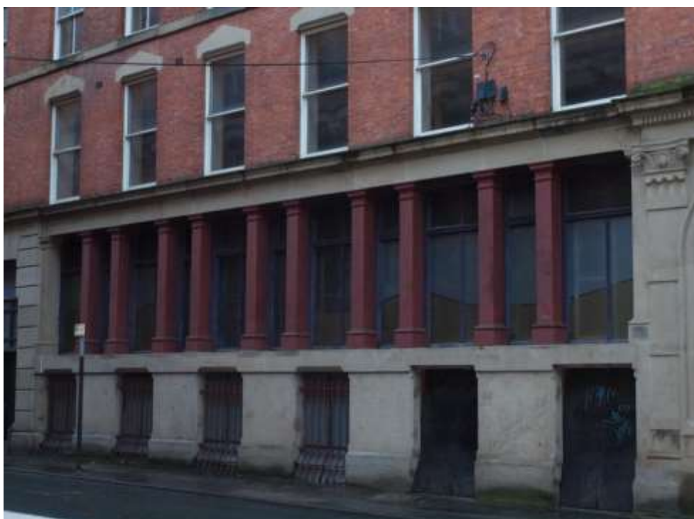
Plate 4: Fenestration and colonnaded screen
