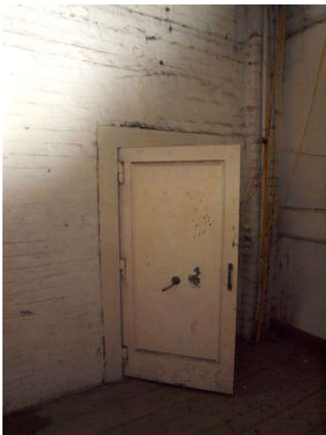
Plate 67: Detail of safe door.
