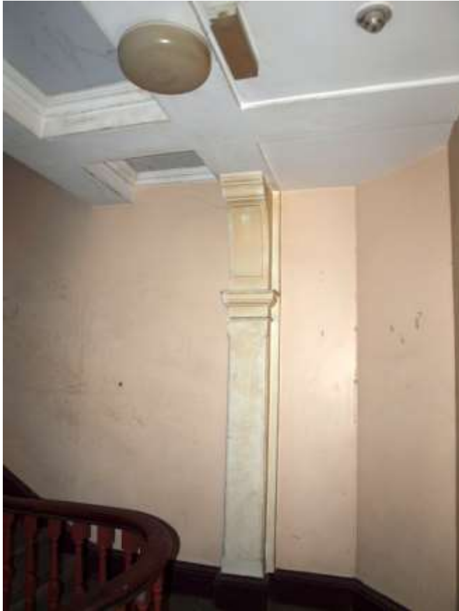
Plate 49: First floor landing showing plastered pillar and ceiling detail
