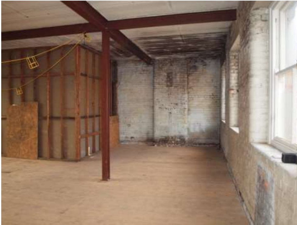
Plate 87: Modern screen surrounding main stairwell
