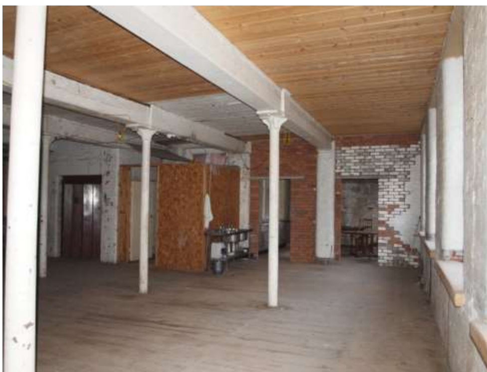
Plate 56: Inserted brick wall forming offices
