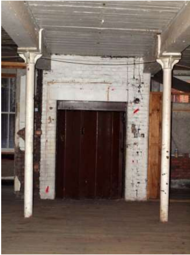
Plate 59: Inserted lift shaft on north wall
