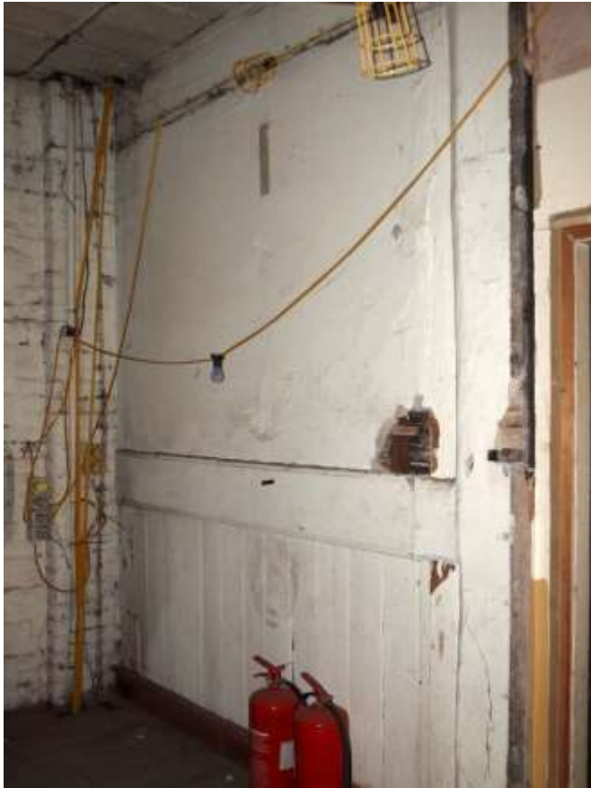
Plate 51: Detail of timber and lath and plaster wall.
