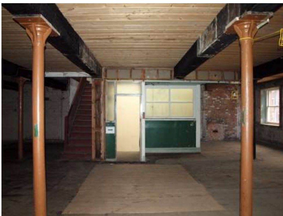
Plate 80: Modern entrance to staircase
