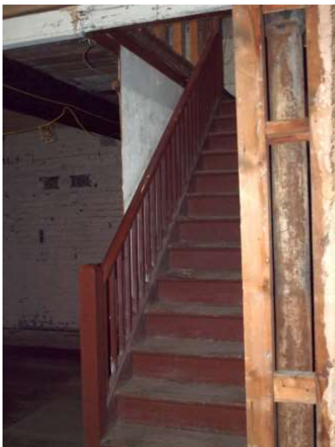
Plate 81: Inserted staircase to fourth floor
