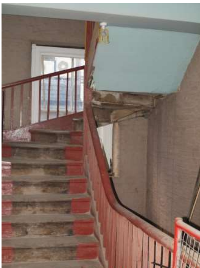
Plate 58: Southern inserted staircase crossing window
