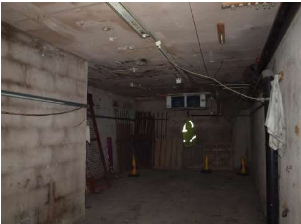
Plate 18: West end of loading bay entrance
