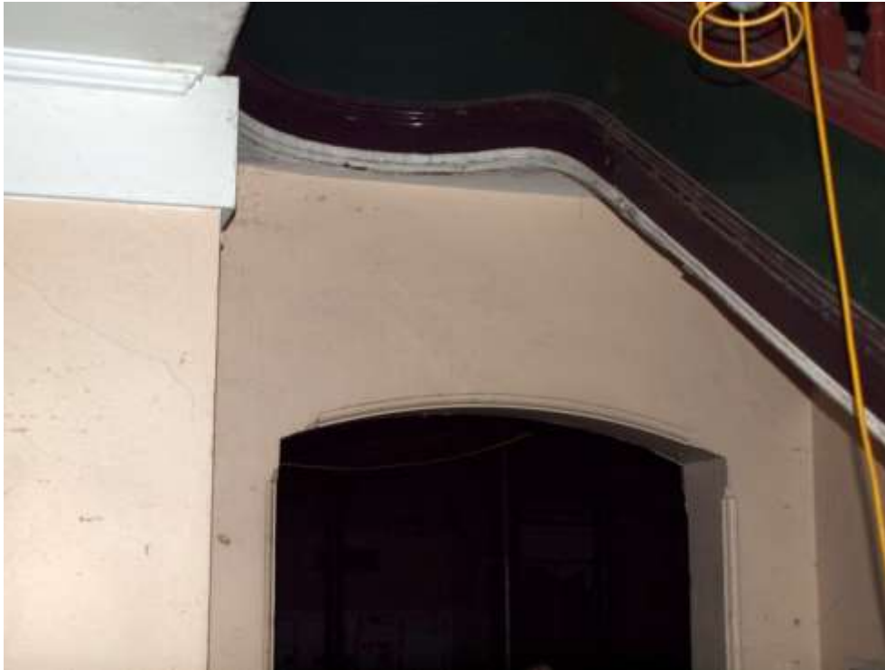
Plate 41: Detail of northern doorway chamfered jamb and cornice within lobby
