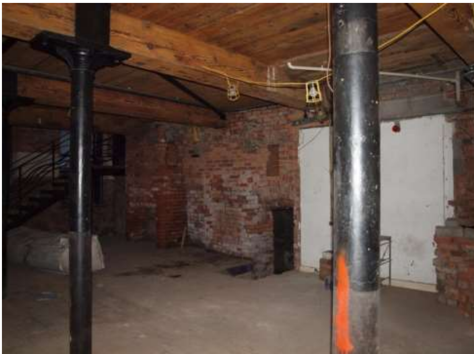
Plate 24: East wall showing (from left to right) inserted staircase, inserted fireplace and entrance to sub-basement
