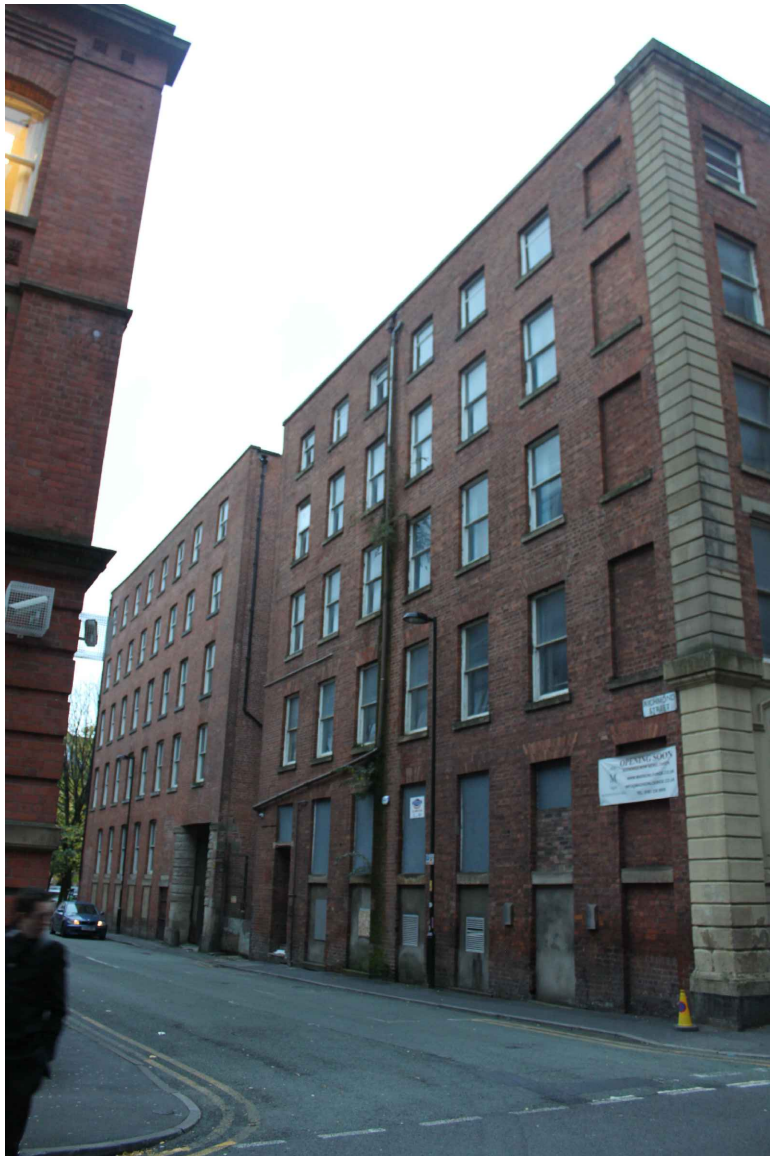
Existing Street View 7
