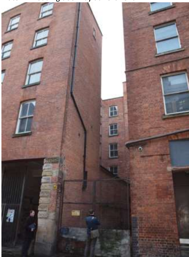
Plate 12: North elevation within yard
