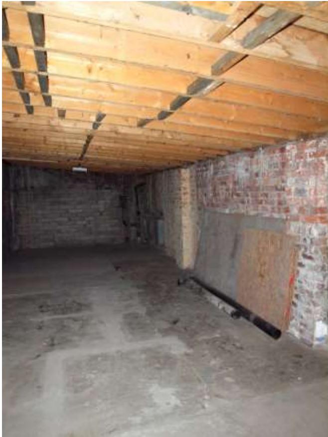
Plate 47: Raised ground floor level above loading bay
