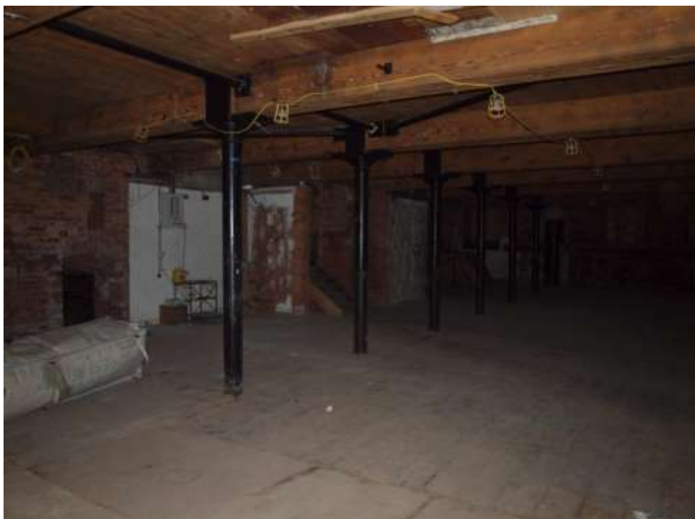
Plate 28: Shot of basement east wall showing (from left to right) doorway to sub-basement, staircase from loading bay and inserted lift shaft
