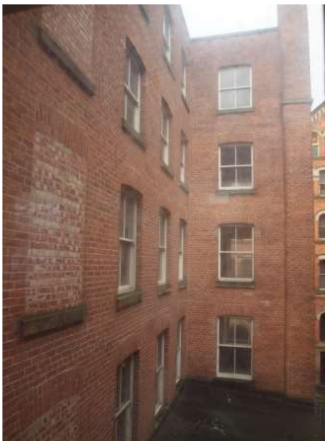
Plate 15: North elevation as viewed from the interior
