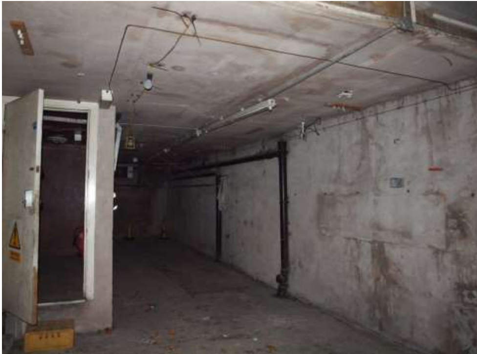
Plate 17: Street level loading bay entrance
