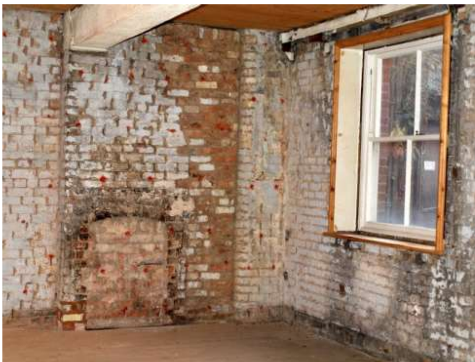
Plate 78: Blocked fireplace in northwestern corner
