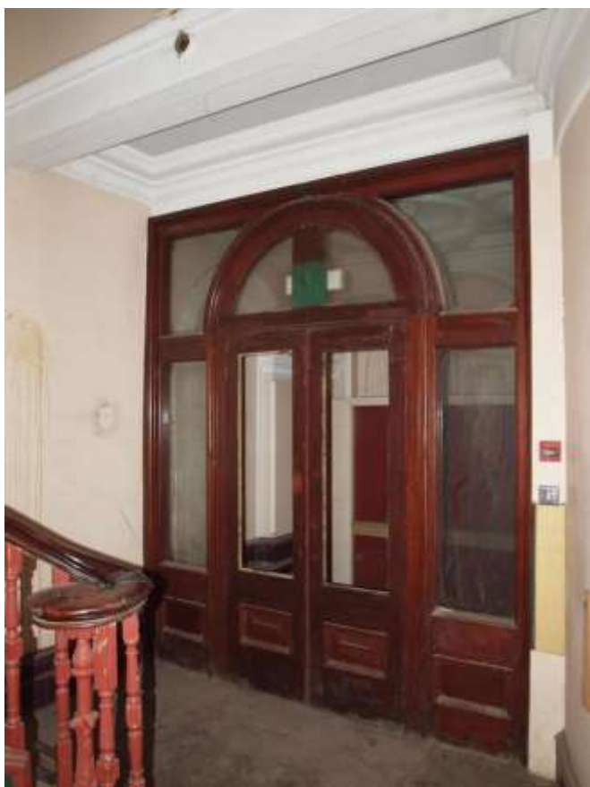
Plate 34: Interior doorway to porch
