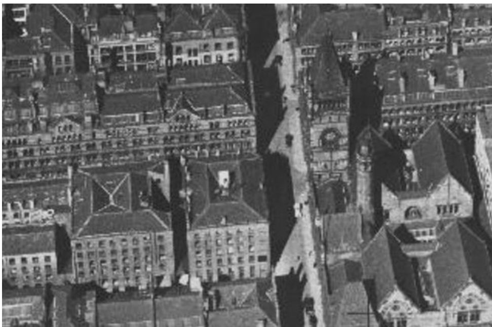
1950's Aerial Photograph showing the original roof to 11 Bloom Street.
