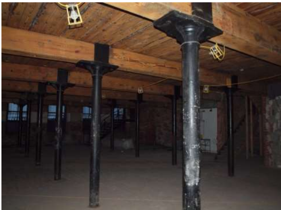
Plate 20: Basement showing columns
