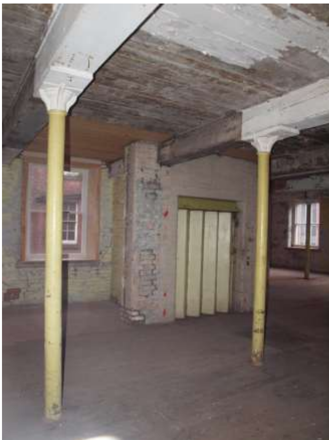
Plate 74: Inserted lift shaft with replaced boards in the ceiling to the left
