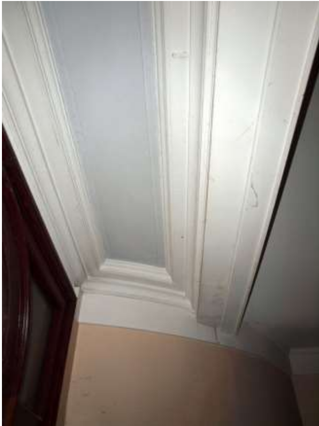
Plate 39: Detailed ceiling in lobby
