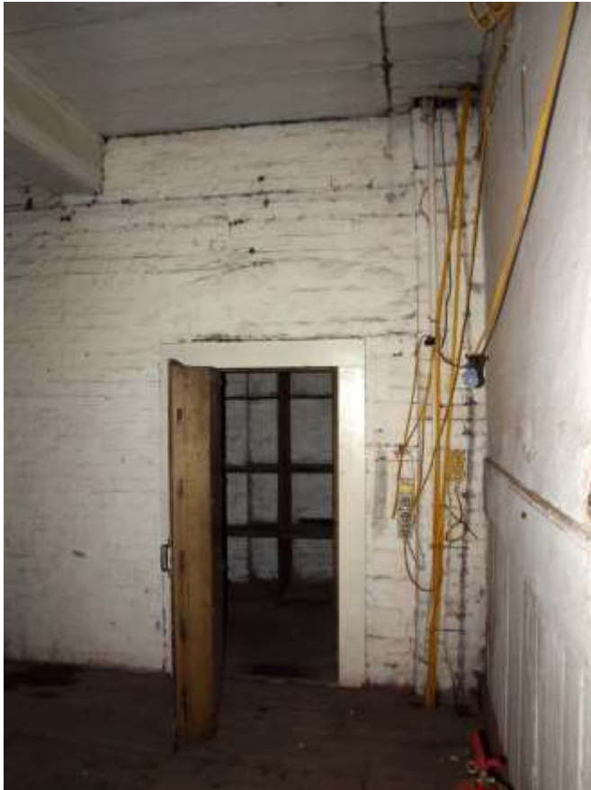
Plate 65: Entrance to safe
