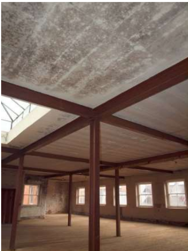
Plate 84: General shot of fourth floor showing RSJ and concrete construction
