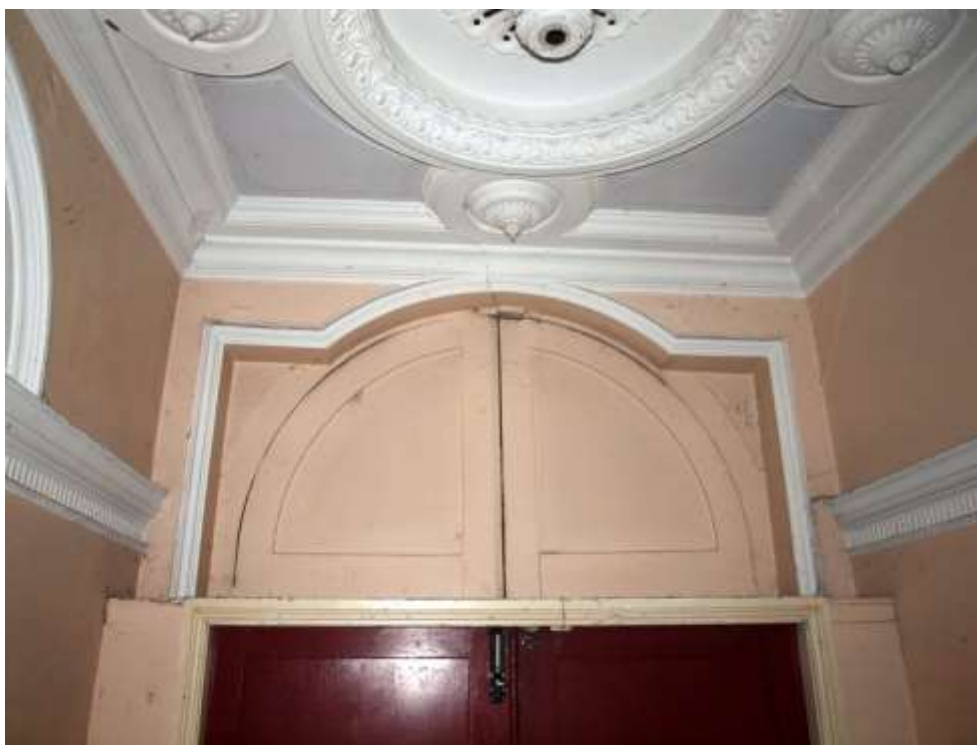
Plate 37: Detail of blocked lights above main entrance
