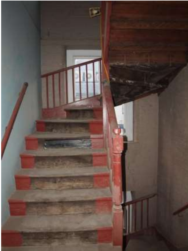
Plate 73: Inserted staircase cutting across window
