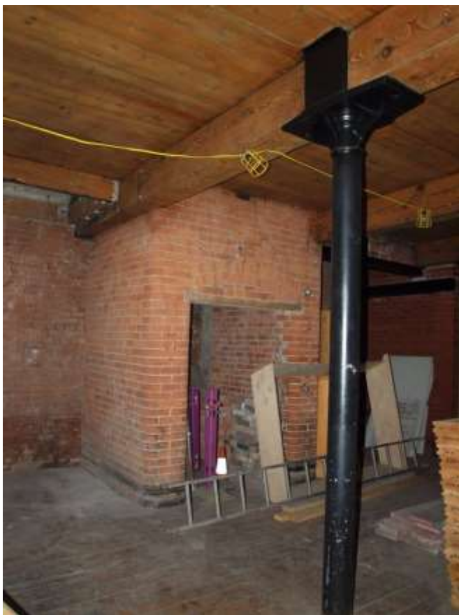
Plate 44: Inserted brick shaft on west wall
