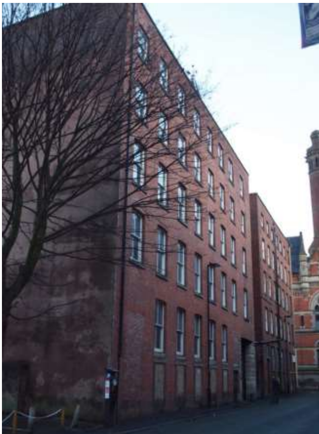
Plate 6: Richmond Street elevation
