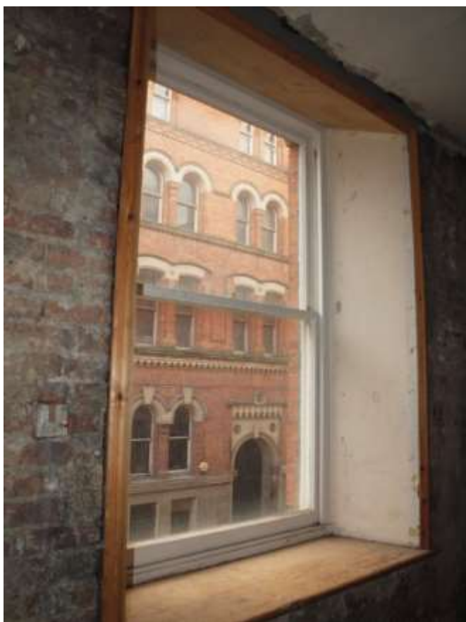
Plate 64: Detail of window surrounds
