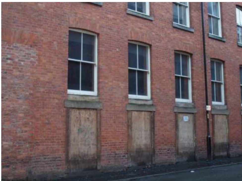
Plate 9: Ground floor windows and cellar lights
