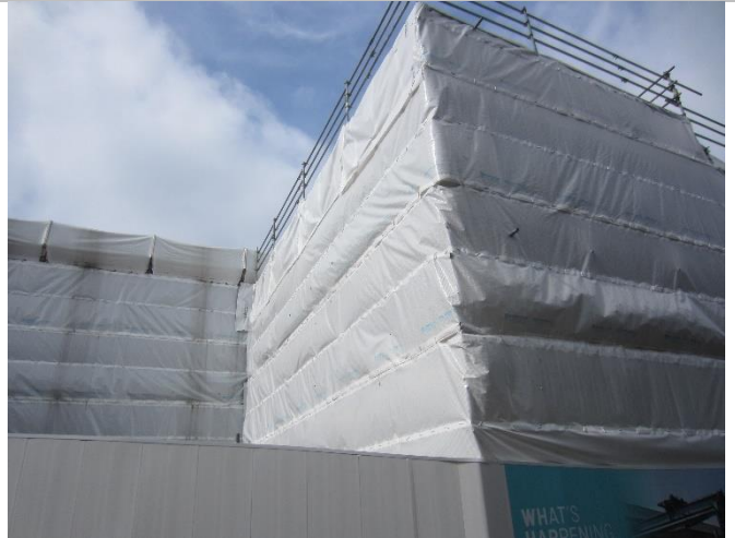
Photo 2: Northern elevation of the Power Hall showing the scaffold and canopy
