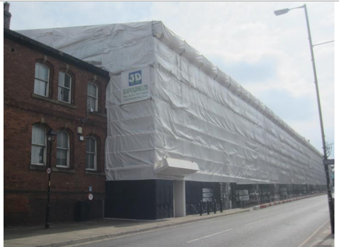
Photo 4: Southern and western elevations of the Power Hall showing the scaffold and canopy
