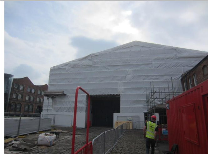
Photo 3: Western elevation of the Power Hall showing the scaffold and canopy
