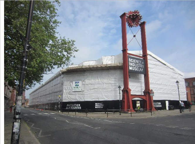
Photo 1: Southern and eastern elevations of the Power Hall showing the scaffold and canopy
