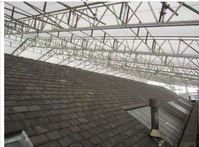
Photo 5: Southern roof pitch beneath the canopy
