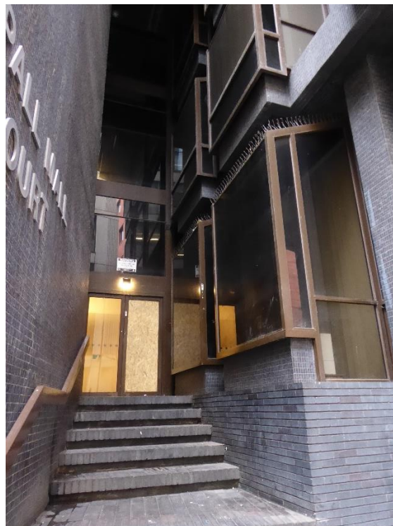
Figure 5: South elevation entrance
