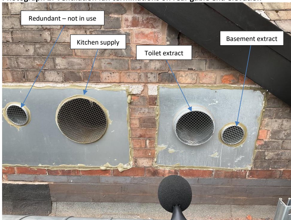
Photograph 2: Ventilation fan terminations on rear gable end elevation
