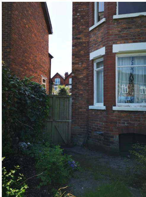
Rear view of left-hand side of existing bay and relationship with boundary to neighbour
