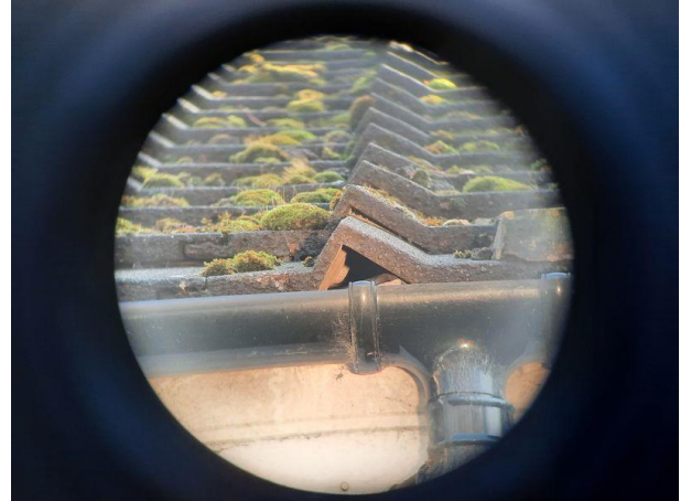
Plate 4.8: Opening Under Overhanging Profile Roof Tiles
