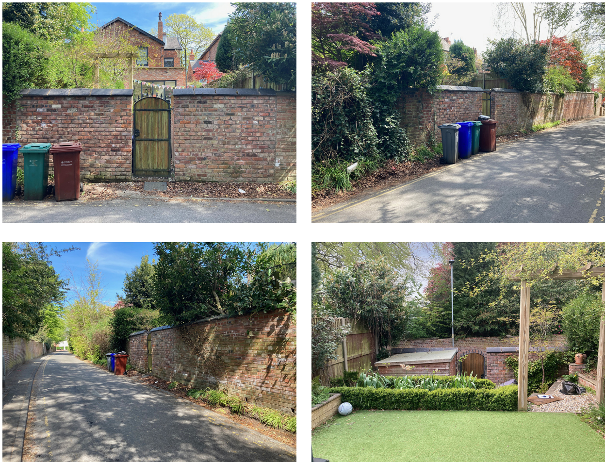
Existing Garden Wall
