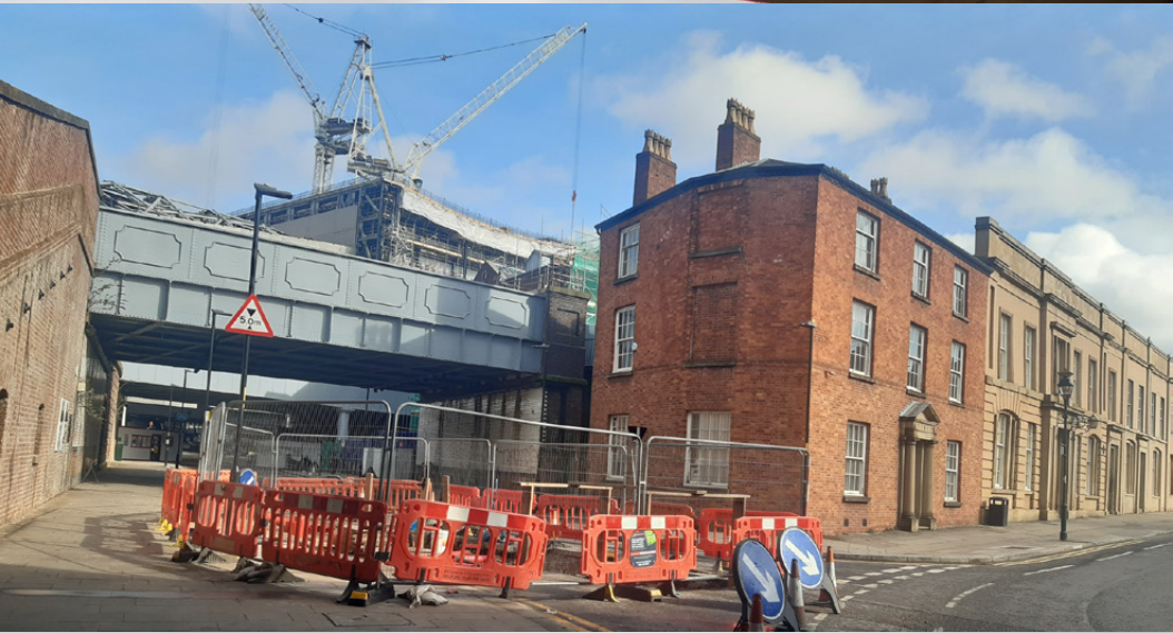
CURRENT VIEW (19/03/21) APPROXIMATING AVR 5A
