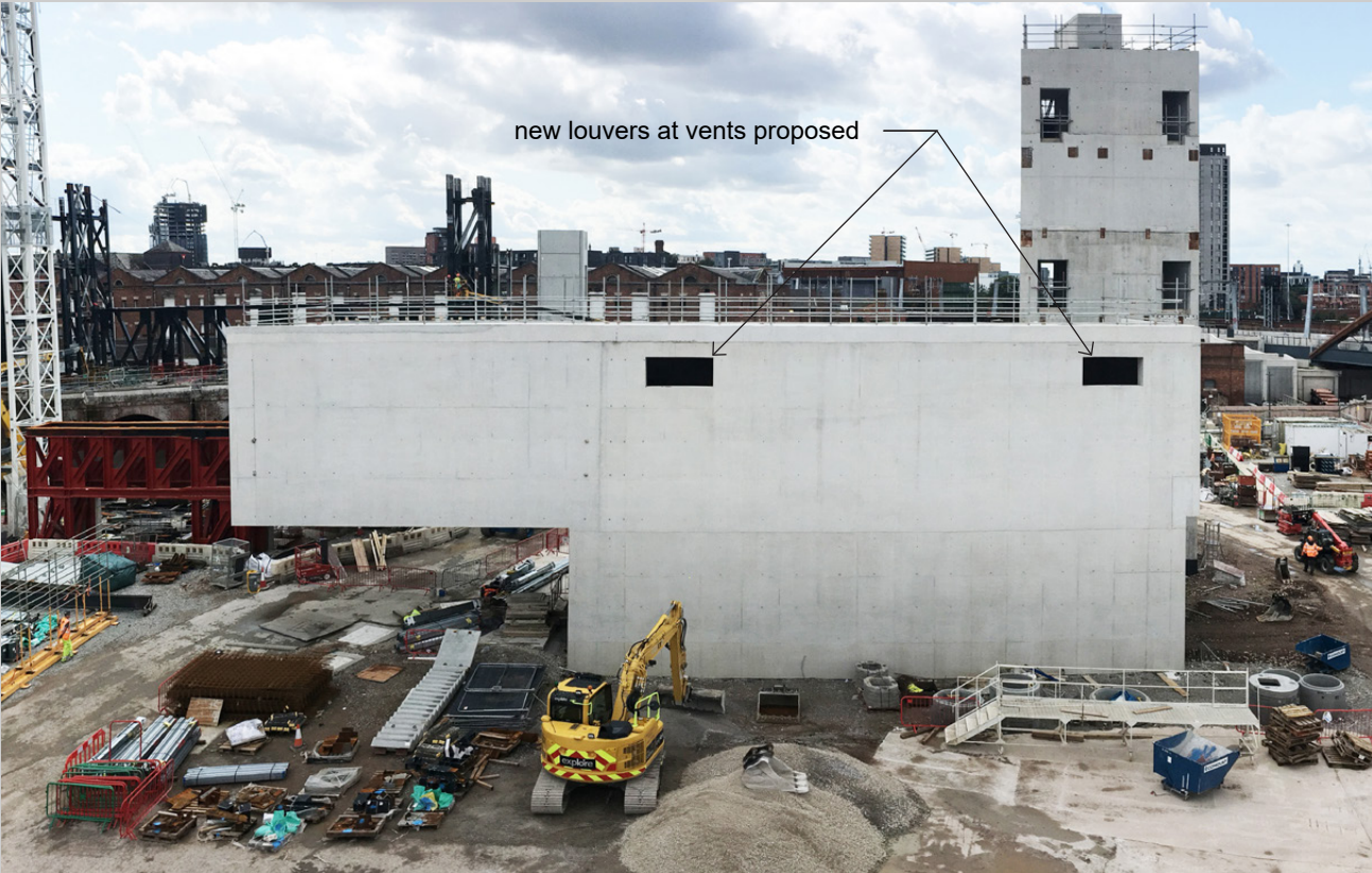
Truck lift - cast in place concrete constructed. photo from 12/2019
