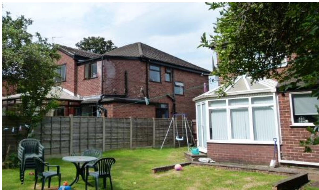
Rear of the site looking towards No.311 to the south
