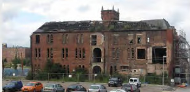
Picture showing the building with scaffolding
