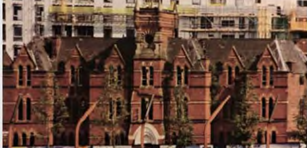
Picture showing building prior to demolition works
