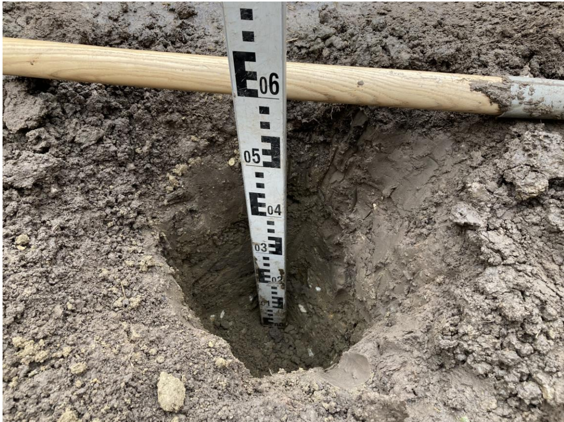
Photograph 3 200mm of topsoil and 400mm of subsoil emplaced in VP01.
