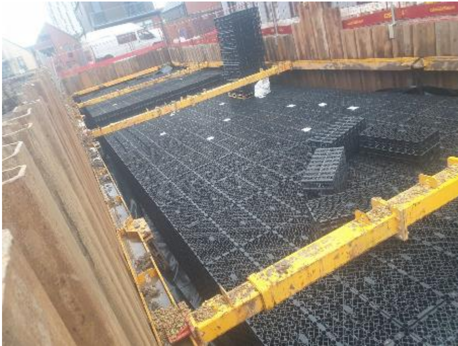
04FEB21 Tank Under Construction
