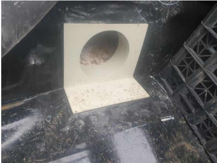
04FEB21 225mm Inlet Connection at Tank Invert Level – Inside View
