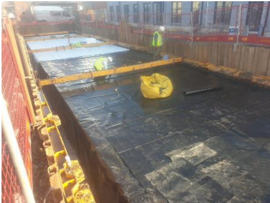
05FEB21 Geomembrane to Top of Tank
