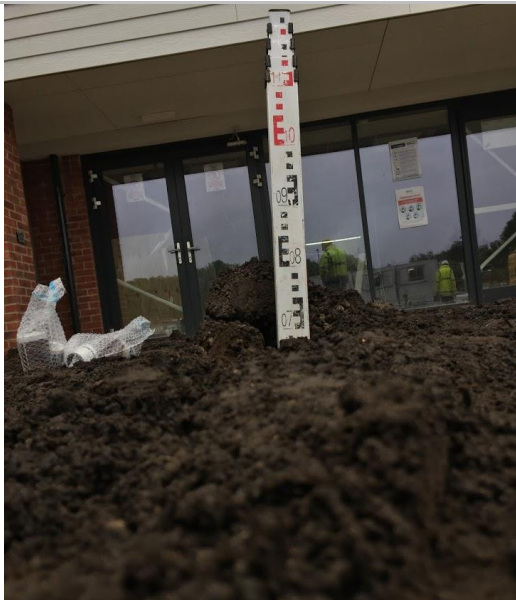
Depth of Cover System at Ground Level
