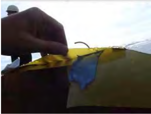
Photographs 1 and 2: Check general condition of membrane for punctures / tears etc
