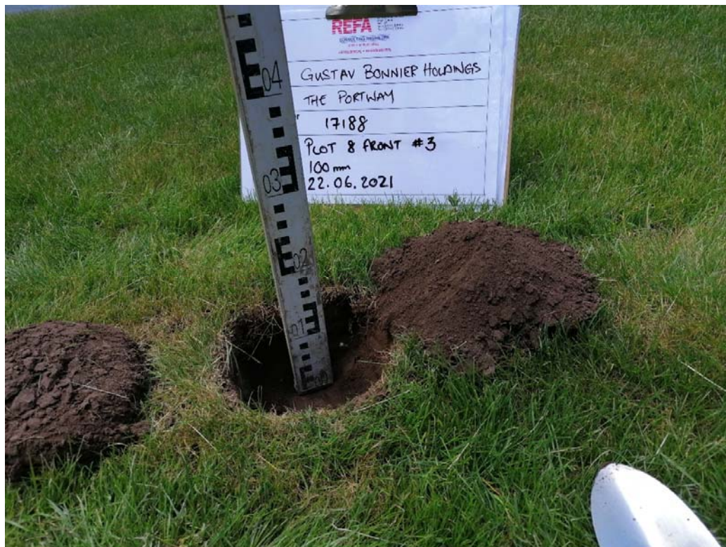
Photo 8 – At least 100mm of topsoil applied to front garden of plot 8
