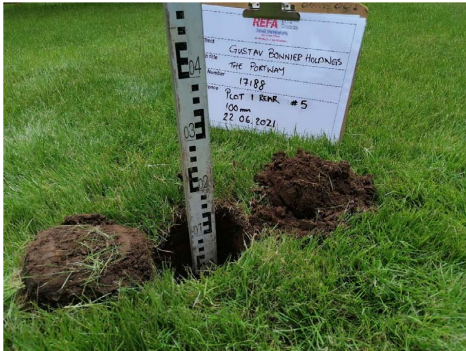
Photo 4 – At least 100mm of topsoil applied to rear garden of plot 1
