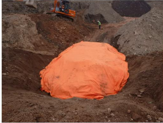
Pic 5 – Cell lining
