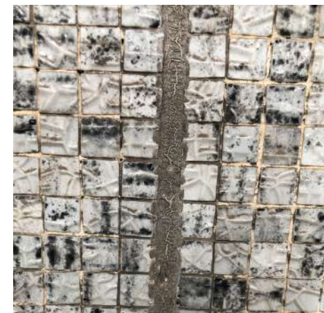
Original grey coloured movement joint between precast panels.
