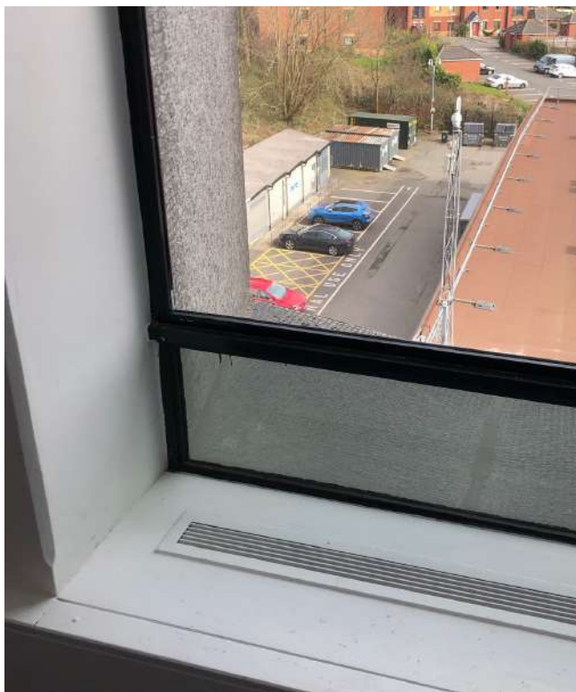
Existing crittal window detail - 30-40mm profile
