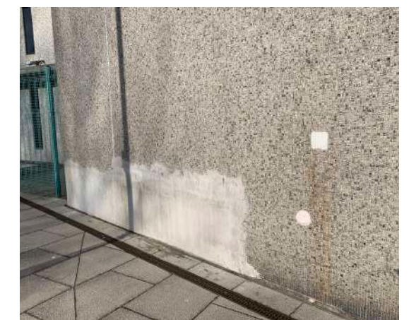
Replacement cladding panels to area of delamination
