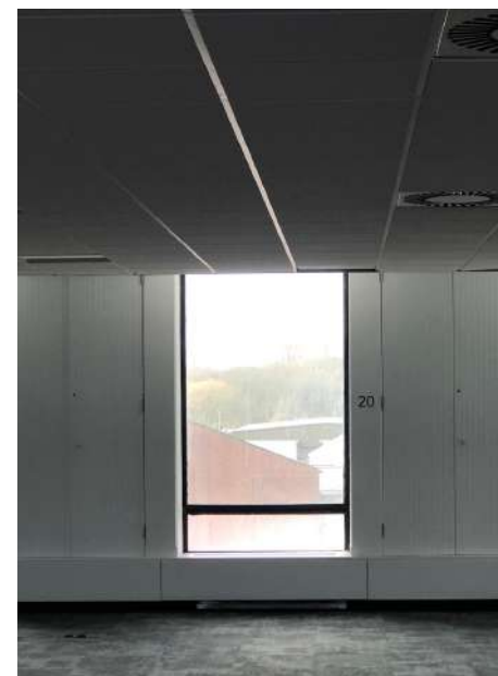
Existing suspended ceiling
