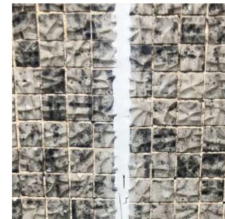
Non-original white coloured movement joint.
