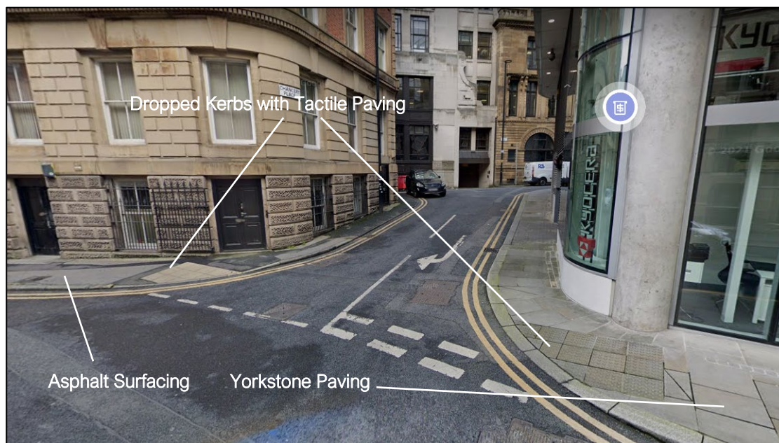
Figure 4.2 Tactile Paving at Chancery Place Junction with Booth Street
