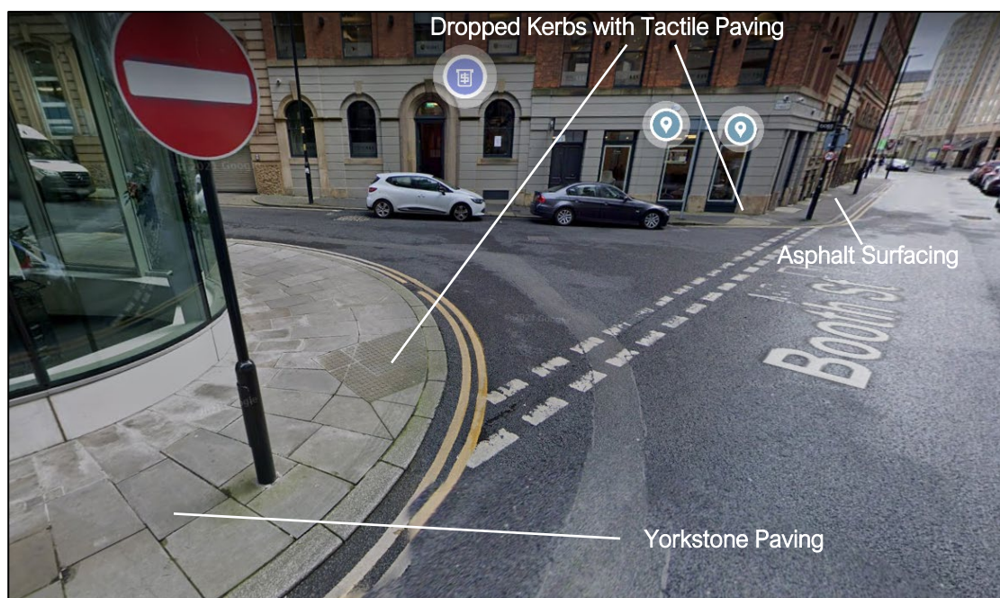
Figure 4.3 Footway Condition at Brown Street Junction with Booth Street
