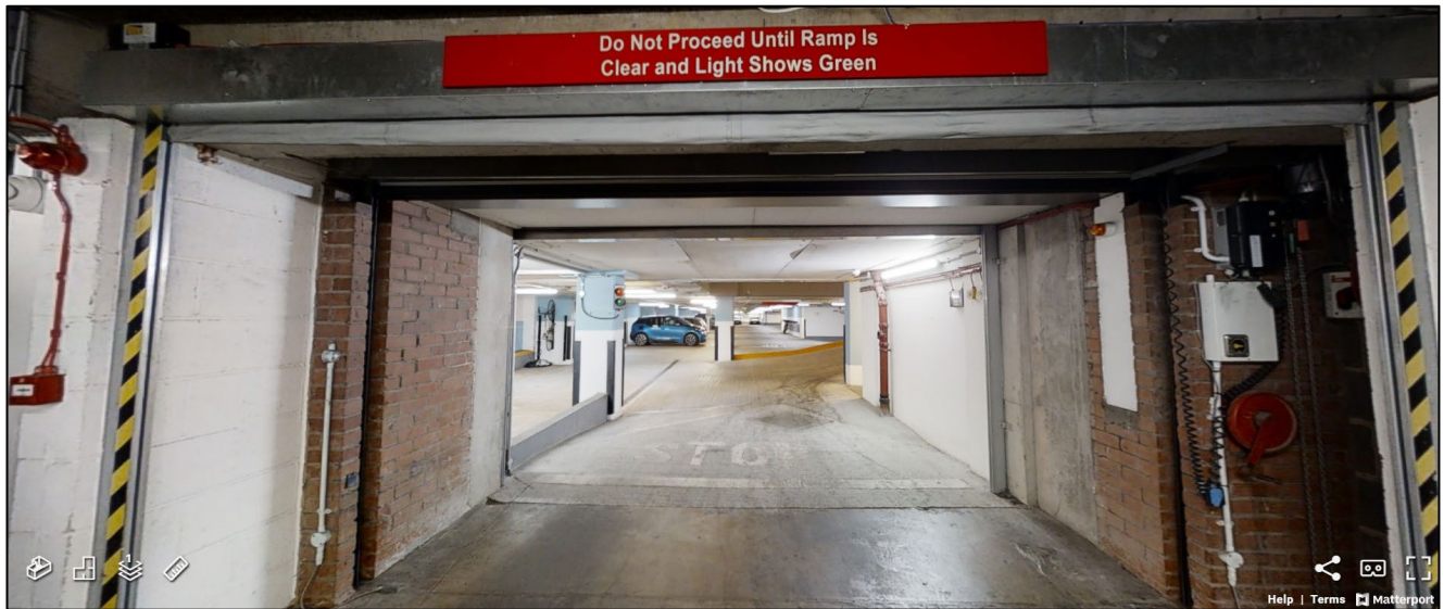
Figure 3.6 Egress of Basement Car Park (looking towards No12 Booth St Basement)
