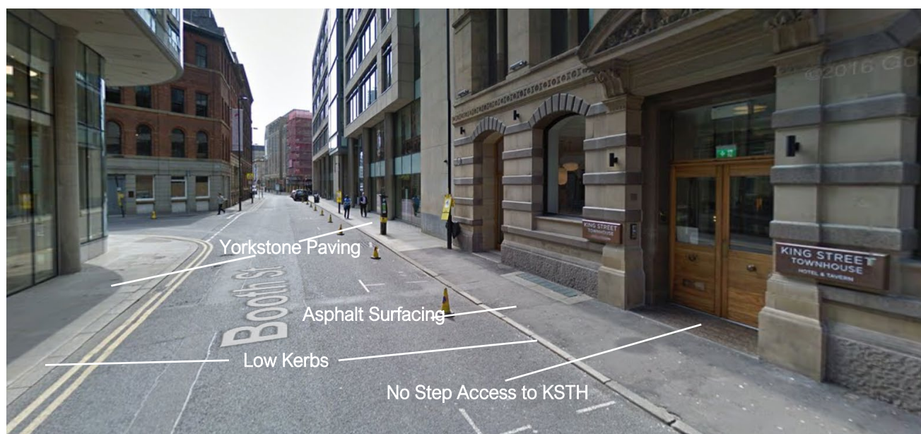
Figure 4.1 Footway Condition Booth Street o/s KSTH
