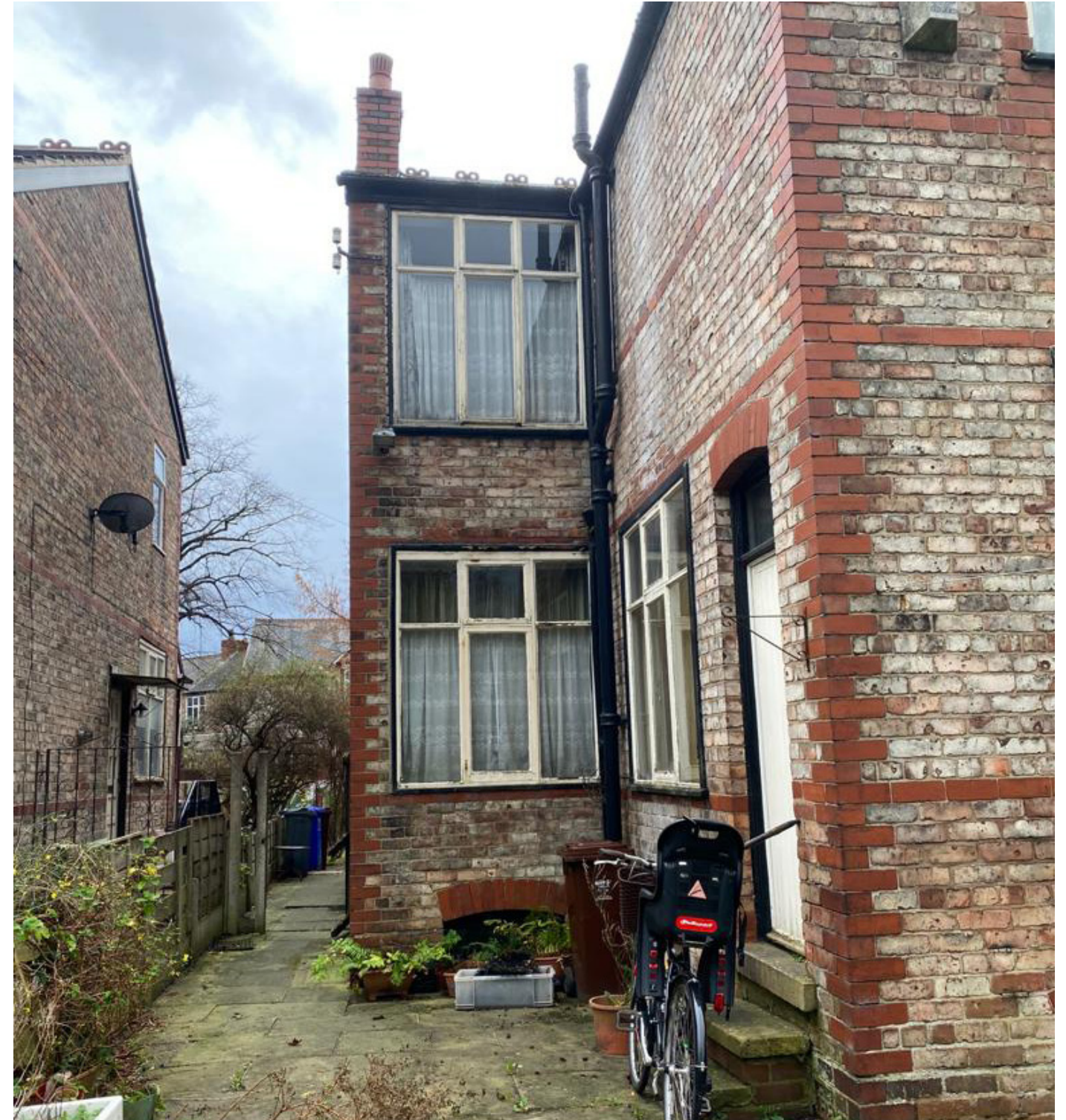
Fig. 4.4 100 Dudley Road - Rear View.
