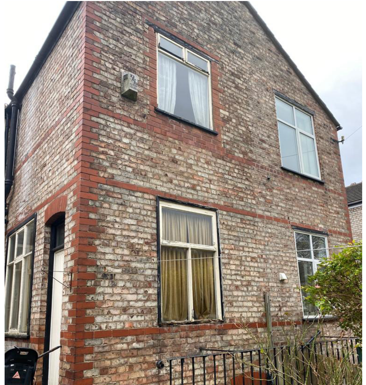
Fig. 4.2 100 Dudley Road - Rear View.
