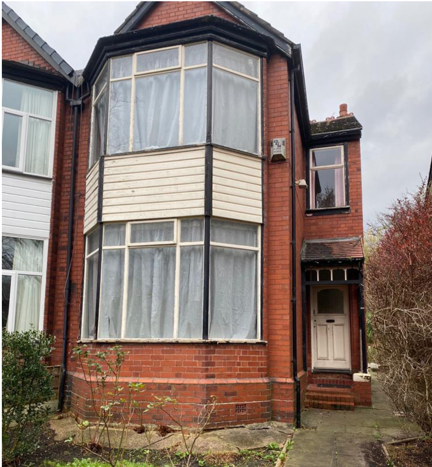
Fig. 4.1 100 Dudley Road - Front View.
