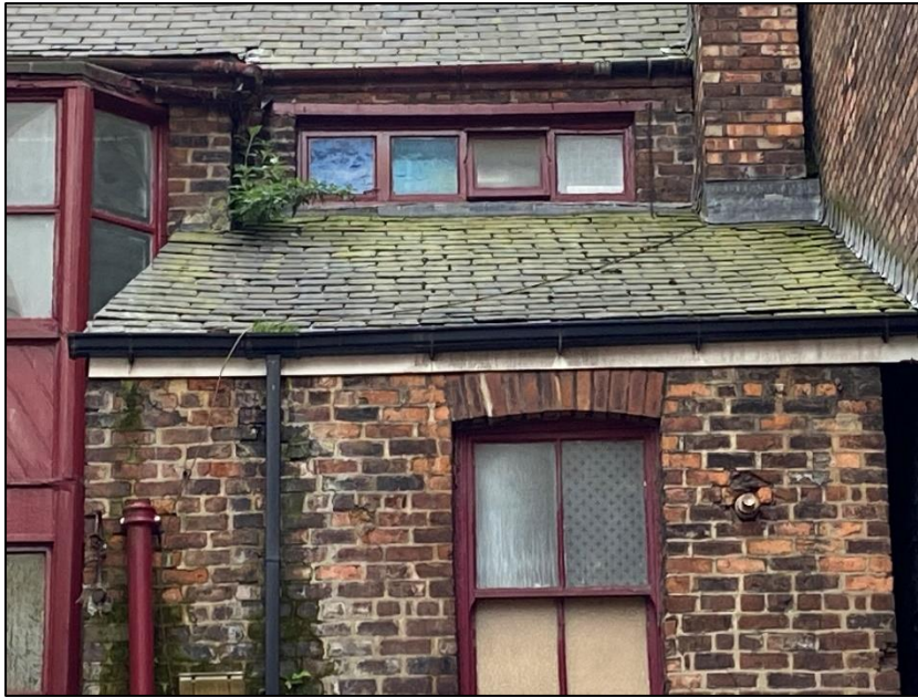
Photograph 4 showing the roof of the property
