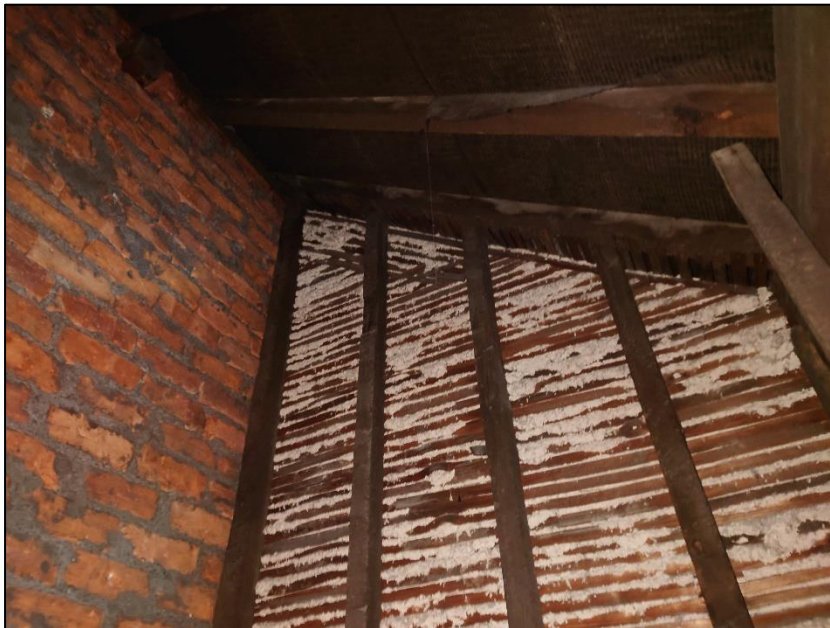
Photograph 5 showing the roof void
