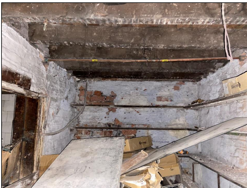
Photograph 7 showing the cellar space
