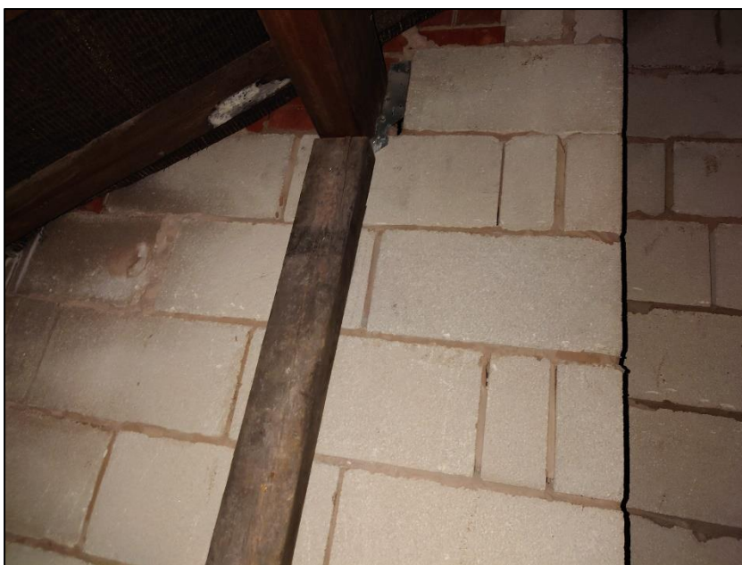
Photograph 6 showing the internal breezeblock inside the roof void
