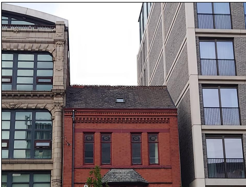
Photograph 3 showing the roof of the property
