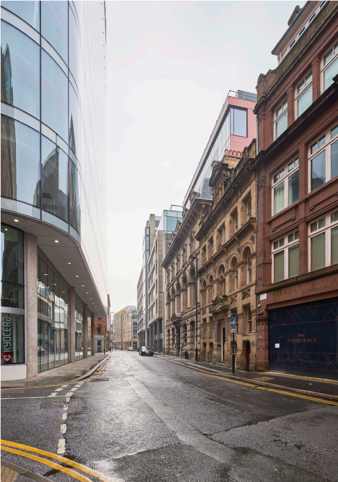
Existing Photo from Verified View Position - Booth Street West
