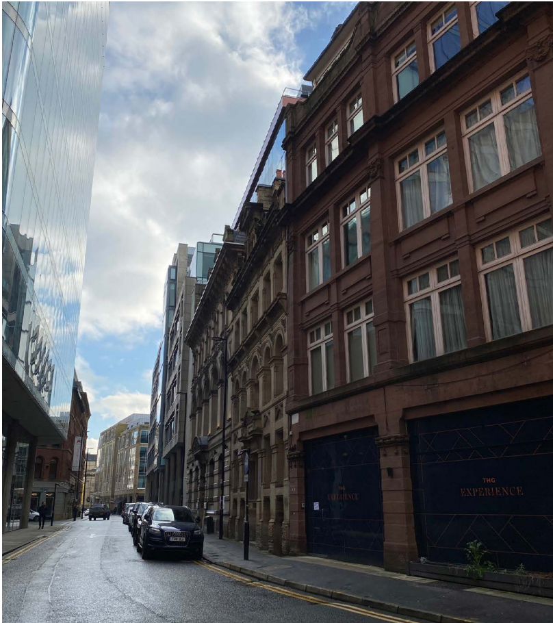
1 View South East from Booth Street
