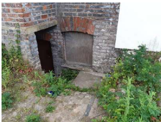
Basement beneath 309 Dickenson Road
