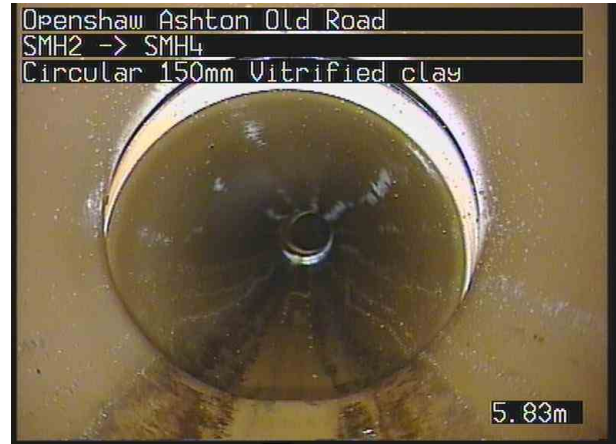
SMH2X_ca212ce1-1c5c-466d-986b-e1789575d57b_20210415_113131_235.jpg, 00:01:37, 5.83 m Joint displaced, medium
