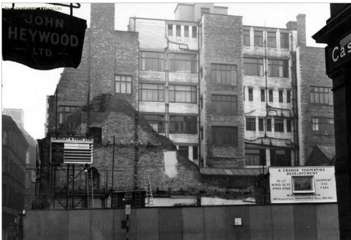
Figure 7: John Dalton Street, Building site in 1959. Source: Manchester Libraries.
