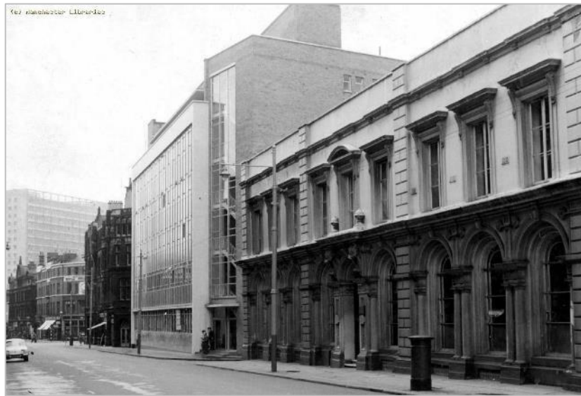
Figure 8: Newly erected Grange House, pictured 1961. Note the original ground floor. Source: Manchester Libraries.
