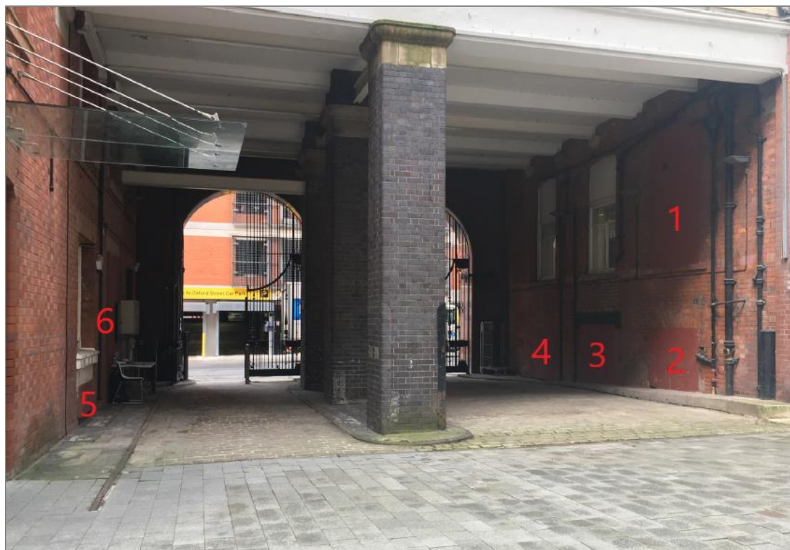
Figure 11: There are a number of modern coverings to the basement and first floor windows within the loading bay. These are numbered in the image above. These areas have previously been blocked up internally, forming solid plastered walls to the upper floors and breezeblock infill to the basement areas (now utilised as a car park.) Source: SLHA.
