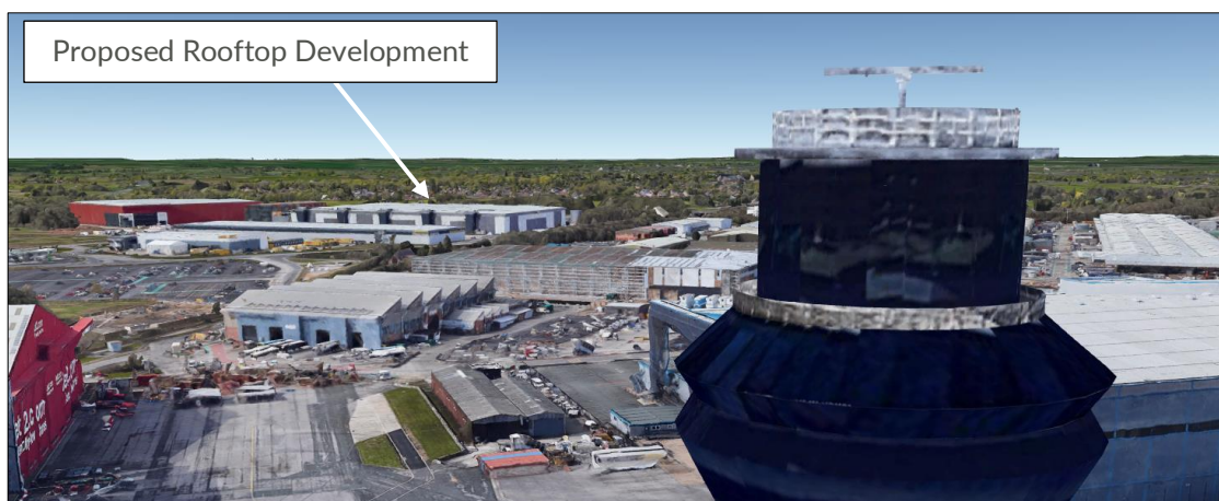
Figure 10 – View of the rooftop from the ATC Tower
