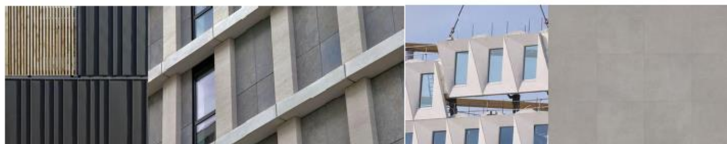
Materials - Zinc Cladding on the main surface exterior Stone Effect GRP Composite Extruded Window Fins
