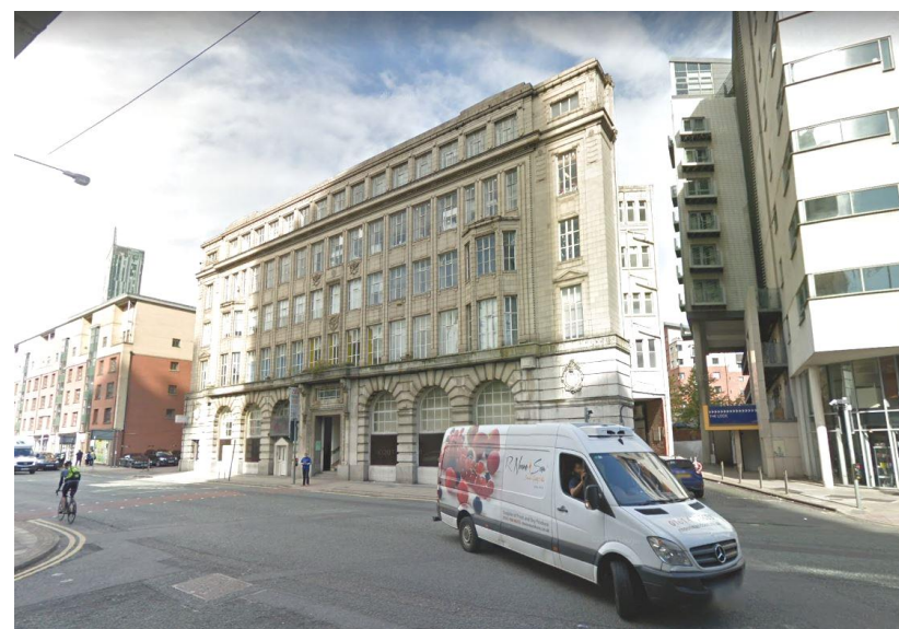
Whitworth Street view of Barclay House
