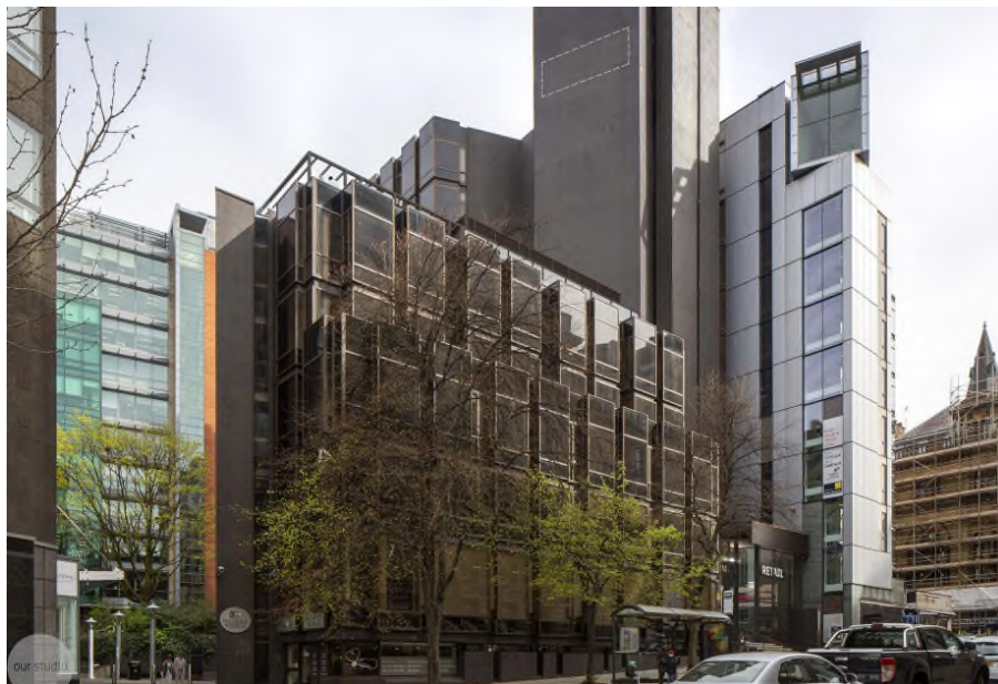
Figure 3.4: King Street roof-top extension (Source: Our Studio, 2022)
