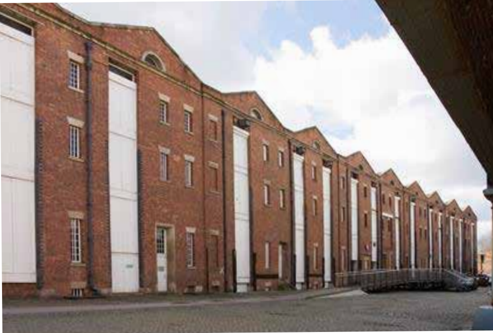
The North elevation
