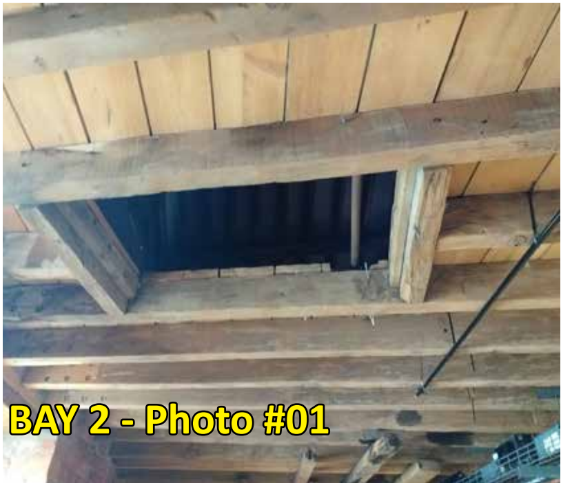
Photo #01 shows the existing opening in the mezzanine of Bay 2.
