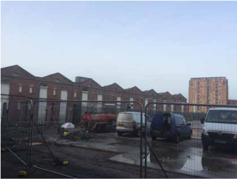
The north elevation from the Pinnapple Line viaduct
