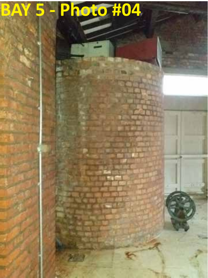
Photo #04 shows the elevational profile of the existing brick enclosure above the existing spiral stair.
