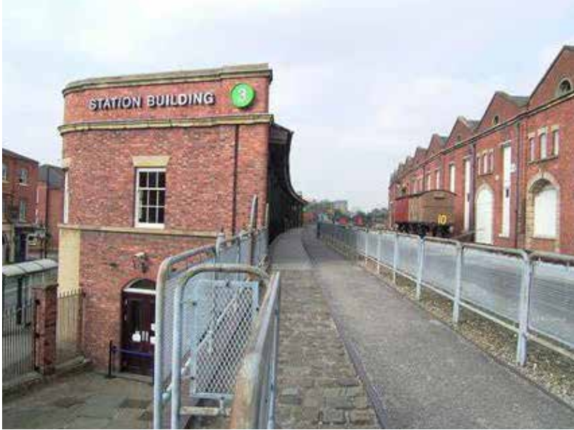
The south elevation looking west from the station platform
