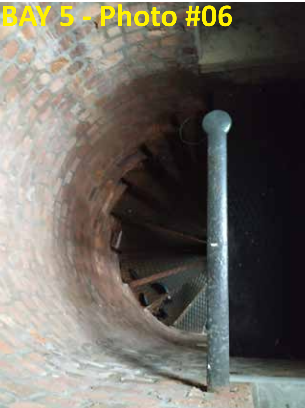
Photo #06 looks down from the existing lower platform on the second floor.
