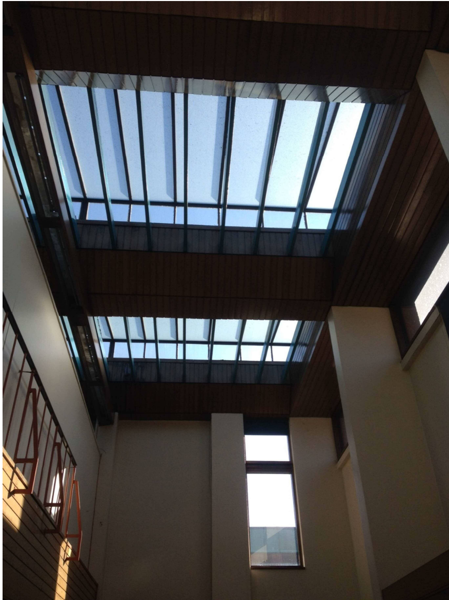
Photo 4. Internal view of roof-lights
