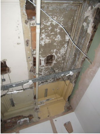
Image 20:- View of plaster ceiling to floor 2, Back Pool Chambers
