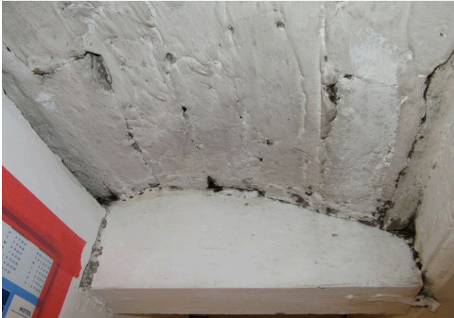
Image 13- Arched ceiling to basement
