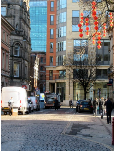
Image 31- Long view of Princes' Chambers as seen from outside St Ann's Church with metal roof structure just visible
