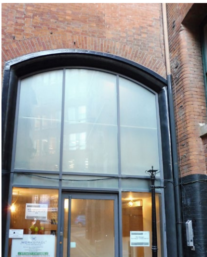
Image 29- View of original opening to loading bay with modern glass screen
