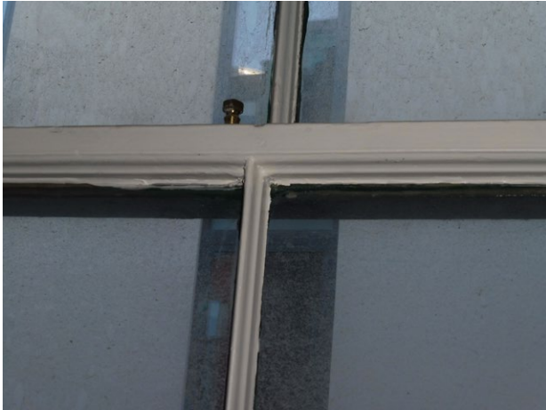
Image 26- Typical detail of finer timber sash frames
