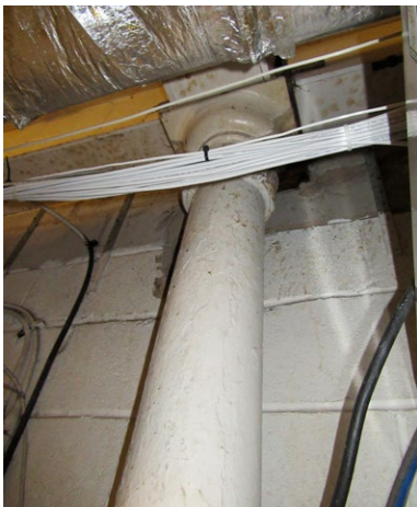
Image 14- Cast iron columns present in Sam's Chop House beer store
