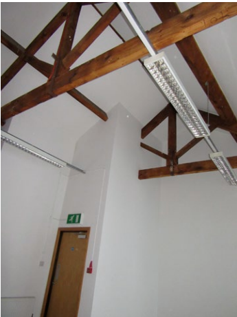
Image 21:- View of exposed timber roof structure in Back Pool Chambers, floor 3
