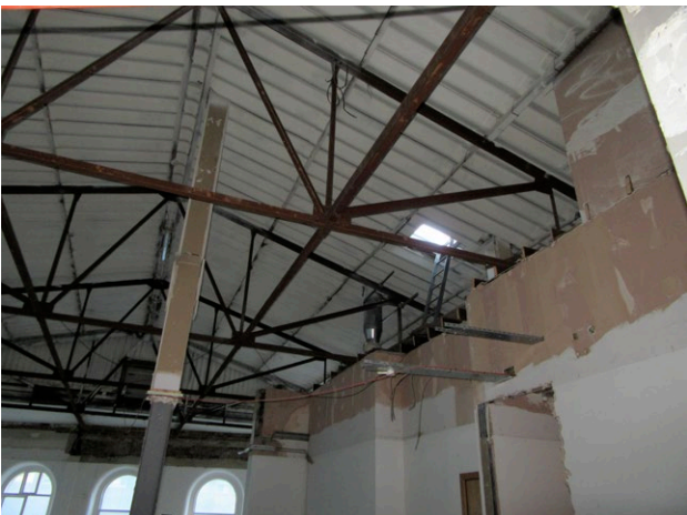
Image 22- View of later addition metal roof to floor 3, Princes' Chambers
