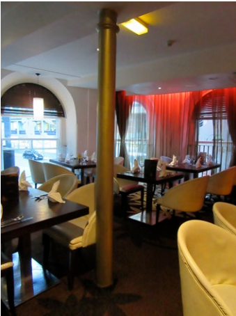
Image 17:- Cast iron columns within existing restaurant space
