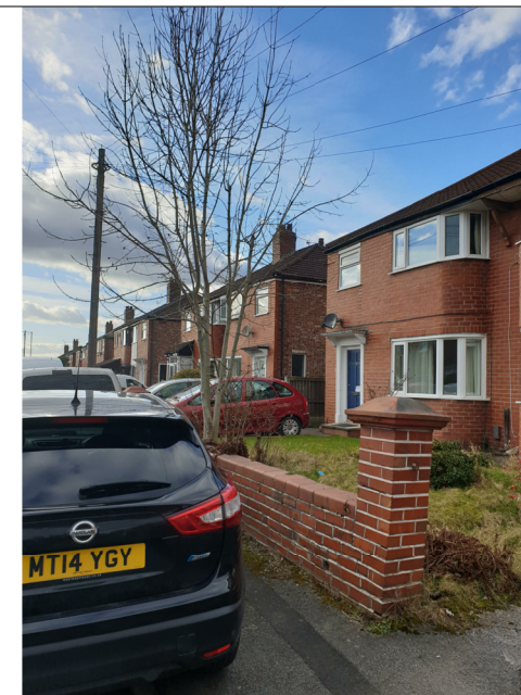
Opening to be made wider by removing external wall
