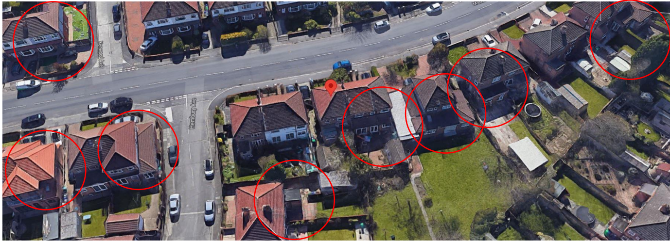
Several examples of immediate neighbours with single and two storey side and rear extensions.
