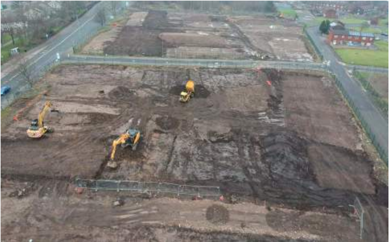
Figure 60 : Stockpile maintenance and final excavation to design levels underway adjacent to Paget Street
