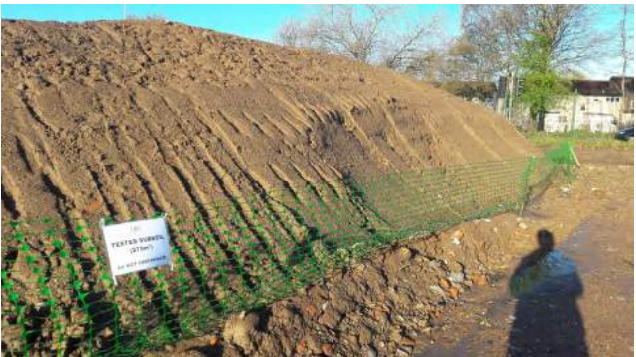
Figure 57 : Southern stockpile of tested subsoil (270m 3 )
