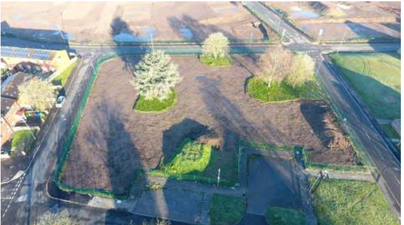
Figure 67 : Works completed in the Park area, root protection fencing removed, topsoil stockpile adjacent to parking area, security bund across access gateway
