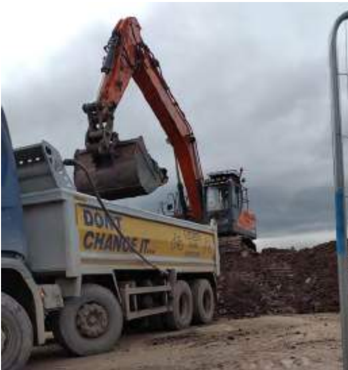
Figure 28 : Loading of surplus fill material for disposal off site
