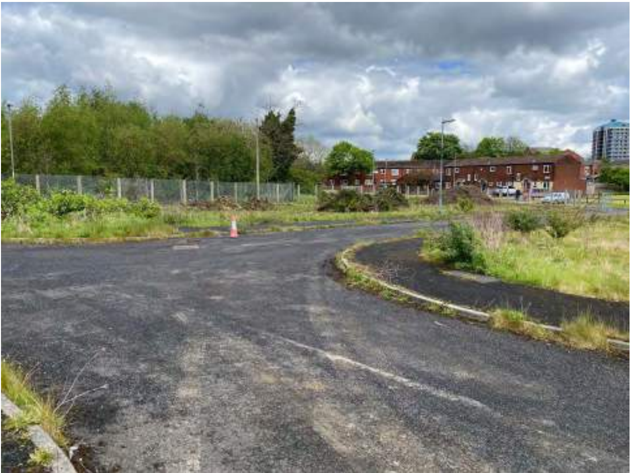
Figure 1 : Initial vegetation clearance adjacent to Needwood Close at commencement of site works
