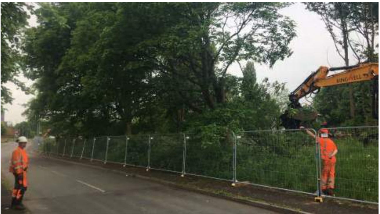
Figure 2 : Tree surgeons at work along the Thornton Street North boundary of the site
