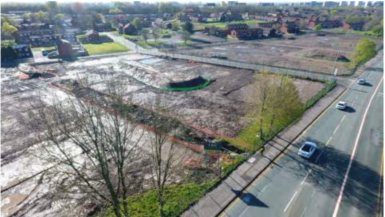
Figure 68 : Looking southeast across the completed site, with remaining fibre-optic easement fenced in orange, and tested subsoil stockpiles fenced in green. Fibre-optic cable was removed in April 2022; LKR remobilised to site and completed remediation of the easement corridor
