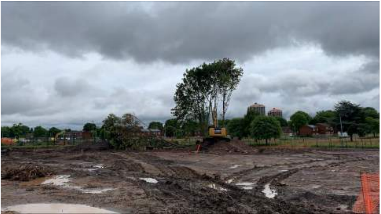
Figure 3 : Tree removal operations well progressed
