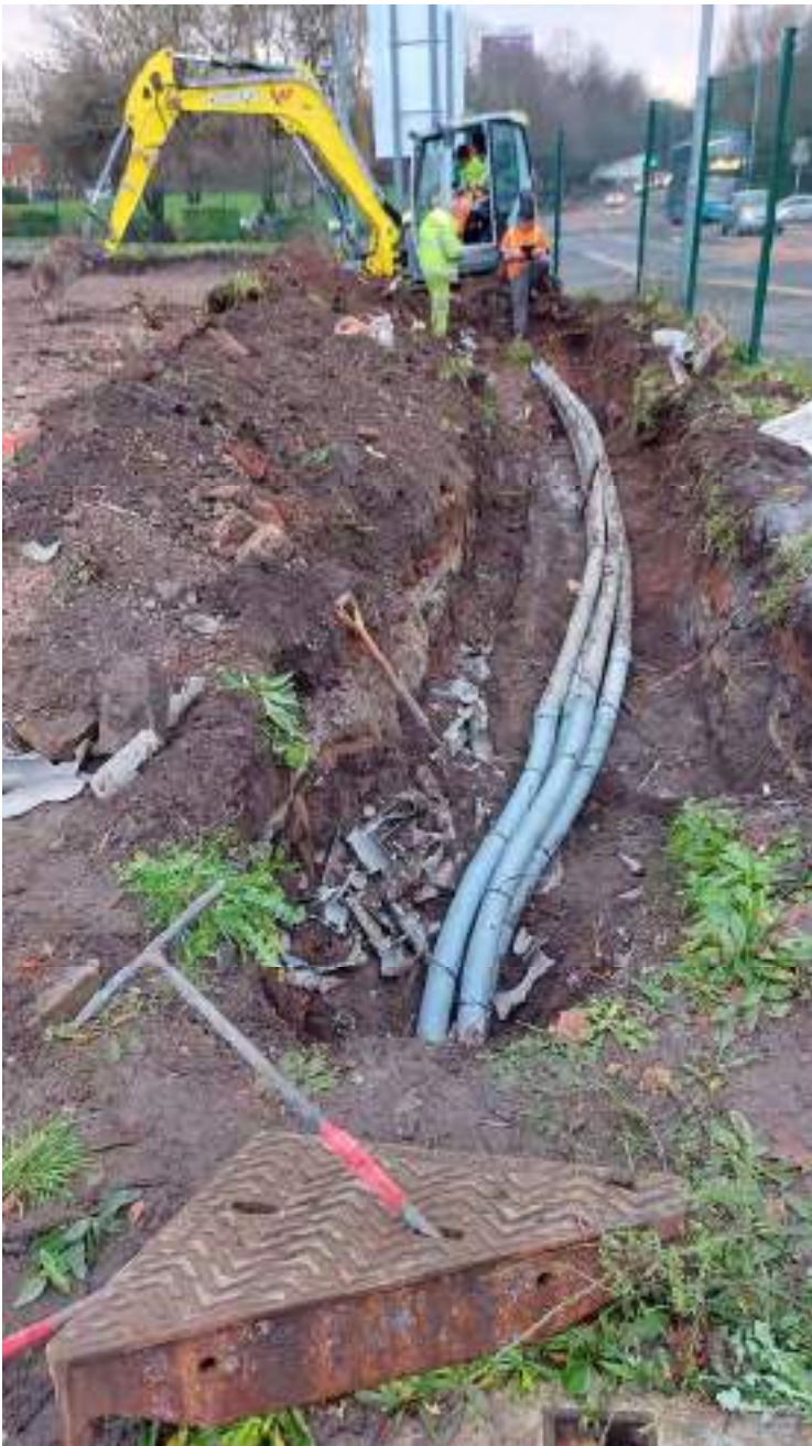
Figure 40 : Diversion of four BT Openreach ducts adjacent to Rochdale Road
