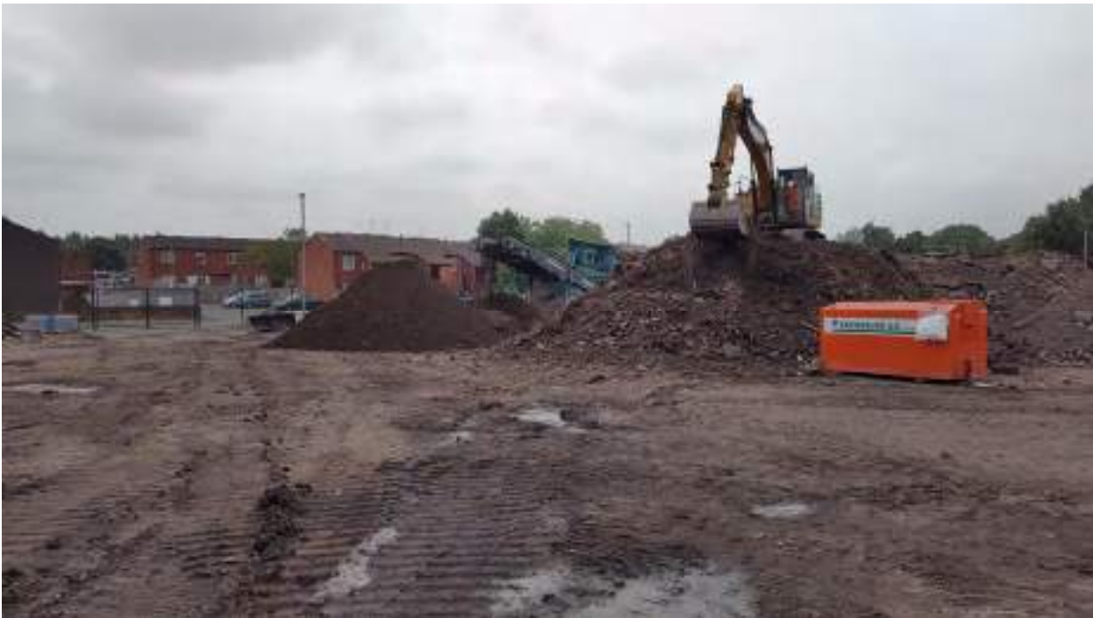
Figure 23 : Screener being used to process excavated material prior to use as backfill
