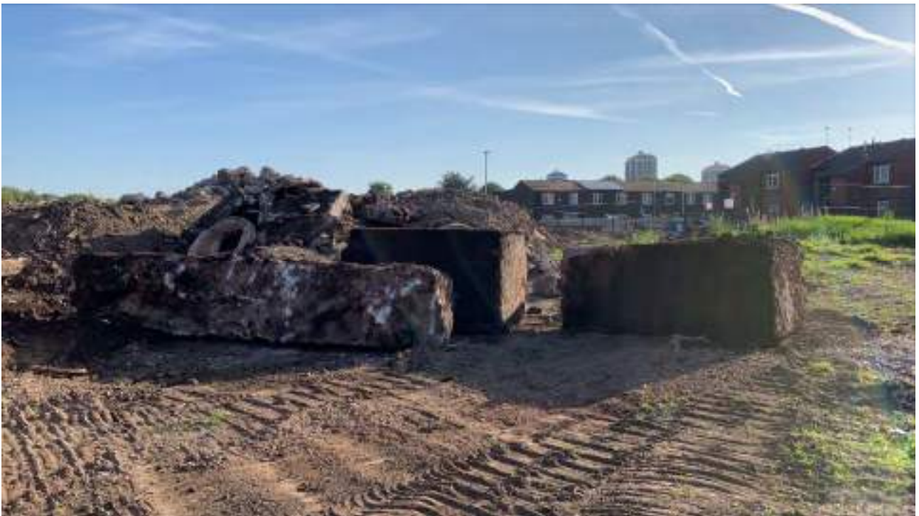
Figure 19 : Large foundation blocks awaiting reduction in size prior to crushing
