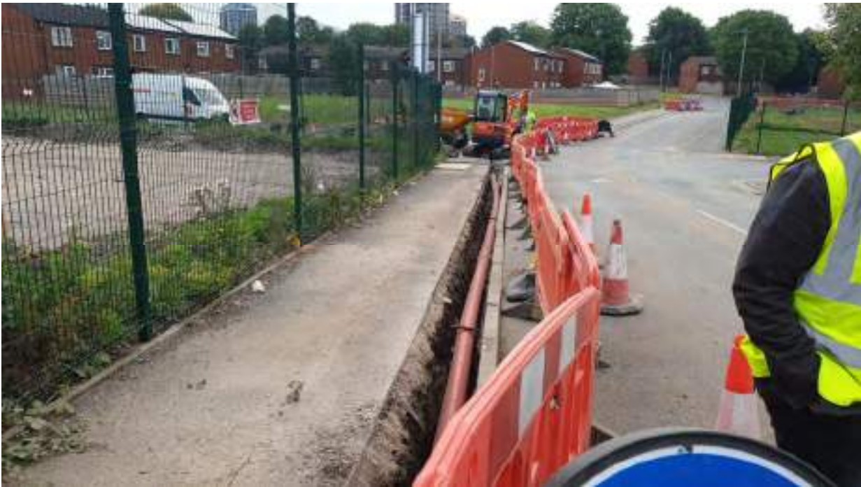
Figure 46 : Installed electricity duct within north footway of Paget Street (looking towards Burgess Street)
