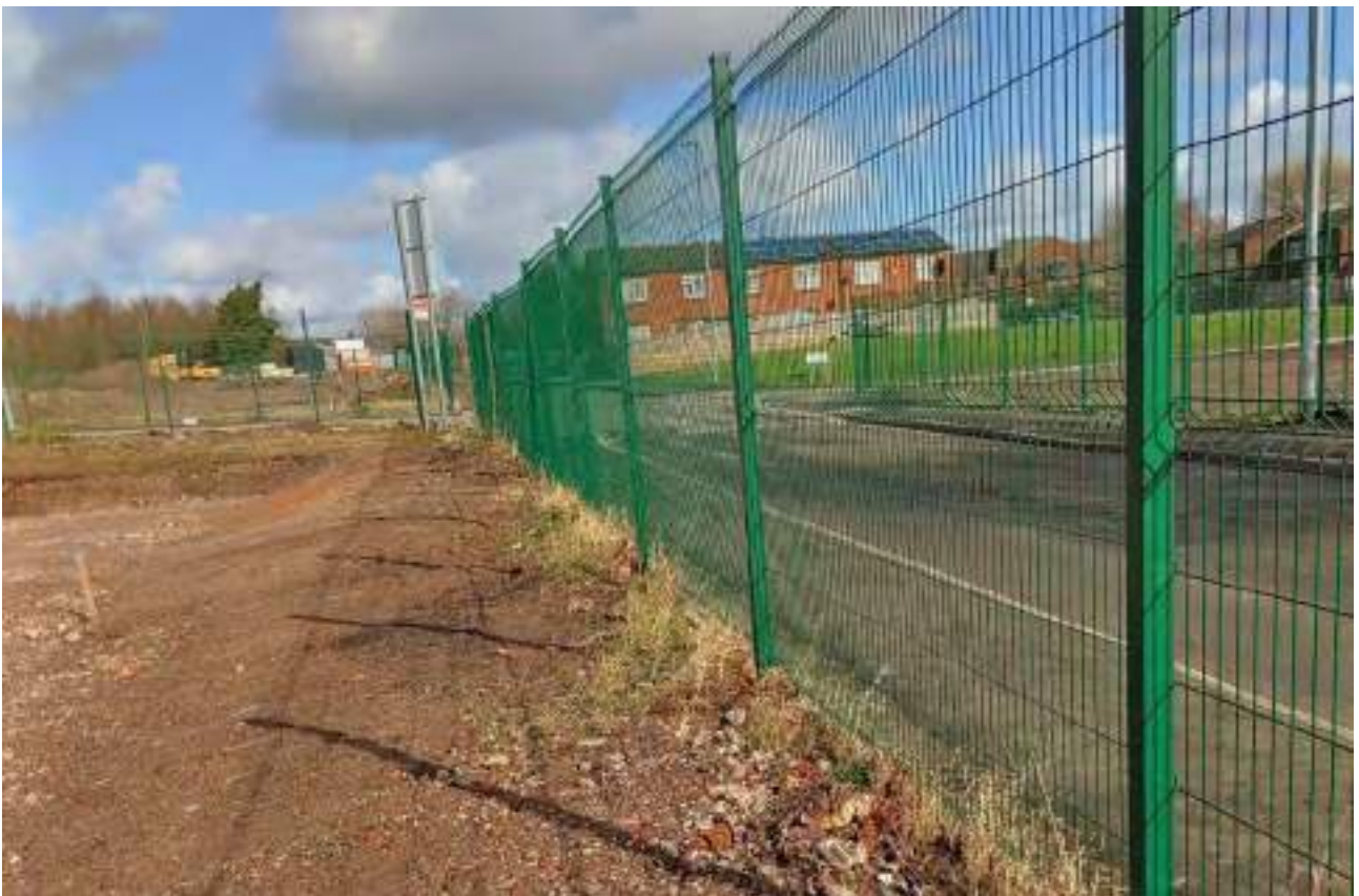
Figure 65 : Security fencing installed along Thornston Street North, with graded batter to adjacent pile mat
