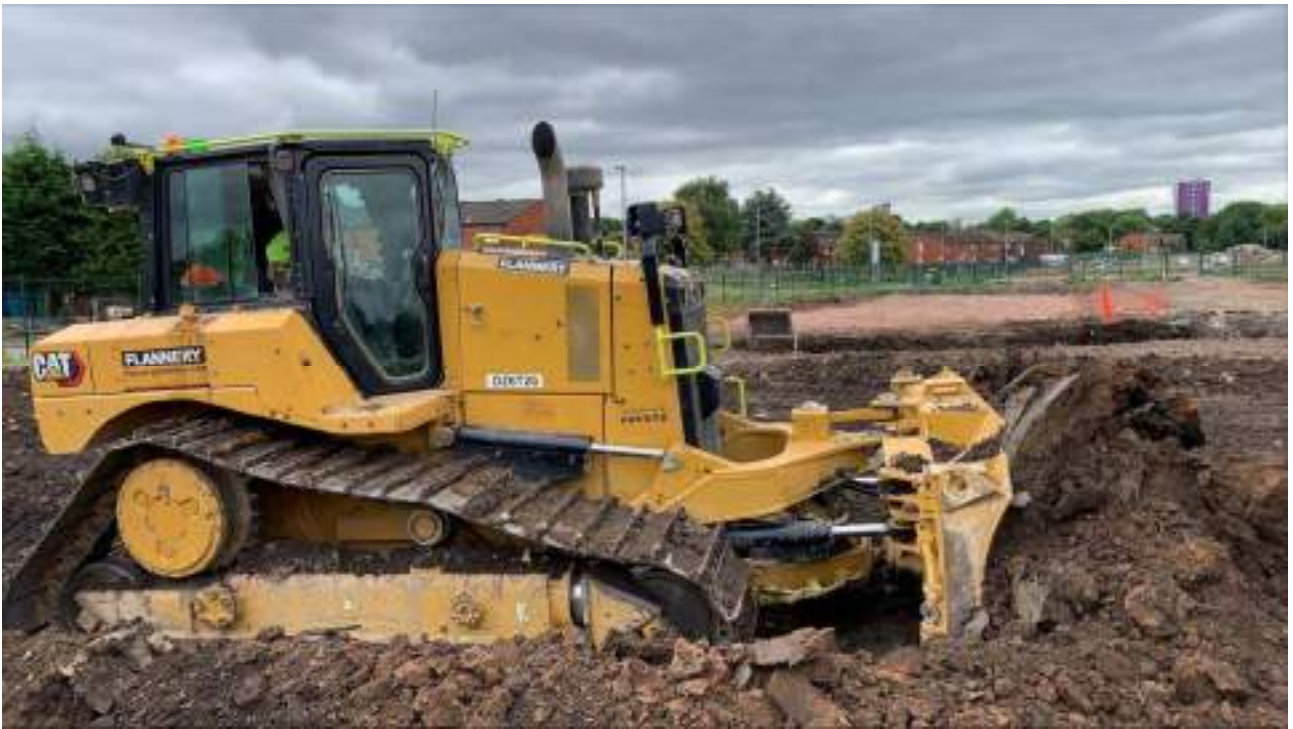
Figure 35 : Dozer in action to cut to design levels in north of site
