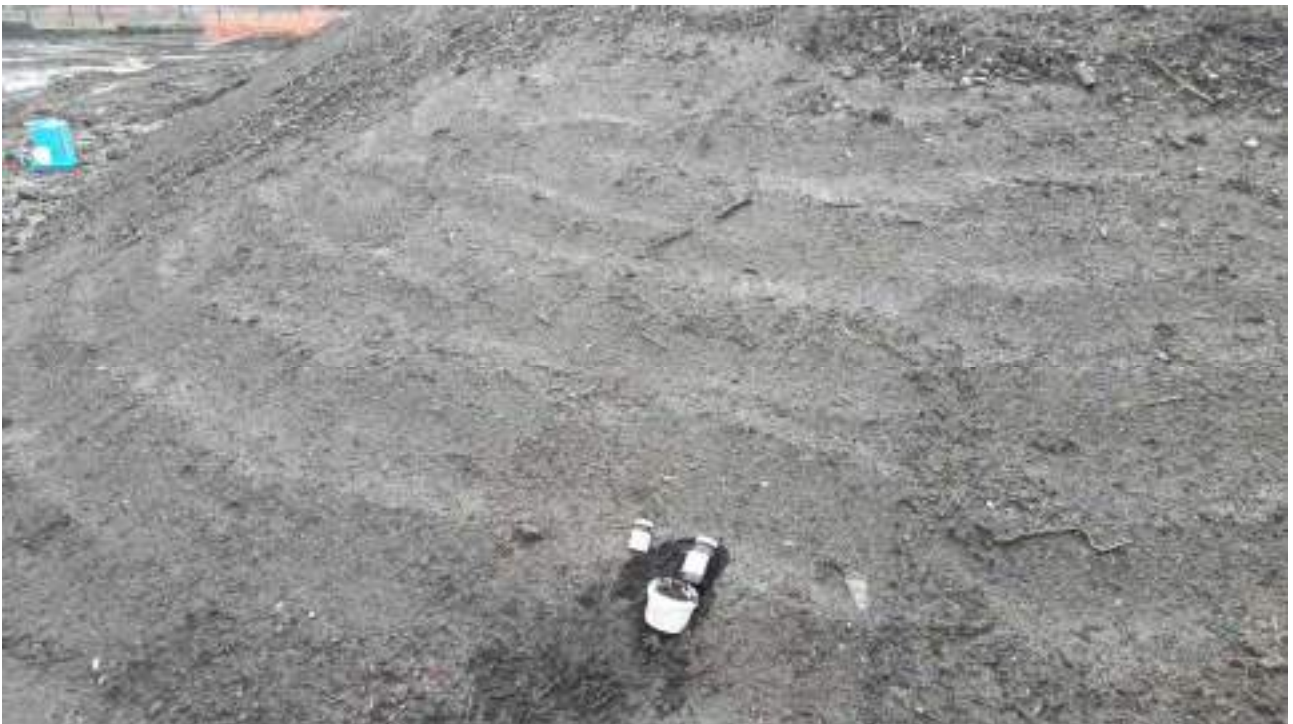
Figure 51 : Sampling of stockpiled topsoil for laboratory analysis
