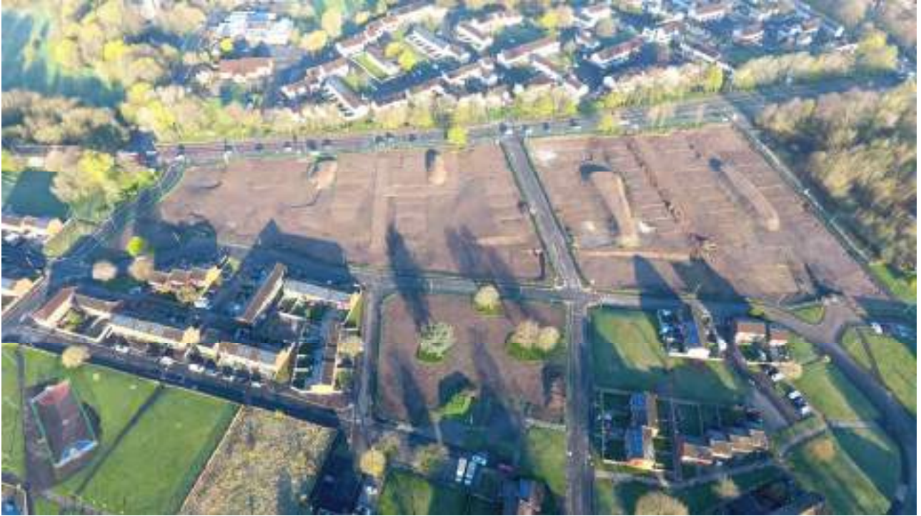
Figure 70 : Completed site seen from east looking towards Rochdale Road
