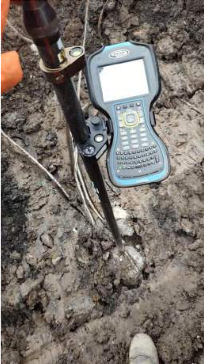
Figure 16 : Concrete pile cropped to specified level and surveyed prior to placement of re-engineered fill
