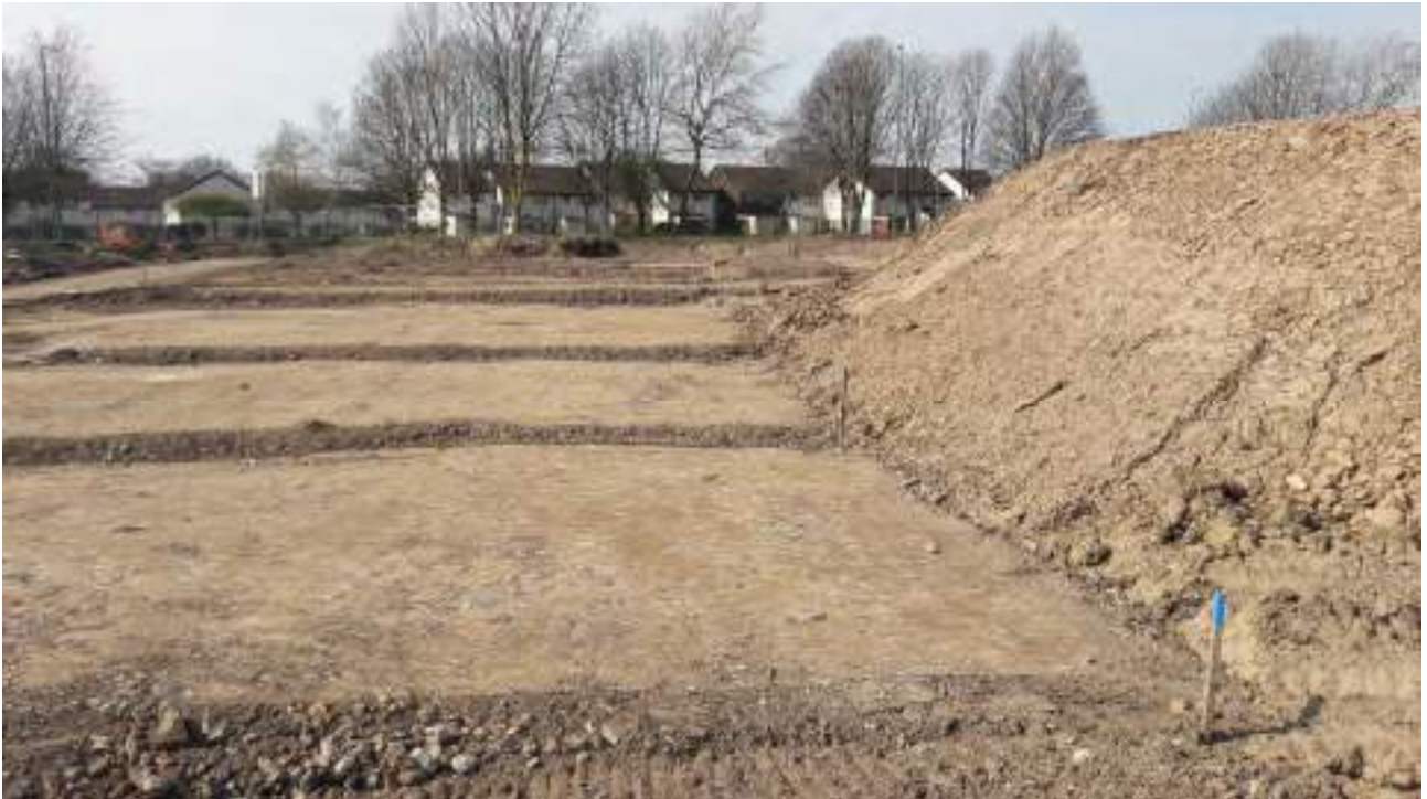
Figure 62 : Completed pile mat to plots seen under construction in Figure 61 (above); stockpile of tested subsoil to right of frame
