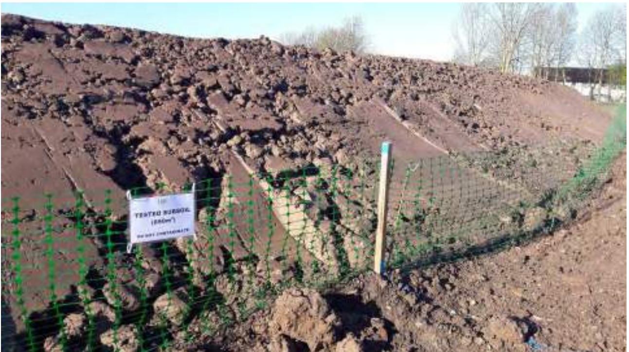
Figure 59 : Northern stockpile of tested subsoil (850m 3 )
