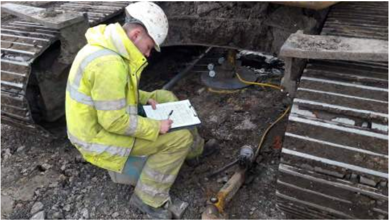
Figure 52 : CBR testing underway using 25T excavator as kentledge
