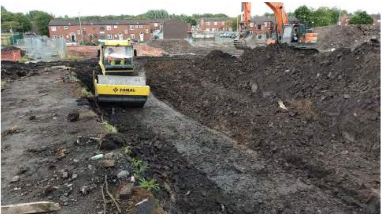
Figure 38 : Compaction of suitable fill adjacent to Churnet Street existing sewer easement
