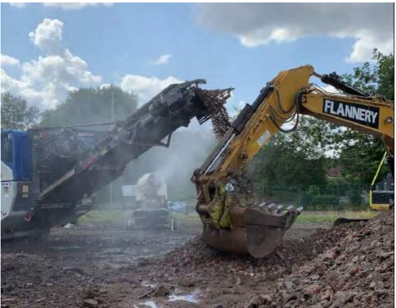
Figure 22 : Crusher in action with misting spray unit deployed to mitigate any potential dust emissions
