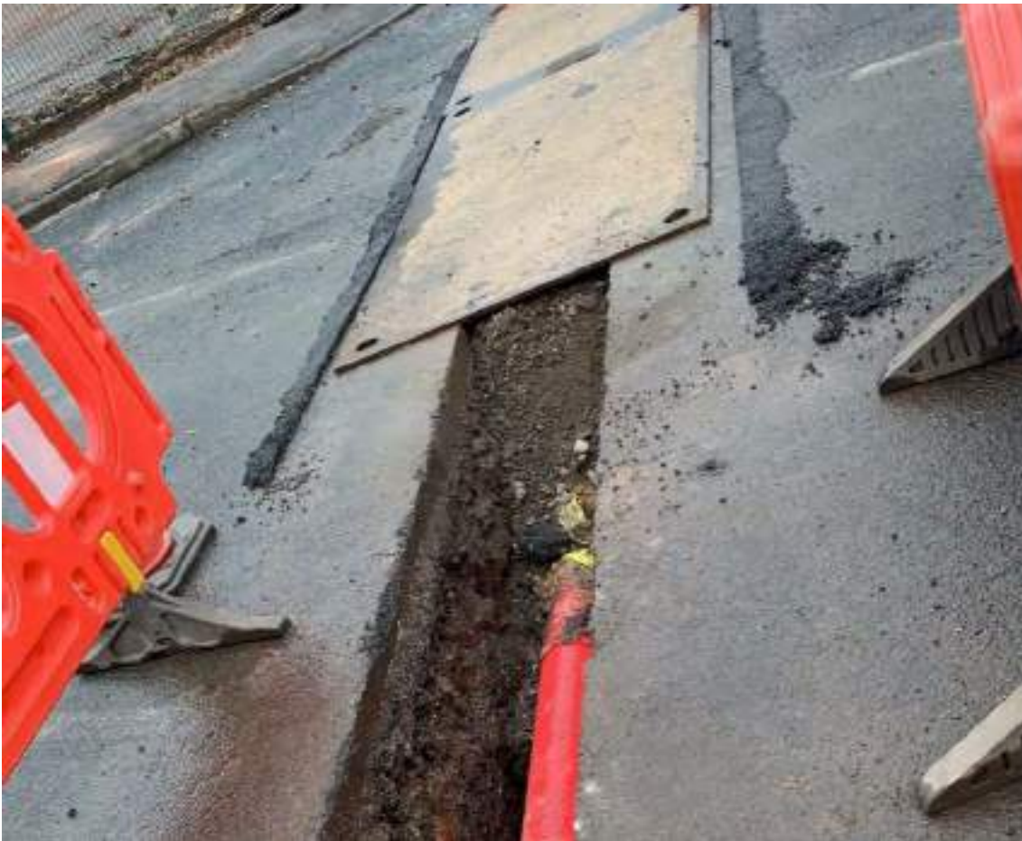
Figure 48 : Diversion of electricity cable across Thornton Street North
