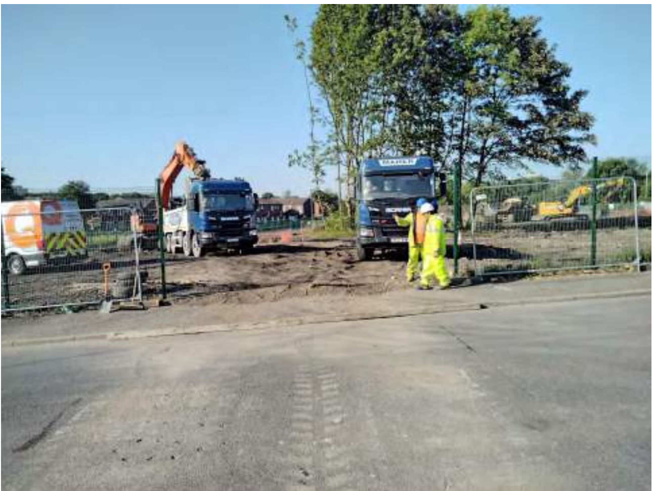
Figure 12 : Loading and export of knotweed-contaminated soils under supervision
