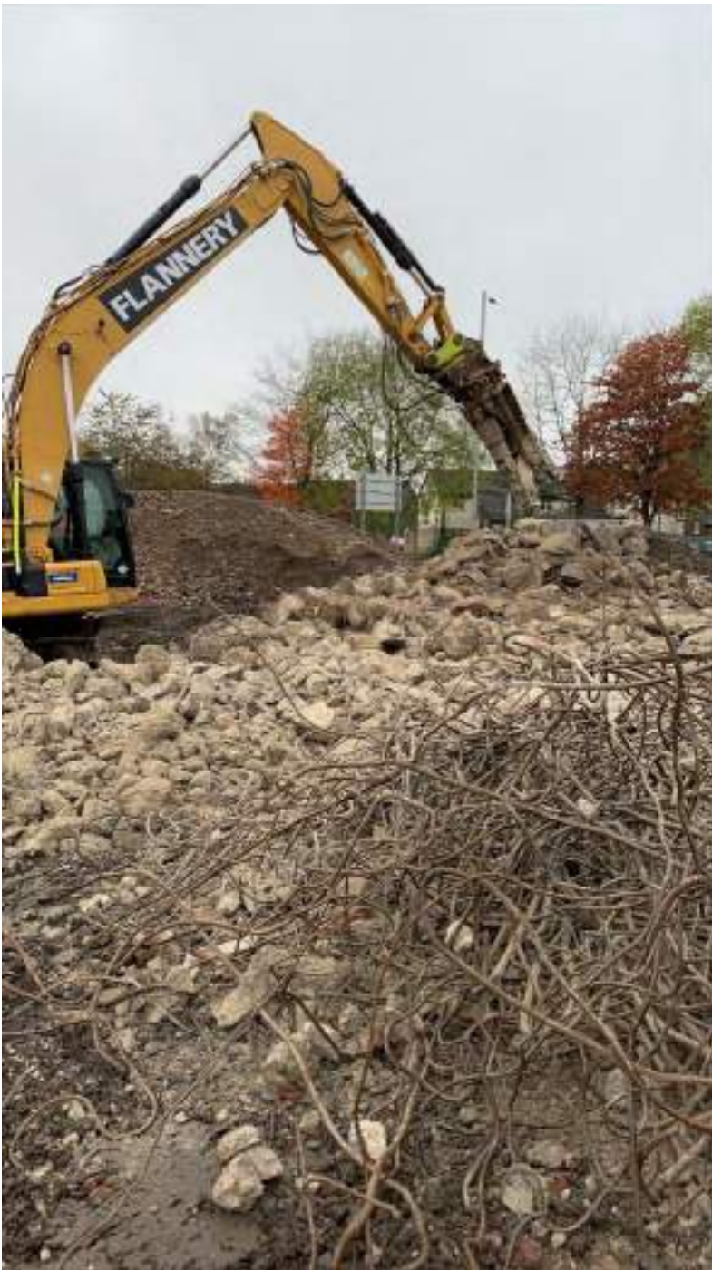
Figure 20 : Excavator using a hydraulic muncher to process oversize and stockpile the recovered reinforcement wire
