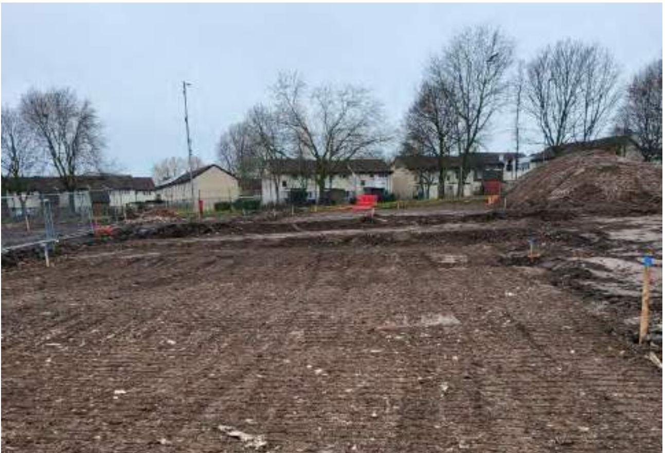
Figure 63 : Completed pile mats adjacent to Paget Street, looking towards Rochdale Road
