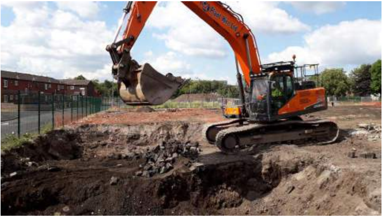
Figure 11 : Excavator working from outside the knotweed quarantine boundary to sift the soils and remove remaining rhizomes
