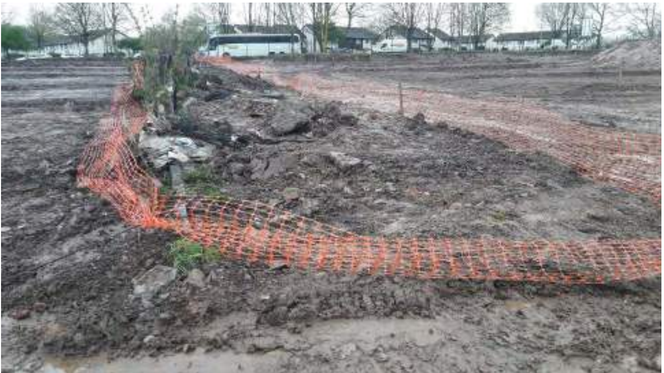
Figure 55 : Easement for BT Openreach fibre-optic fenced off during remediation works to avoid damage. The fibre-optic cable was finally removed in April 2022, after which LKR remobilised to site and completed remediation of the easement corridor
