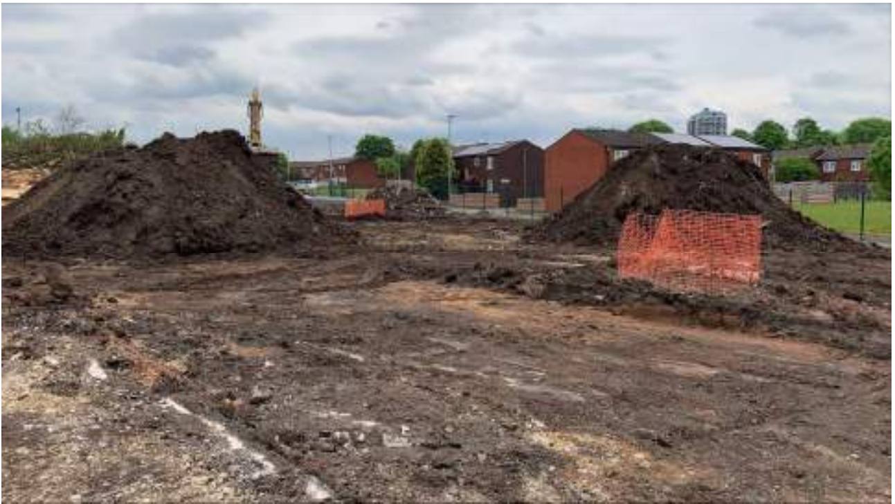
Figure 25 : Segregated stockpiles of excavated materials, with fenced-off drainage manholes (to be retained)
