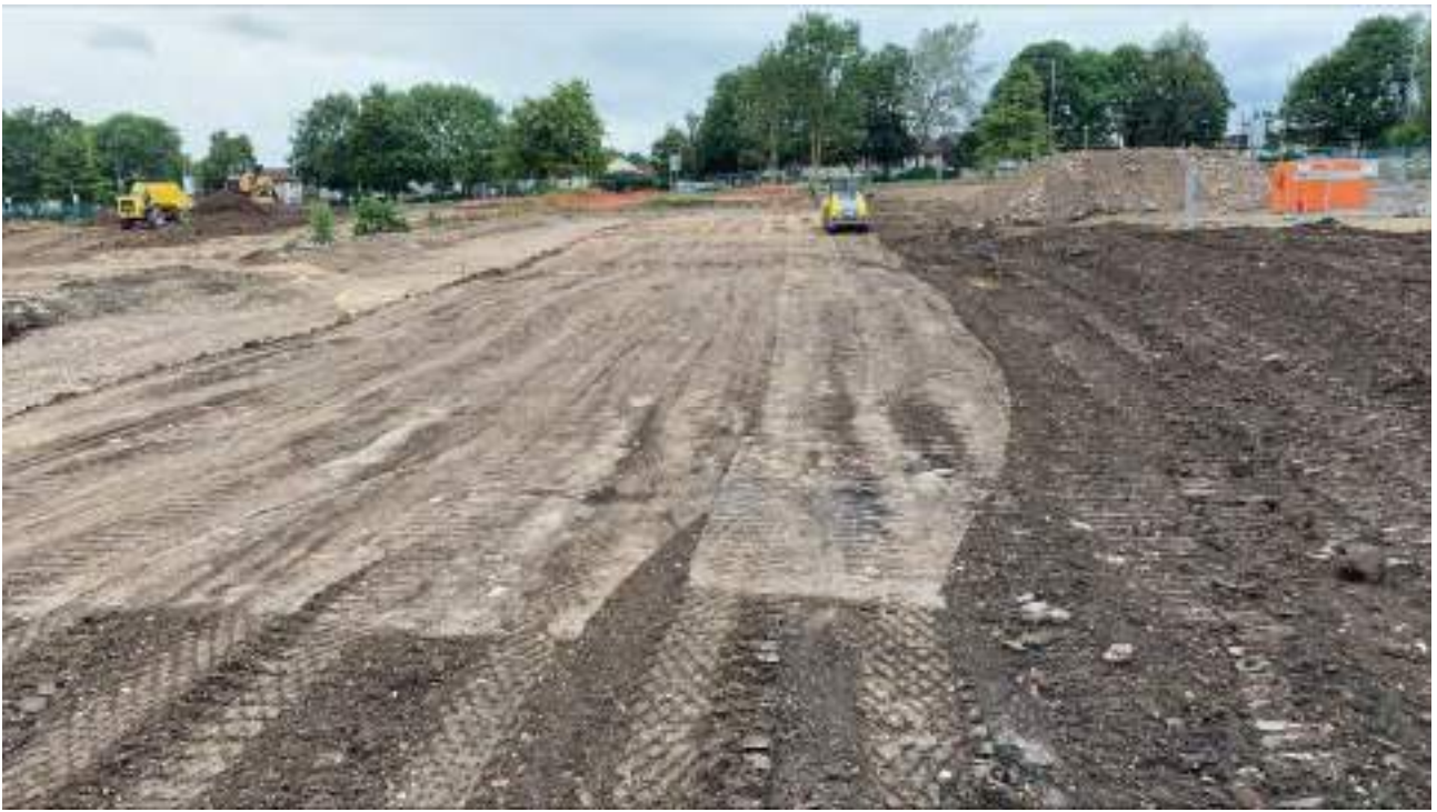
Figure 39 : Compaction of suitable fill in accordance with the specification
