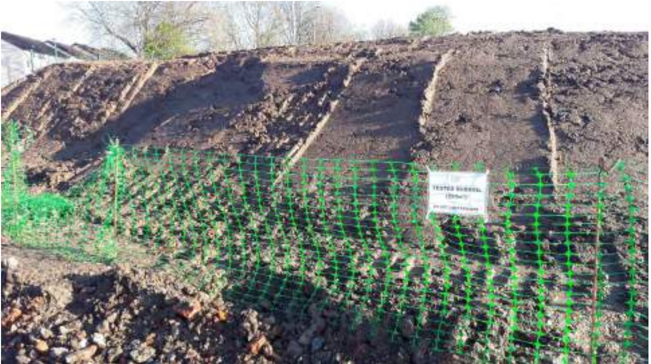
Figure 56 : Southern stockpile of tested subsoil (250m 3 )
