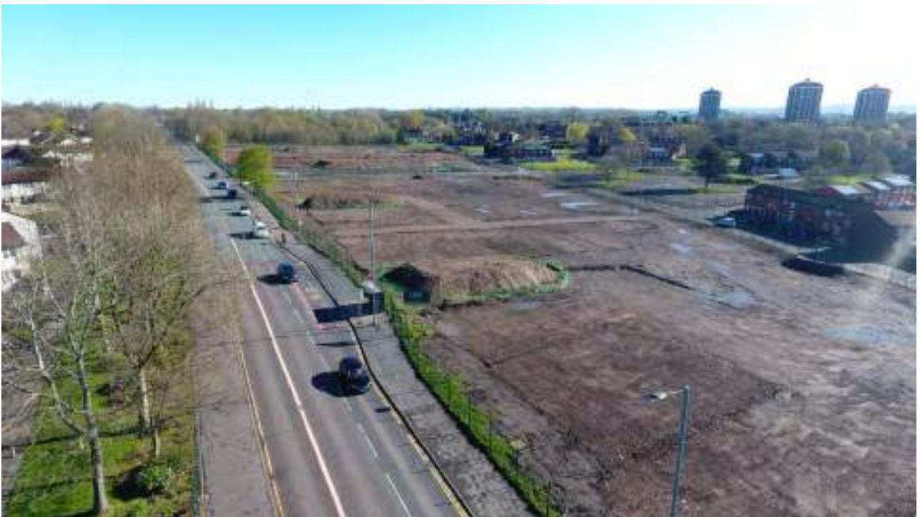
Figure 69 : Looking north from Rochdale Road across completed site, with remaining fibre-optic easement fenced in orange, and tested subsoil stockpiles fenced in green. Fibre-optic cable was removed in April 2022; LKR remobilised to site and completed remediation of the easement corridor
