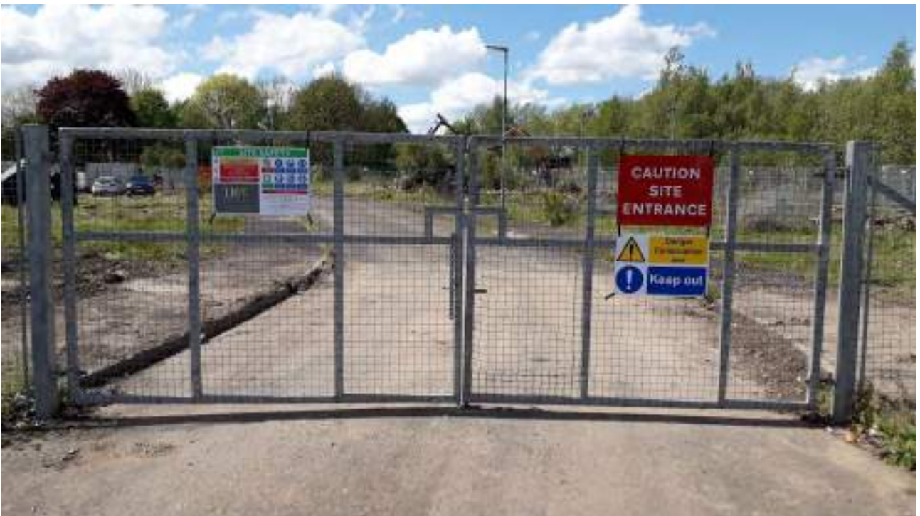
Figure 8 : Site entrance retained existing gates until new perimeter fencing had been installed
