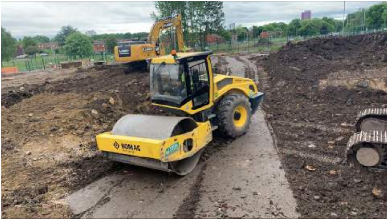
Figure 37 : Compaction of suitable fill material in accordance with the specification
