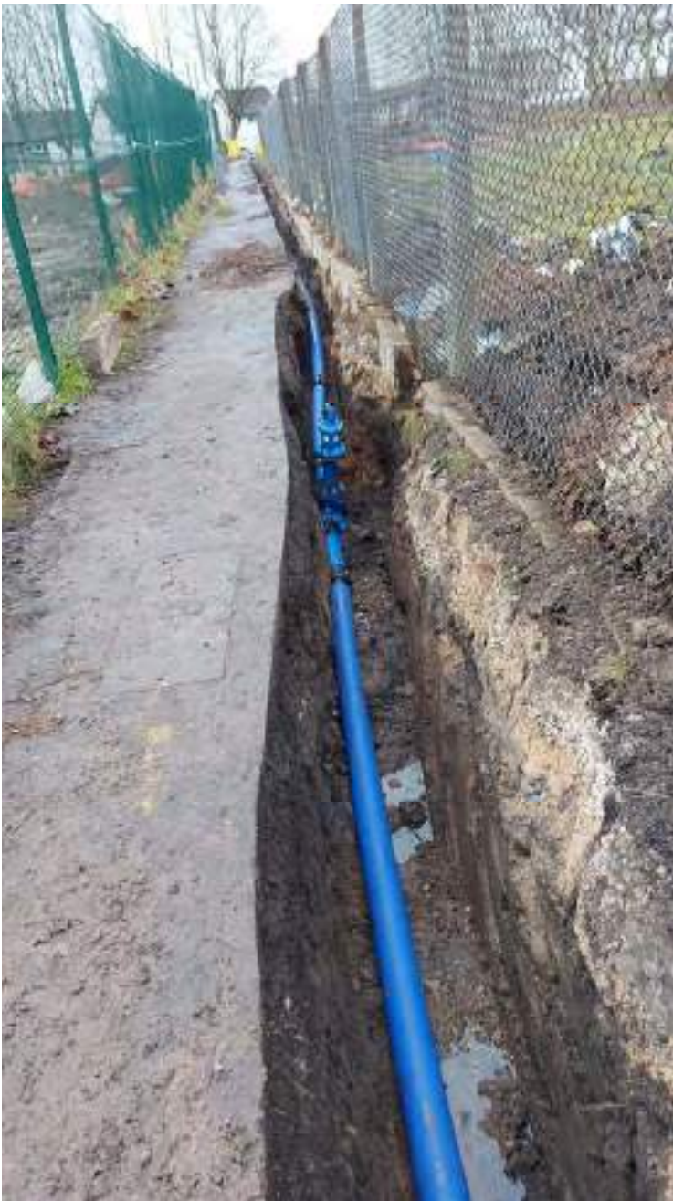
Figure 45 : Installation of water main diversion within Marston Street footpath at north of site
