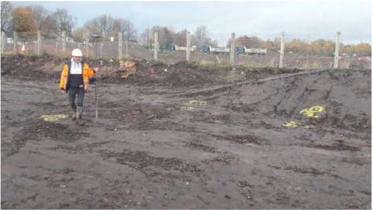
Figure 31 : GPS control of earthworks operations
