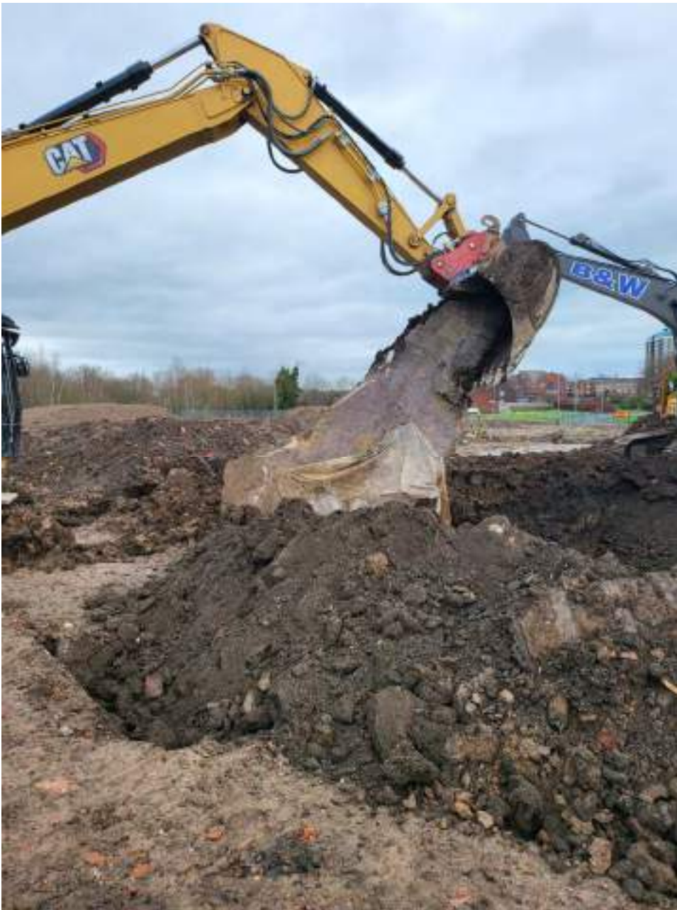
Figure 17 : Relic slab being removed by excavator
