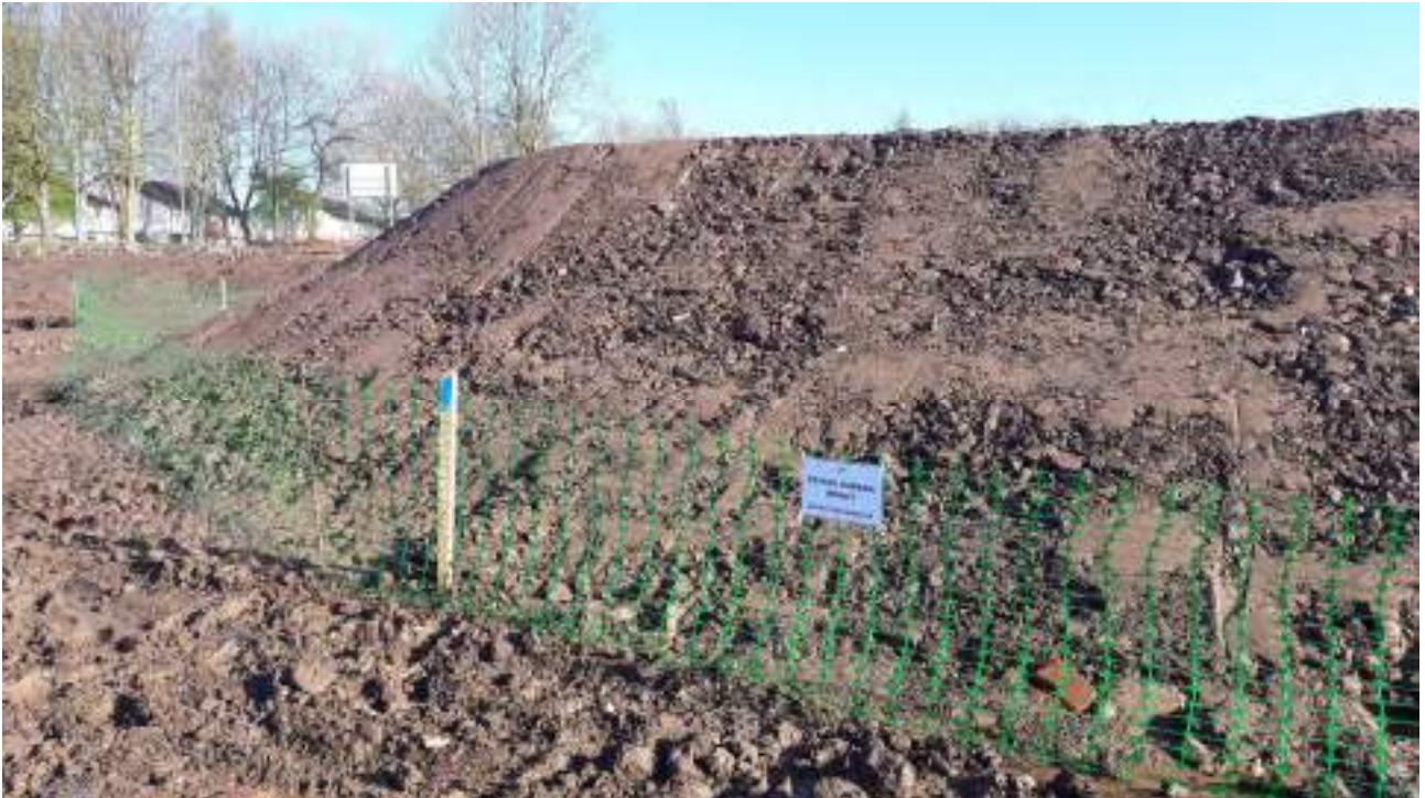
Figure 58 : Northern stockpile of tested subsoil (900m 3 )
