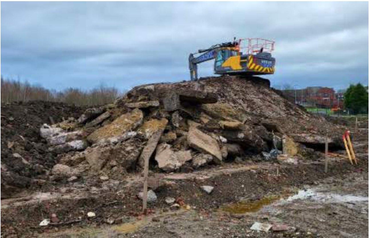
Figure 18 : Blocks of relic foundations and slabs awaiting processing, segregated from adjacent stockpiles of suitable fill
