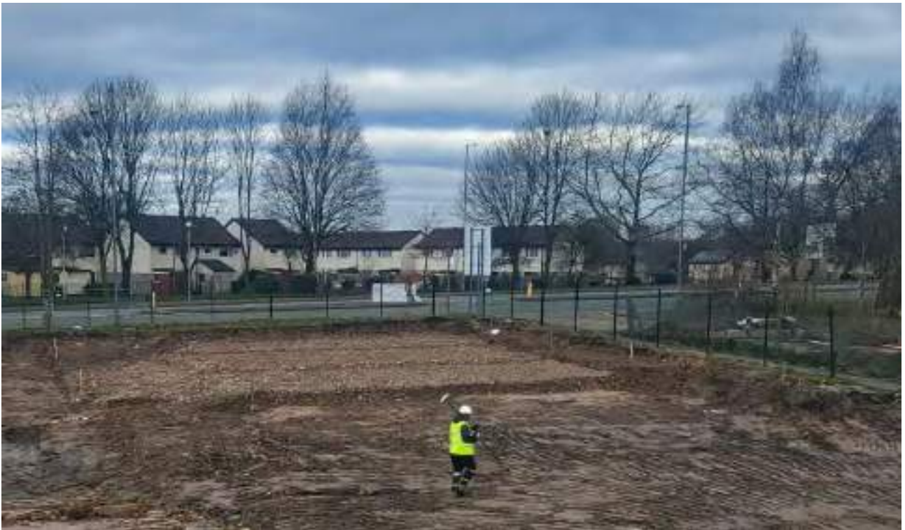
Figure 64 : Completed pile mats in the north-west corner of the site, adjacent to Marston Street footpath
