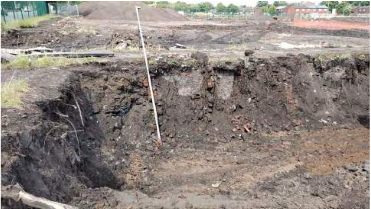
Figure 54 : Depth to natural being recorded with surveyor's staff as turnover works proceed
