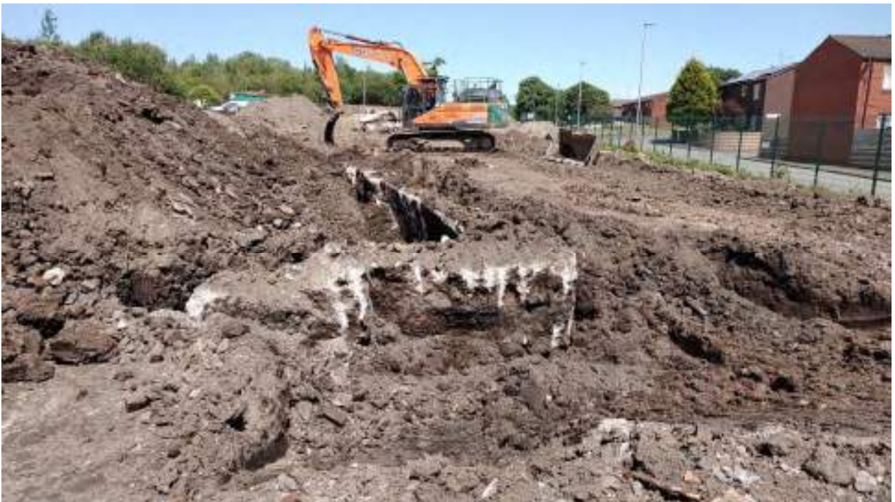
Figure 14 : Relic foundations being exposed prior to removal
