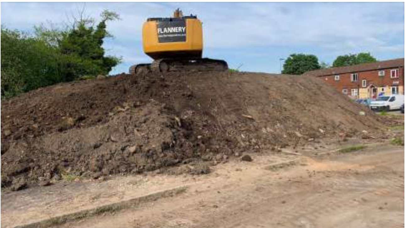
Figure 26 : Stockpile of mixed soils and roots awaiting disposal off site (Needwood Close entrance)
