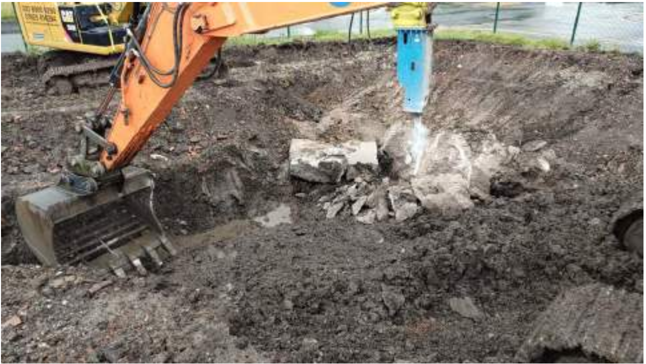
Figure 21 : Hydraulic breaker in use to assist in the removal of a large buried mass concrete foundation
