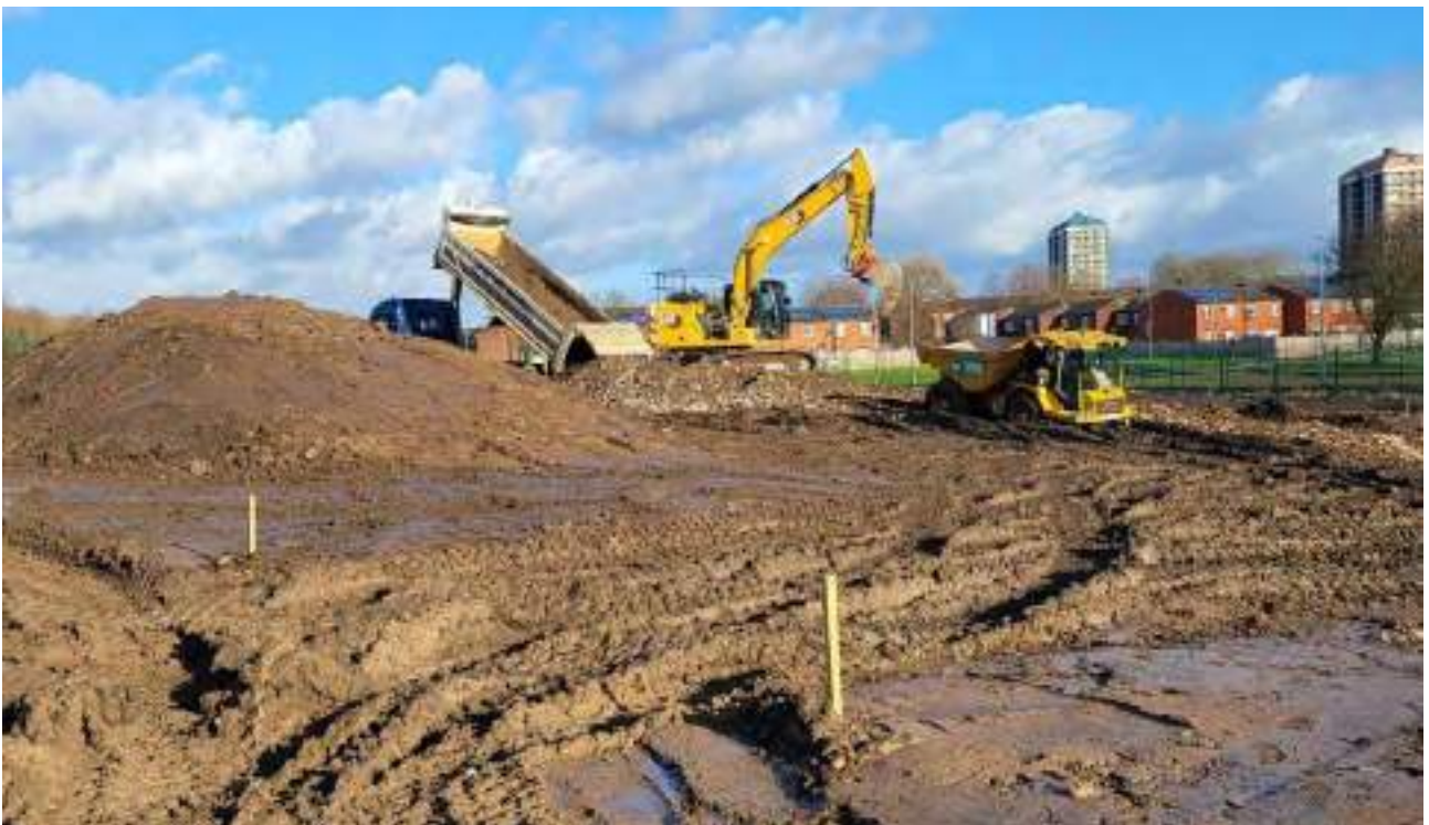
Figure 34 : Handling of imported crush for pile mat construction
