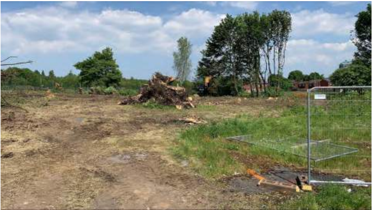
Figure 7 : Root mass stockpile awaiting collection and disposal as green waste
