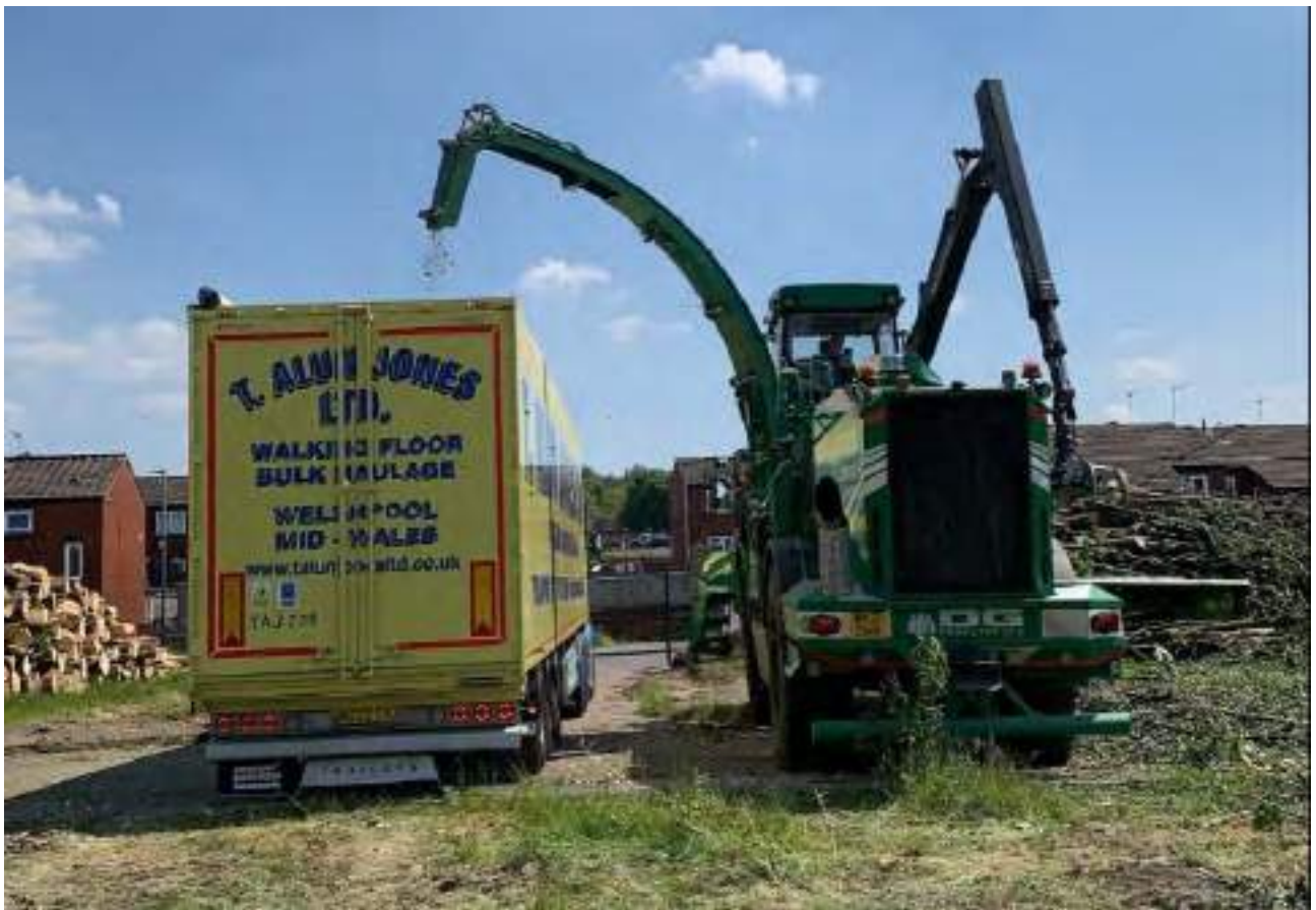
Figure 5 : Chipper unit processing felled timber into biomass
