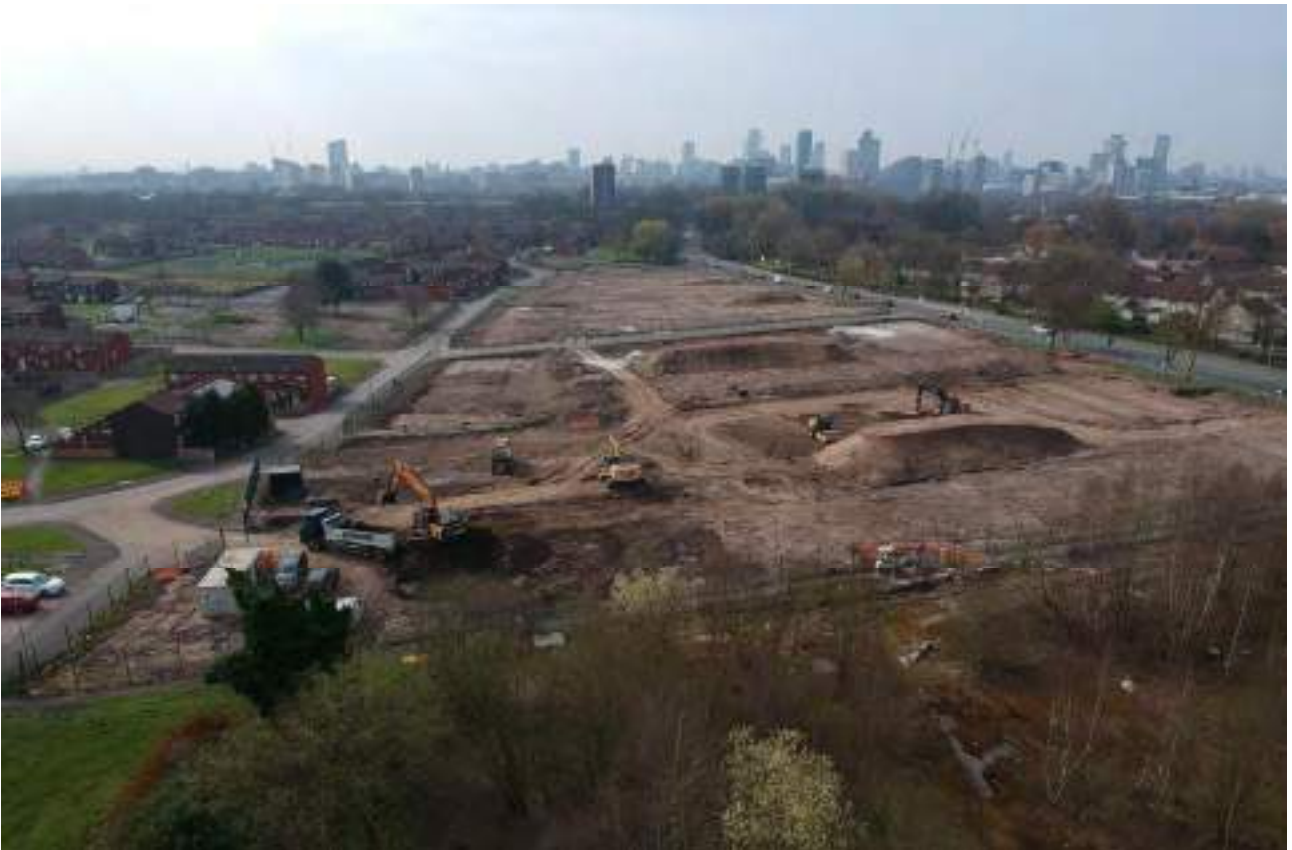
Figure 29 : Aerial view looking south: surplus soils being loaded for disposal, imported crush being placed to pile mats
