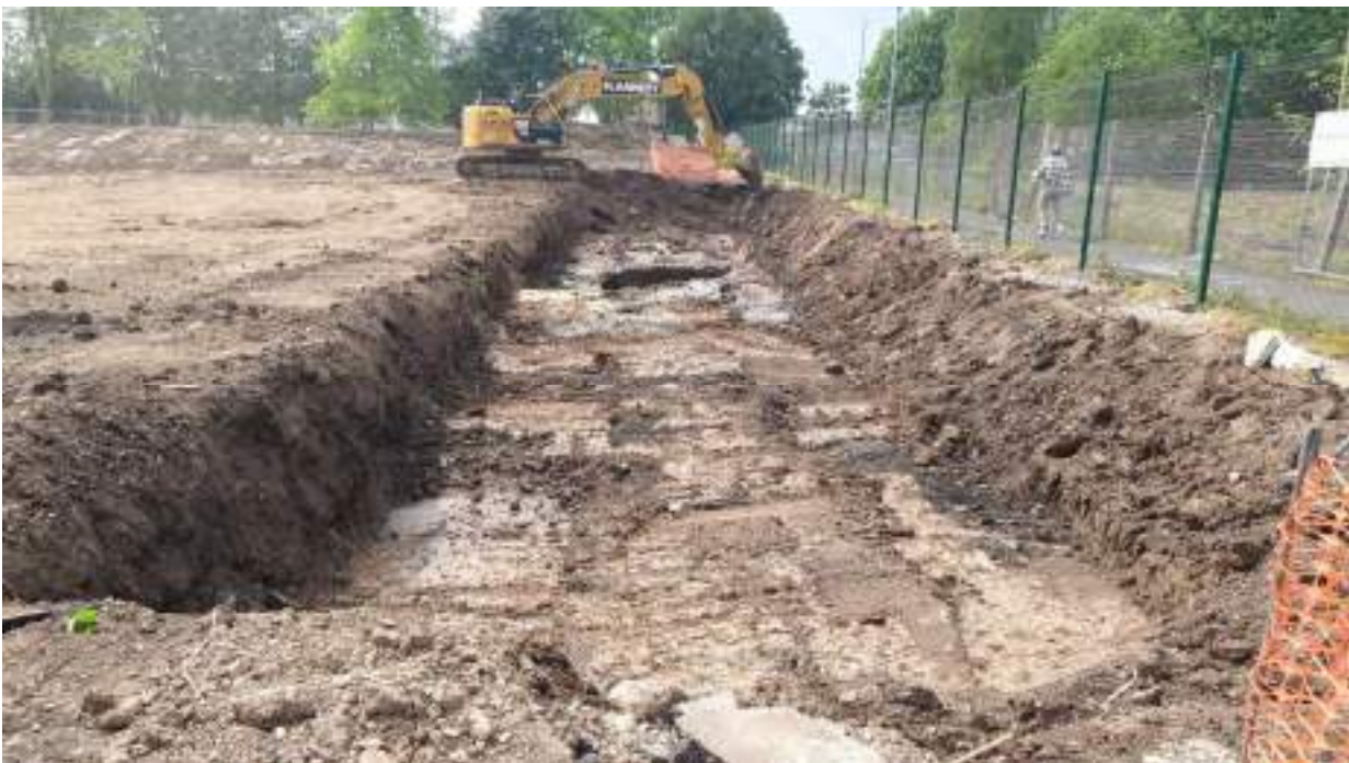
Figure 32 : Excavation to natural ground along the Marston Street boundary (north)
