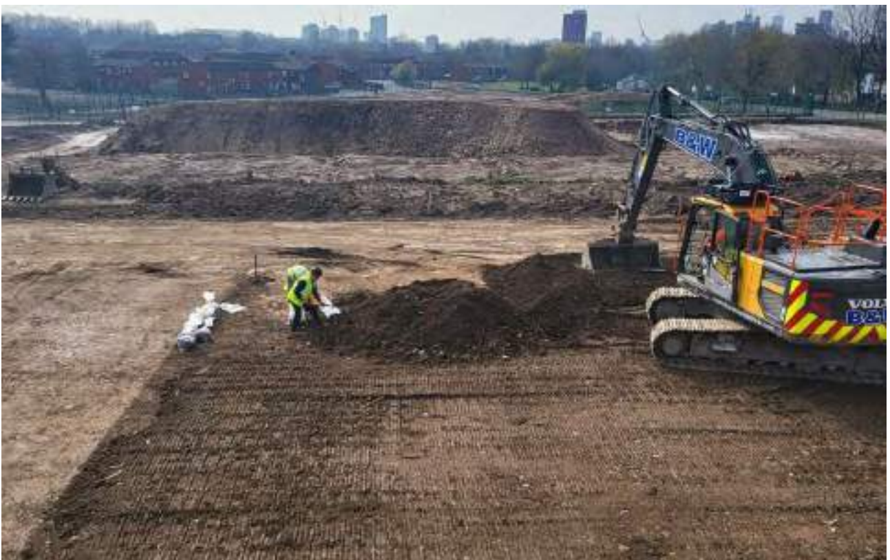
Figure 49 : Sampling of imported crush for geotechnical assessment
