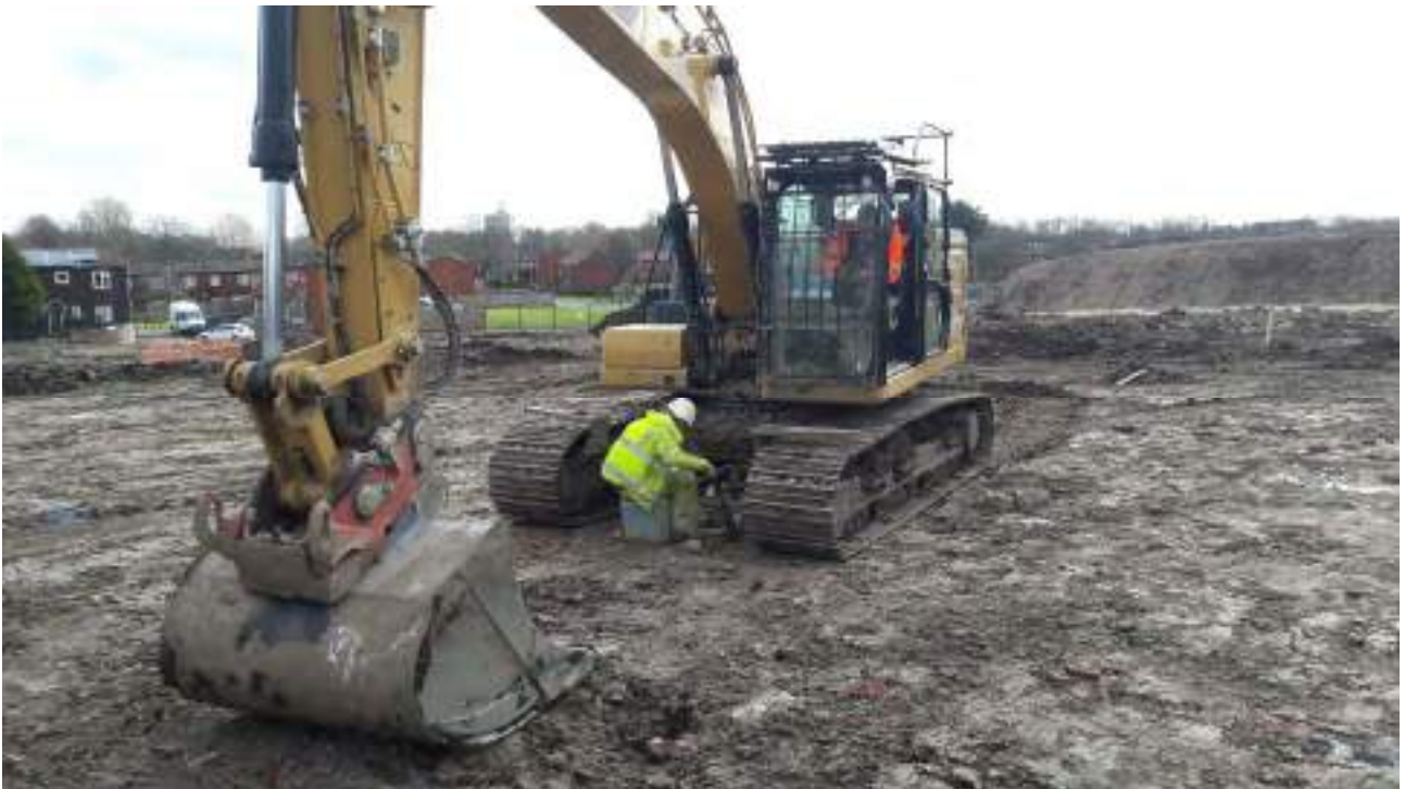
Figure 53 : CBR testing in progress
