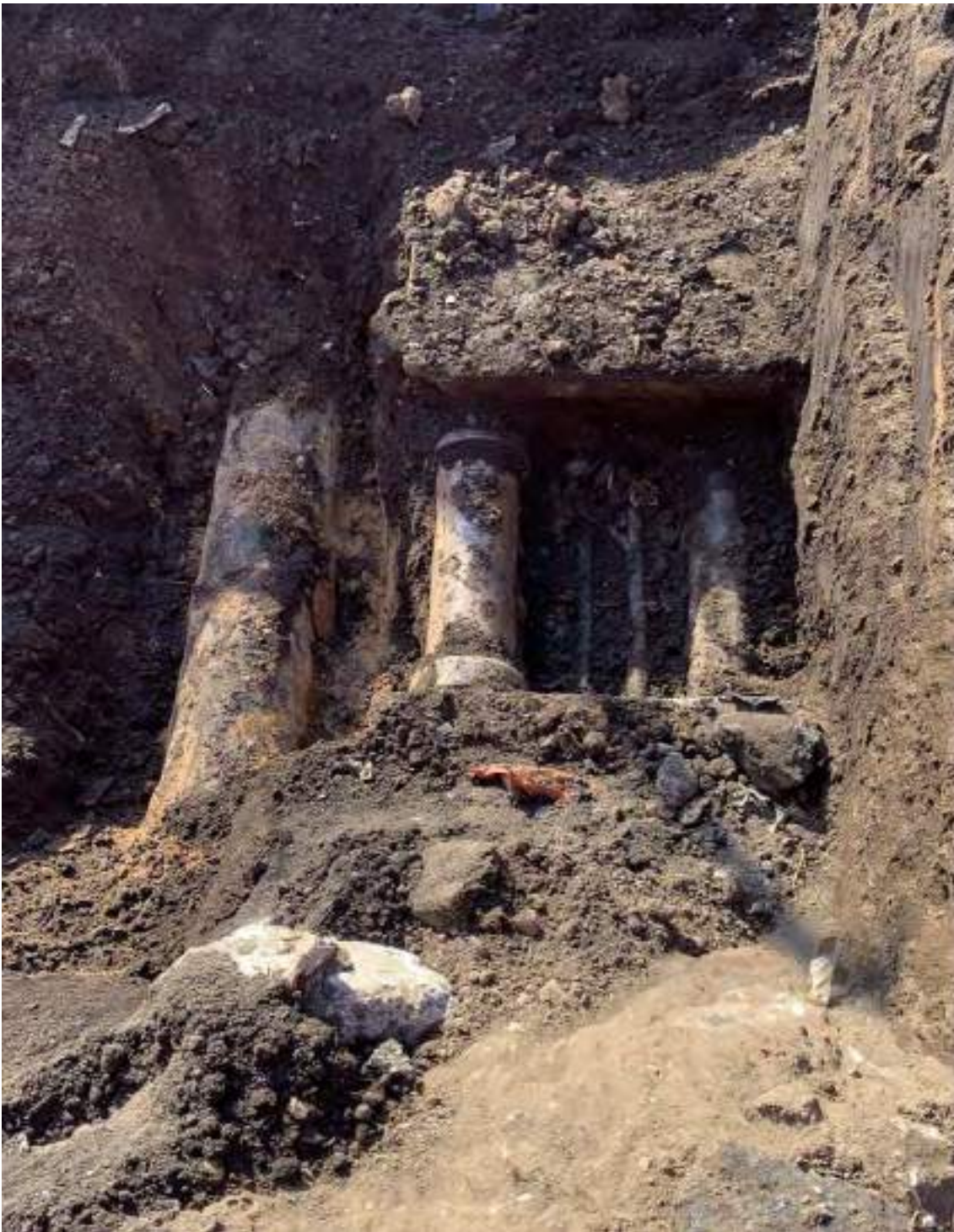
Figure 42 : Typical hand-dug excavation to locate and identify existing services on the site
