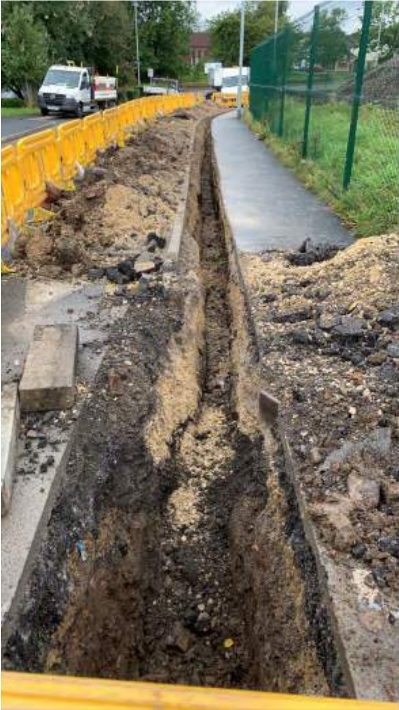
Figure 44 : Excavated trench ready for diversion of water pipe along Shellard Road on southern boundary of the site
