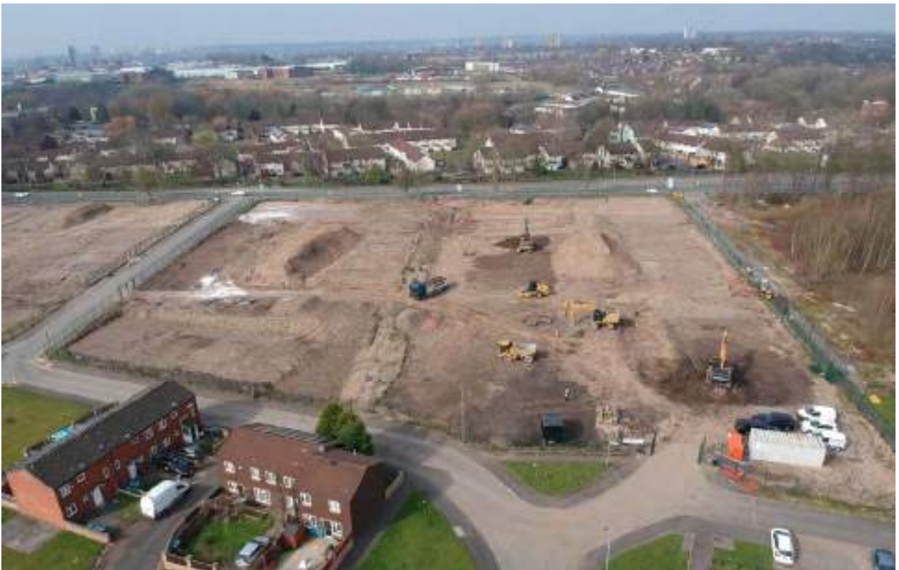
Figure 61 : Pile mat construction and export of surplus soils in northern part of site (backloading to reduce traffic movements)
