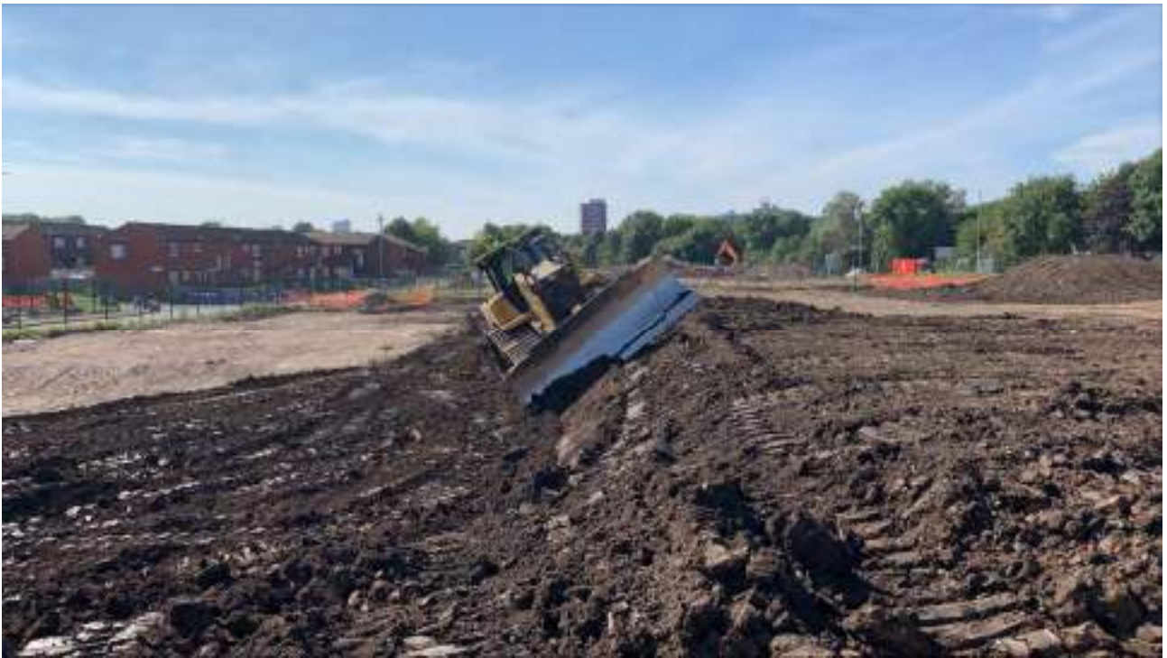
Figure 33 : Dozer being used to cut steep batters to profile
