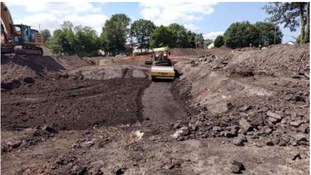
Figure 36 : Compaction of suitable fill material in accordance with the specification
