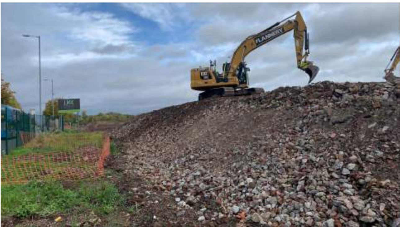
Figure 24 : Excavator maintaining the stockpile of site-produced crushed brick and concrete
