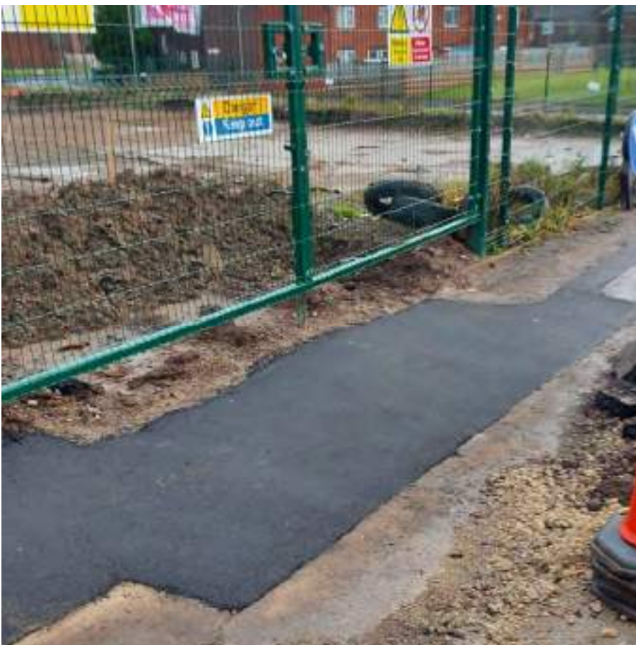
Figure 47 : Reinstatement of diversion trench to north footway of Paget Street
