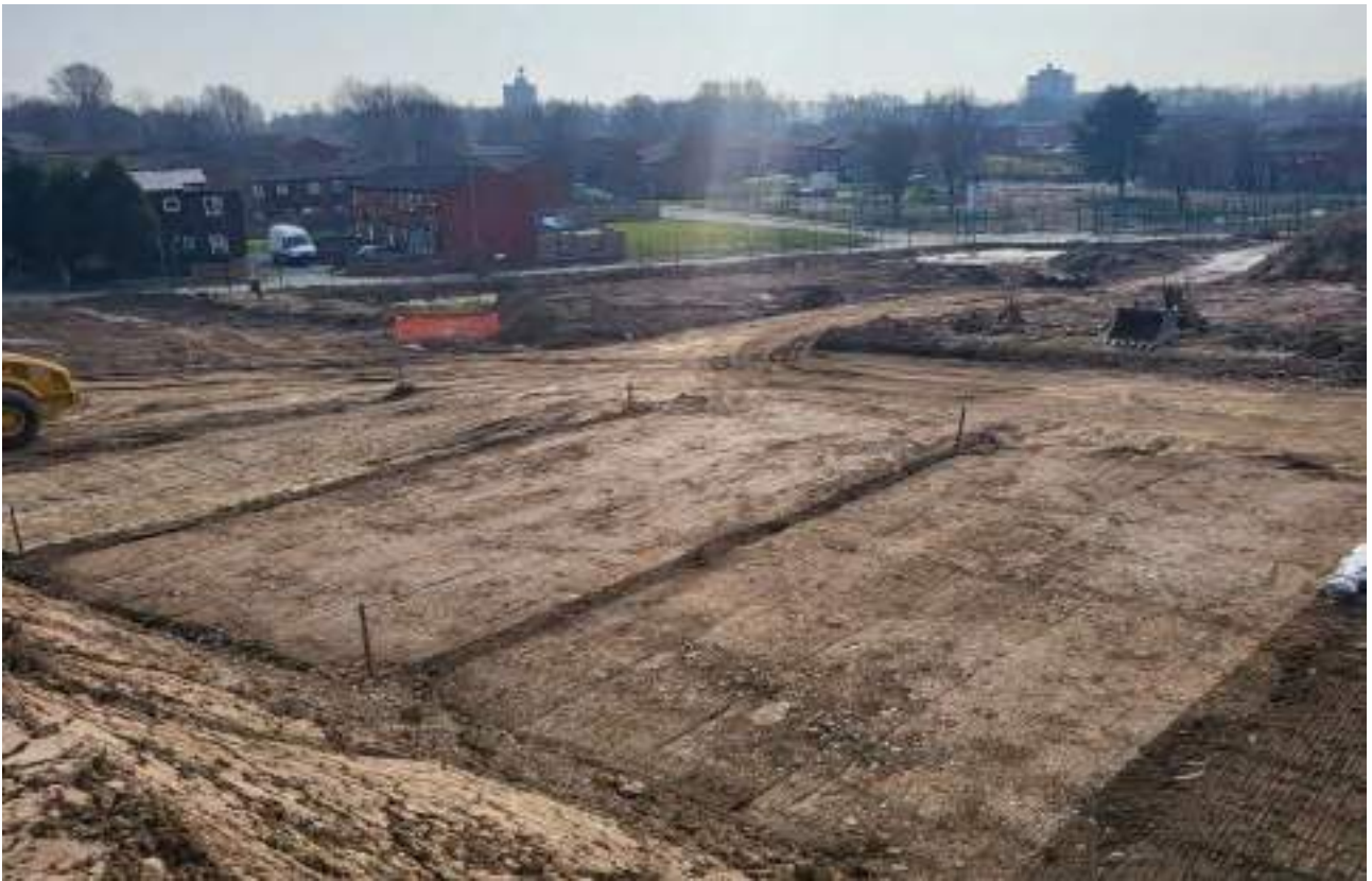
Figure 66 : Completed pile mats in north of site adjacent to Needwood Close access
