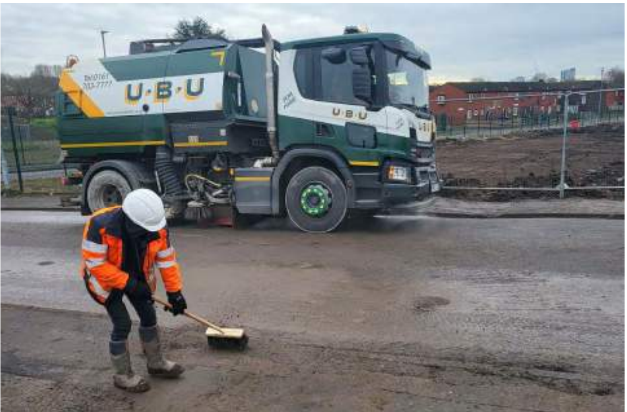
Figure 30 : Mechanical and manual maintenance of road pavement and footways during export operations
