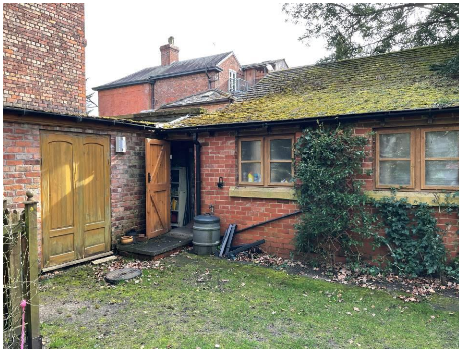
View at rear towards garage
