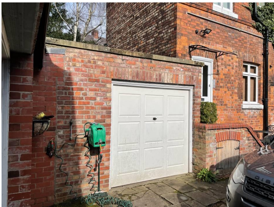
View from drive of outbuilding store to be demolished
