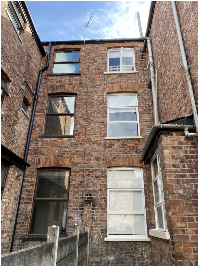
Photo 2 – Rear elevation of existing property
