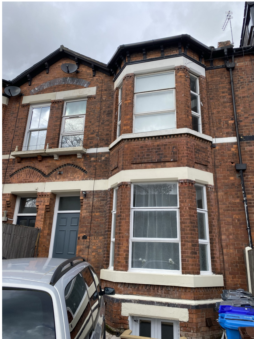
Photo 1 – Front elevation of existing property
